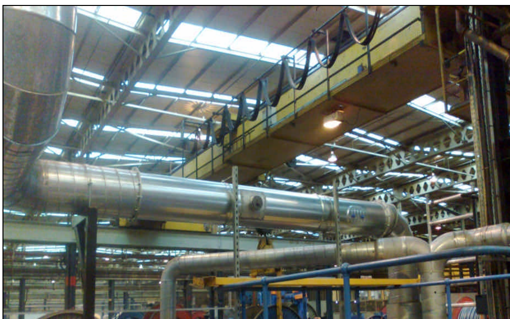
Picture of new pipework in position
