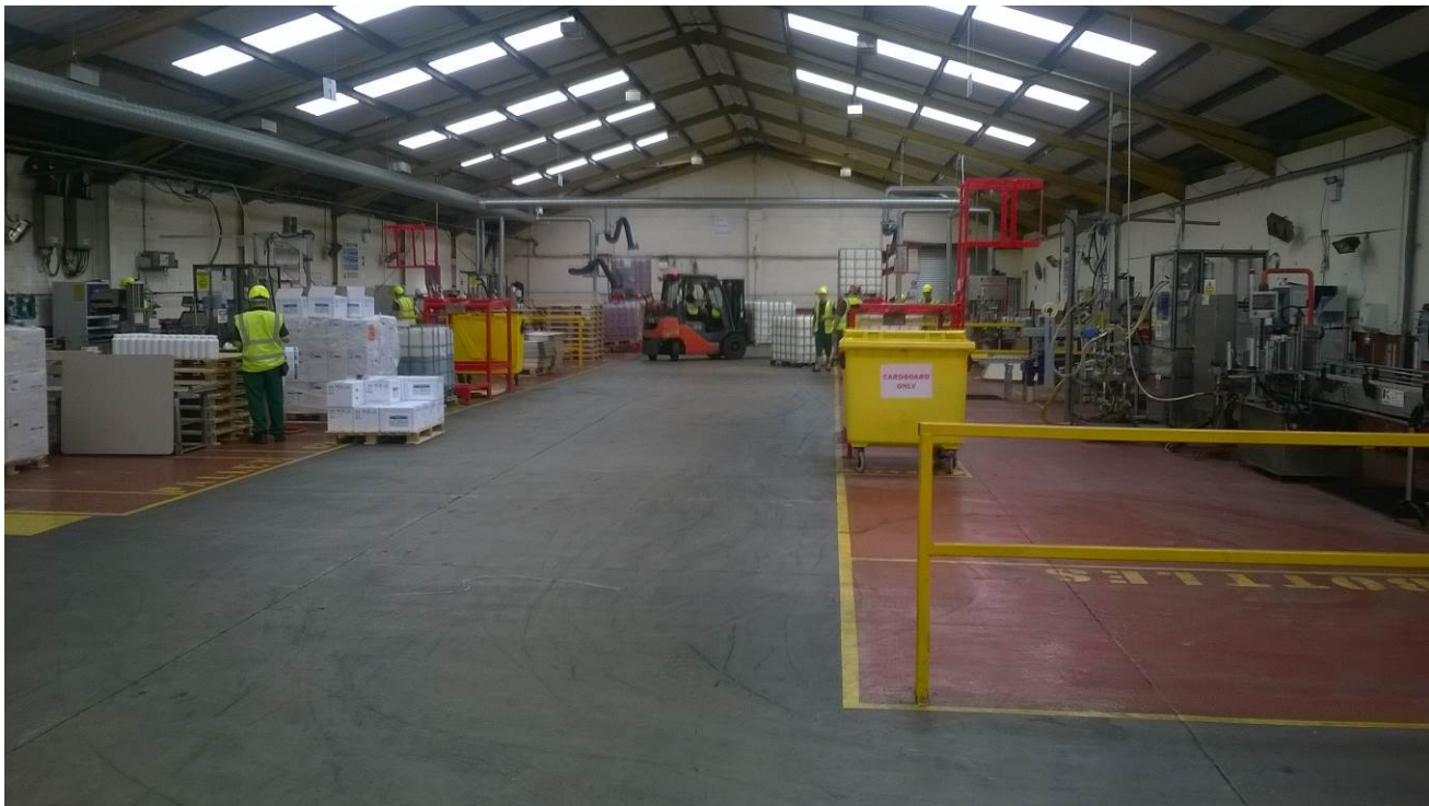
Micro-nutrient Bottle Filling Facility – note condition of ground slab and good level of house keeping
