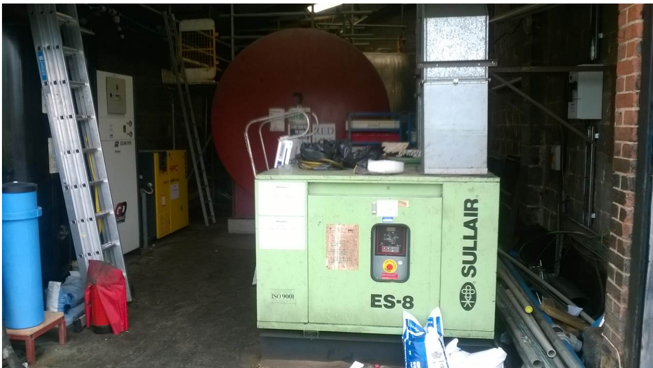
Former Herbicide Storage Area
