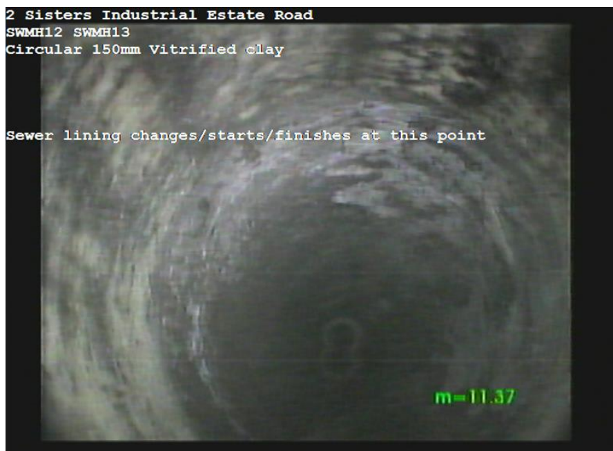
SWMH12X_075f19c8-260a-4442-bee9-583696bc34d0_20170623_160120_183.jpg, 00:00:44, 11.37m Sewer lining changes/starts/finishes at this point
