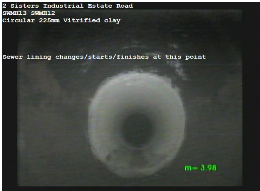
SWMH13X_8cb6fbfa-99dc-4d21-a428-313d3db1b8f1_20170623_154227_380.jpg, 00:06:32, 3.98m Sewer lining changes/starts/finishes at this point
