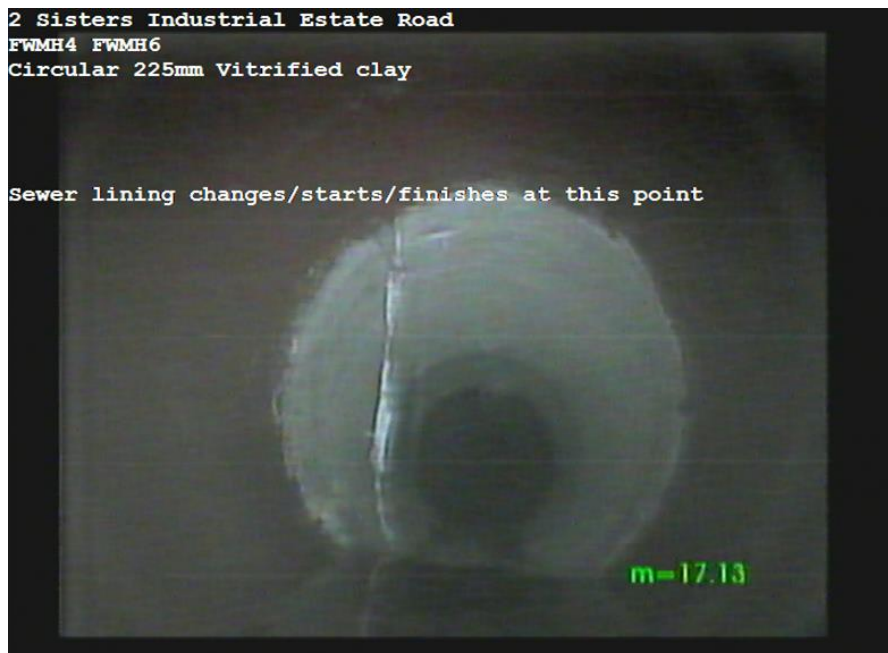
FWMH4X_c92f4f40-966b-4dac-bea2-30dd2616dc94_20170622_124837_089.jpg, 00:05:10, 17.13m Sewer lining changes/starts/finishes at this point
