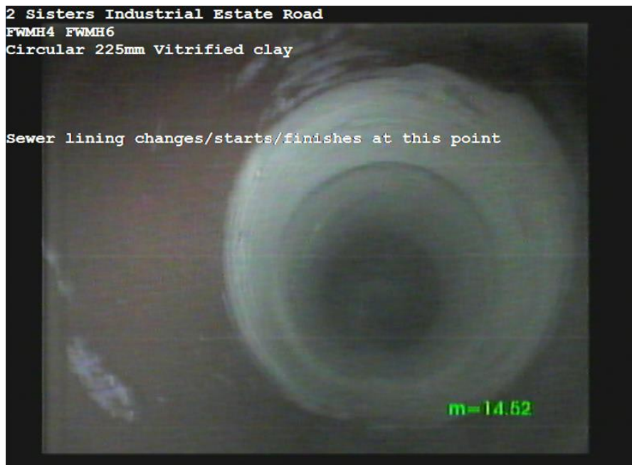
FWMH4X_88a9eda9-8477-4c78-97fb-2801c5b99fe4_20170622_124623_852.jpg, 00:03:43, 14.52m Sewer lining changes/starts/finishes at this point
