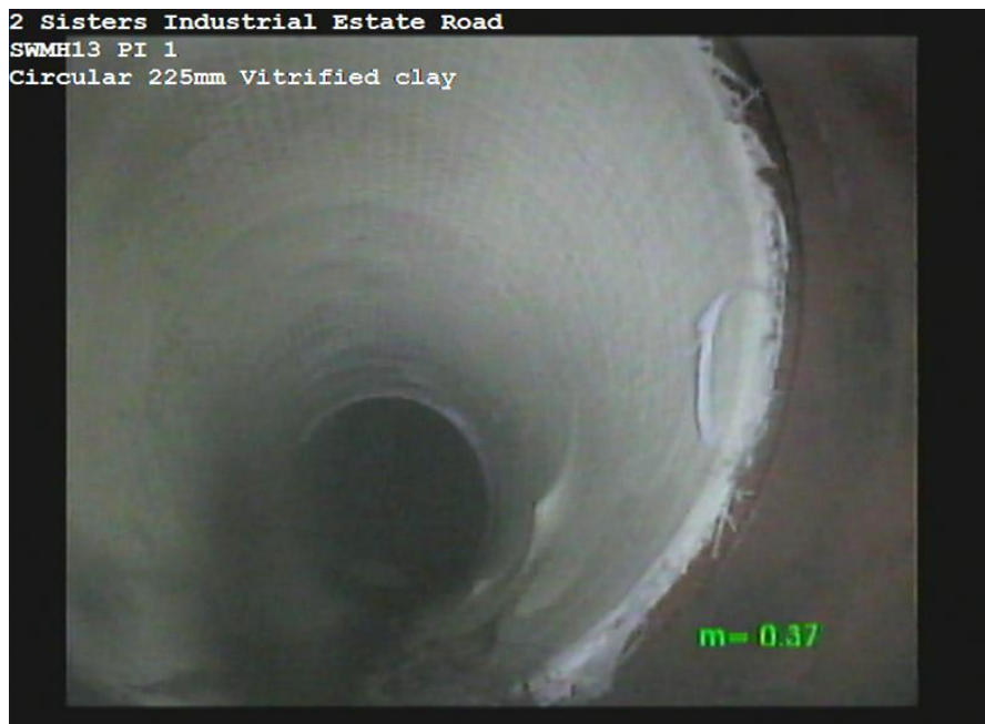
SWMH13X_e7789cd4-cdb6-4824-87b5-772fc65de6b3_20170620_152211_616.jpg, 00:00:00, 0.37m Sewer lining changes/starts/finishes at this point
