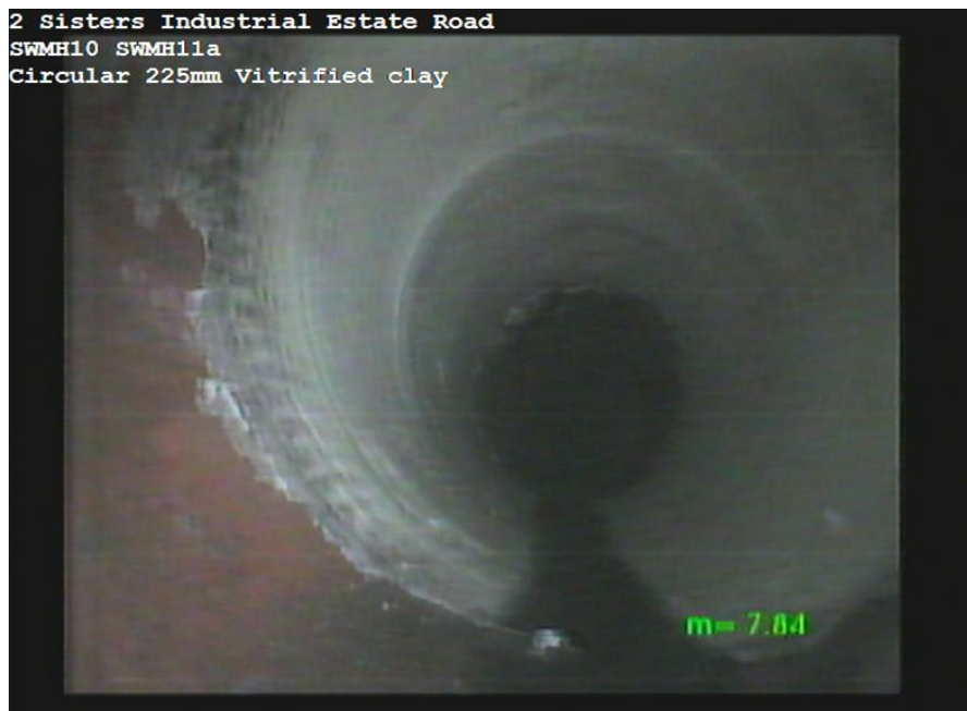
SWMH10X_9aac5131-bd9b-41d0-89fb-81cbdd461637_20170622_065351_994.jpg, 00:00:24, 7.87m Sewer lining changes/starts/finishes at this point
