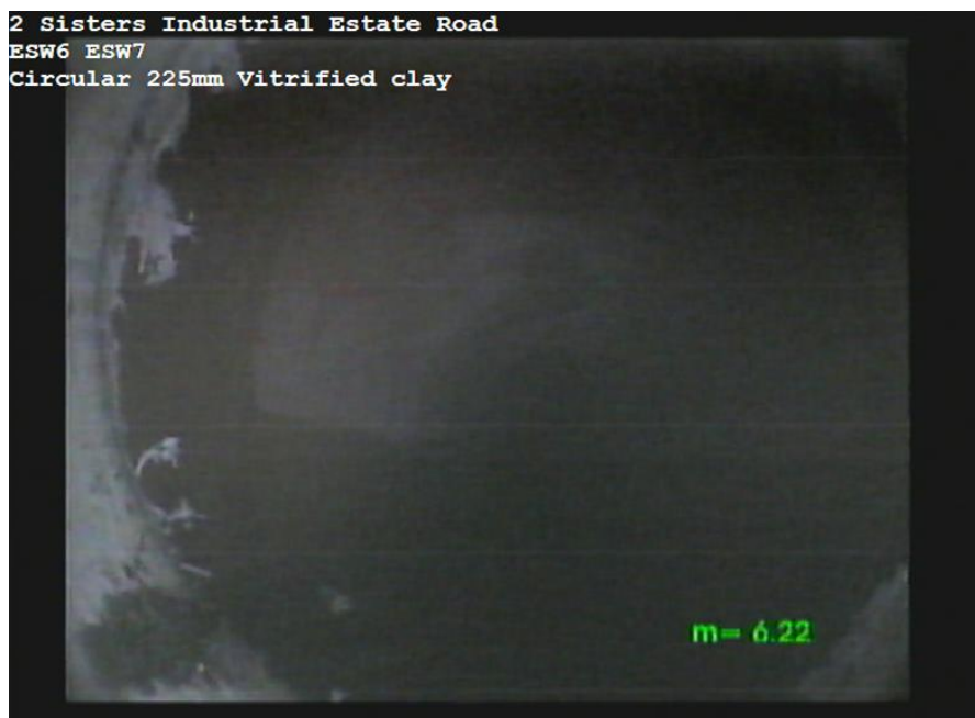
ESW6X_48006c78-d775-4be3-81e2-b1af41b6605d_20170623_152353_093.jpg, 00:00:47, 6.22m Sewer lining changes/starts/finishes at this point
