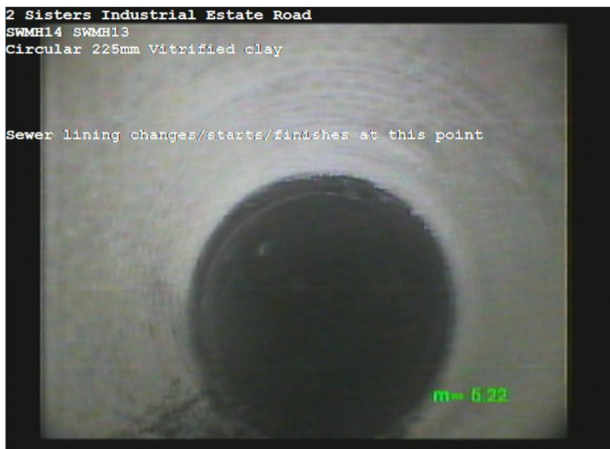
SWMH14X_3cf4f22c-c7c9-4d10-aa1f-c9d3c18e2699_20170623_153243_031.jpg, 00:01:51, 5.22m Sewer lining changes/starts/finishes at this point
