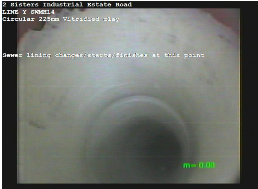
LINE YX_021c3de1-5d3d-41df-b5ab-a3a3a360c7d1_20170623_133006_960.jpg, 00:00:02, 0.00m Sewer lining changes/starts/finishes at this point
