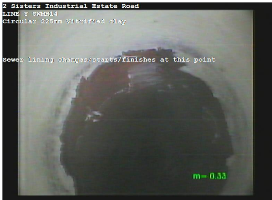
LINE YX_0e3e7a11-6a3b-4479-8b92-bf6e4fb0f9d8_20170623_133045_762.jpg, 00:00:24, 0.33m Sewer lining changes/starts/finishes at this point
