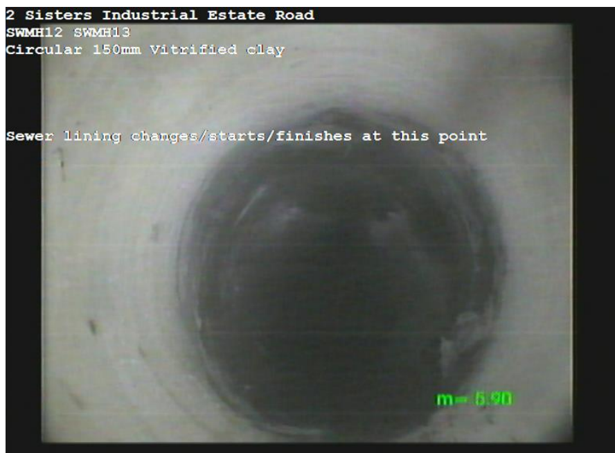
SWMH12X_81ab399a-8ae1-4155-81d9-0ddff52074c4_20170623_155928_081.jpg, 00:00:00, 5.90m Sewer lining changes/starts/finishes at this point
