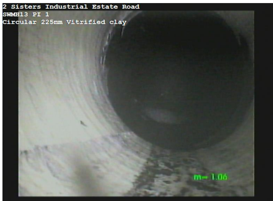
SWMH13X_dd588aea-59b7-4d0f-a5c0-c70071613441_20170620_152341_569.jpg, 00:01:03, 1.06m Sewer lining changes/starts/finishes at this point
