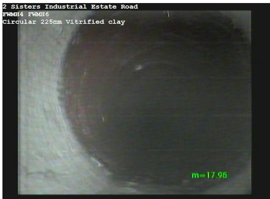
FWMH4X_ed670d45-7678-48c9-b225-86665e92ac73_20170622_125005_943.jpg, 00:05:32, 17.95m Sewer lining changes/starts/finishes at this point
