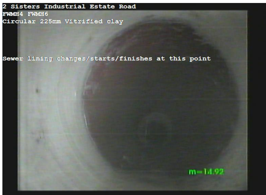
FWMH4X_5235b1f3-41d3-47b2-aef3-8563609d1de4_20170622_124708_162.jpg, 00:03:58, 14.92m Sewer lining changes/starts/finishes at this point
