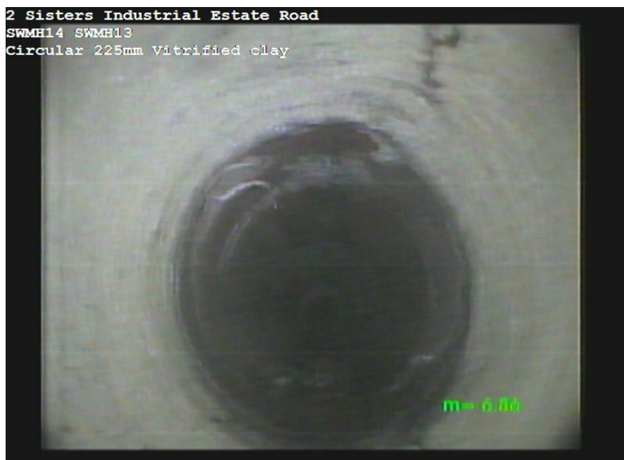
SWMH14X_bc4eaccb-041a-4fe0-ace0-eca2422328ec_20170623_153408_637.jpg, 00:02:38, 6.87m Sewer lining changes/starts/finishes at this point
