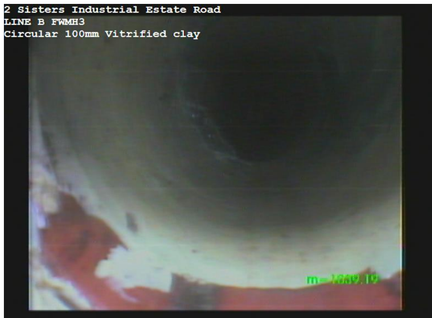
LINE BX_98fe3b8d-390e-491a-974a-eccb7cfcdb41_20170623_134034_080.jpg, 00:00:00, 0.01m Sewer lining changes/starts/finishes at this point
