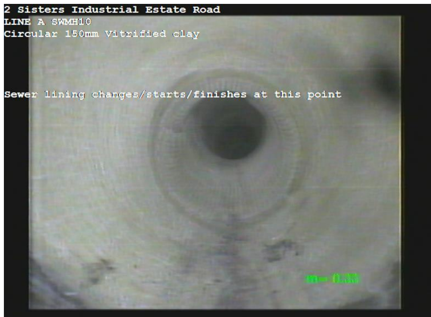
LINE AX_1fbc1e05-b299-436a-9252-769fd5c77bff_20170620_114150_457.jpg, 00:00:13, 0.33m Sewer lining changes/starts/finishes at this point
