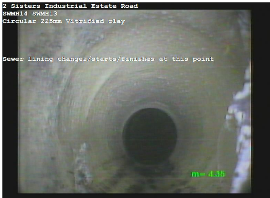
SWMH14X_5ee8f9ab-a427-48ce-83c6-79fee2651629_20170623_153055_237.jpg, 00:00:33, 4.35m Sewer lining changes/starts/finishes at this point
