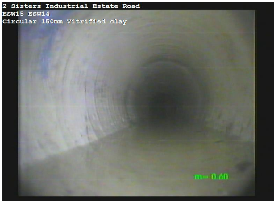
ESW15X_3ec77f19-61bf-4152-aa76-f4e0fd1c5cb7_20170623_055005_159.jpg, 00:00:00, 0.60m Sewer lining changes/starts/finishes at this point
