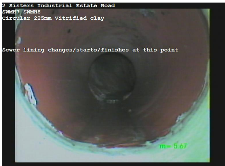
SWMH7X_051899fe-31e4-47c8-bb6f-31994bfe1854_20170622_174924_754.jpg, 00:01:04, 5.67m Sewer lining changes/starts/finishes at this point
