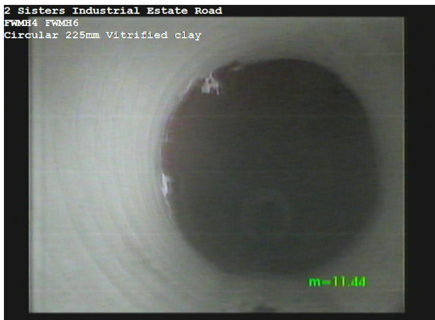
FWMH4X_cf664817-d747-42e8-b4b5-289354077130_20170622_124352_568.jpg, 00:02:01, 11.44m Sewer lining changes/starts/finishes at this point
