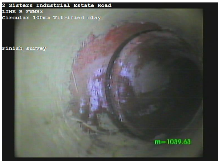
LINE BX_f2997f23-f1f9-4459-bfec-56504196a0b0_20170623_134129_319.jpg, 00:00:44, 0.35m Sewer lining changes/starts/finishes at this point
