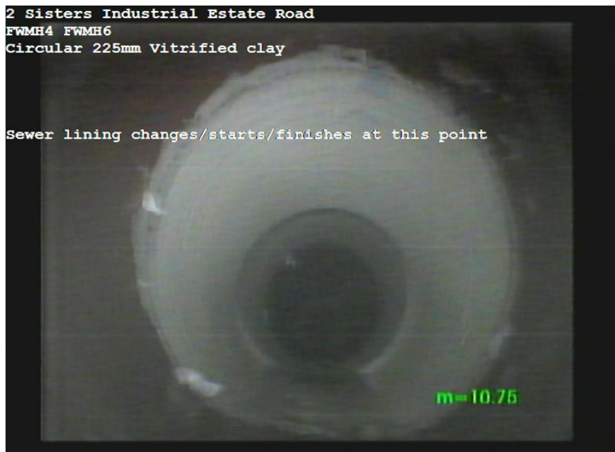
FWMH4X_be5f6ca3-4b84-40f6-a85a-a5fcacce18b9_20170622_124309_459.jpg, 00:01:39, 10.75m Sewer lining changes/starts/finishes at this point
