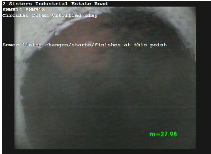
SWMH14X_58a39c6a-91ba-4d30-a303-18e4979c10cb_20170623_153836_690.jpg, 00:05:21, 27.98m Sewer lining changes/starts/finishes at this point
