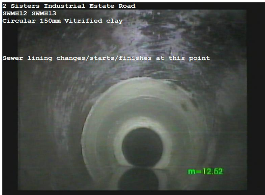
SWMH12X_d05aedic9-15cb-41da-85b7-c522af7caab4_20170623_160227_720.jpg, 00:01:30, 12.52m Sewer lining changes/starts/finishes at this point
