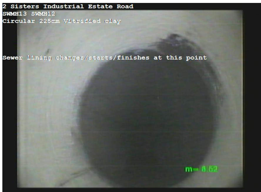
SWMH13X_4f7a62b8-330c-4daf-a230-443930e307f4_20170623_154503_096.jpg, 00:01:02, 8.53m Sewer lining changes/starts/finishes at this point
