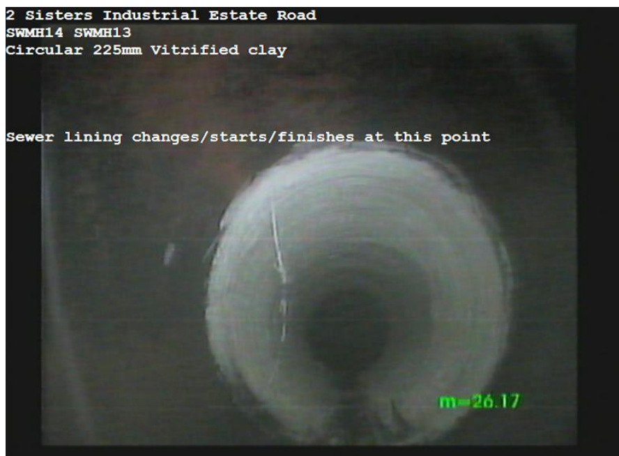
SWMH14X_491e6763-f1d0-4a81-825a-773ee96bd826_20170623_153750_342.jpg, 00:04:59, 26.17m Sewer lining changes/starts/finishes at this point
