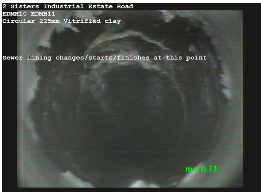
EDMH10X_184e0cd9-7154-424c-9ab7-e700b0c67050_20170623_122308_167.jpg, 00:00:25, 0.73m Sewer lining changes/starts/finishes at this point
