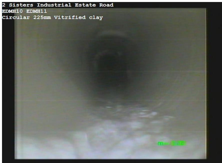
EDMH10X_b9de2752-edb1-4100-80fb-94f571934139_20170623_122606_461.jpg, 00:00:04, 0.00m Sewer lining changes/starts/finishes at this point
