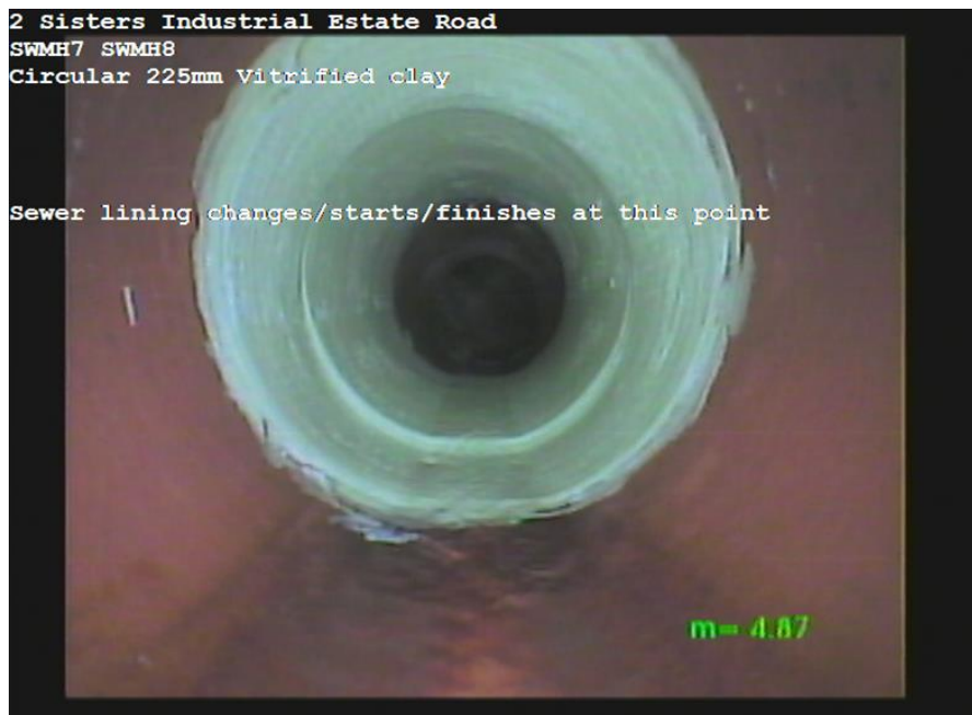
SWMH7X_403ed8c3-5bb3-4782-8120-80dc687a1669_20170622_174835_108.jpg, 00:00:38, 4.87m Sewer lining changes/starts/finishes at this point
