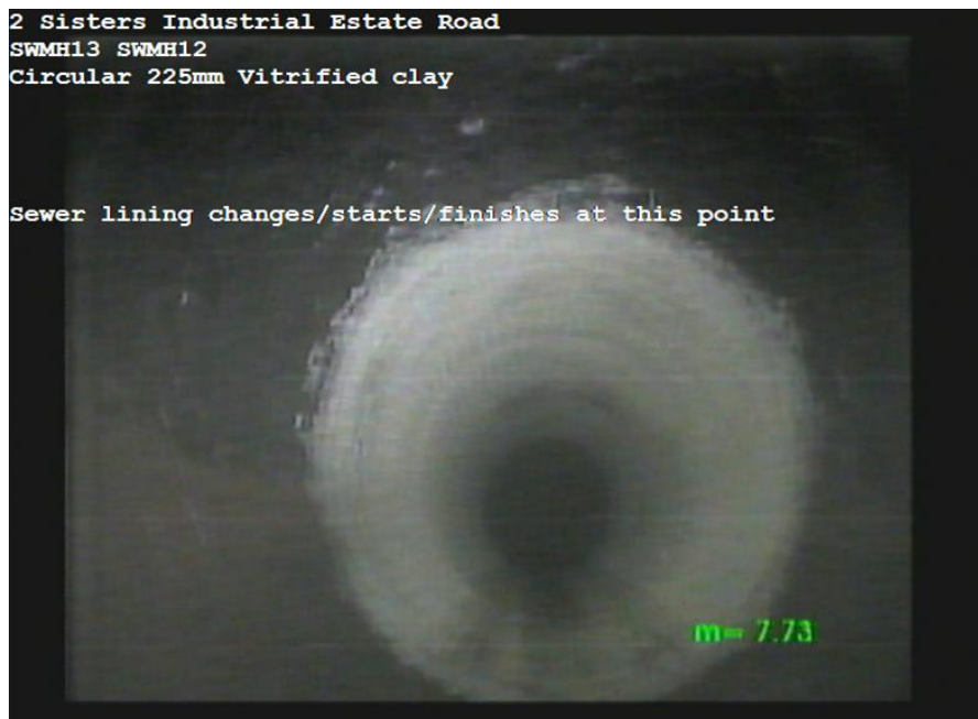
SWMH13X_bd16db54-2aa8-43dd-975d-c54e5d65a4a8_20170623_154422_191.jpg, 00:00:49, 7.73m Sewer lining changes/starts/finishes at this point
