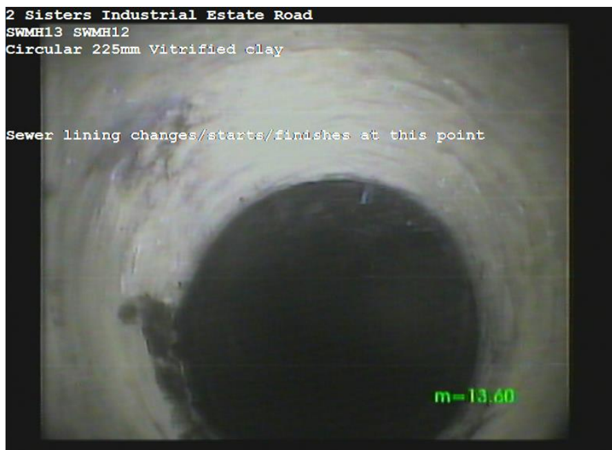
SWMH13X_08acc3c8-6cf6-41b0-aeae-9900846d65c2_20170623_154717_579.jpg, 00:01:51, 13.60m Sewer lining changes/starts/finishes at this point
