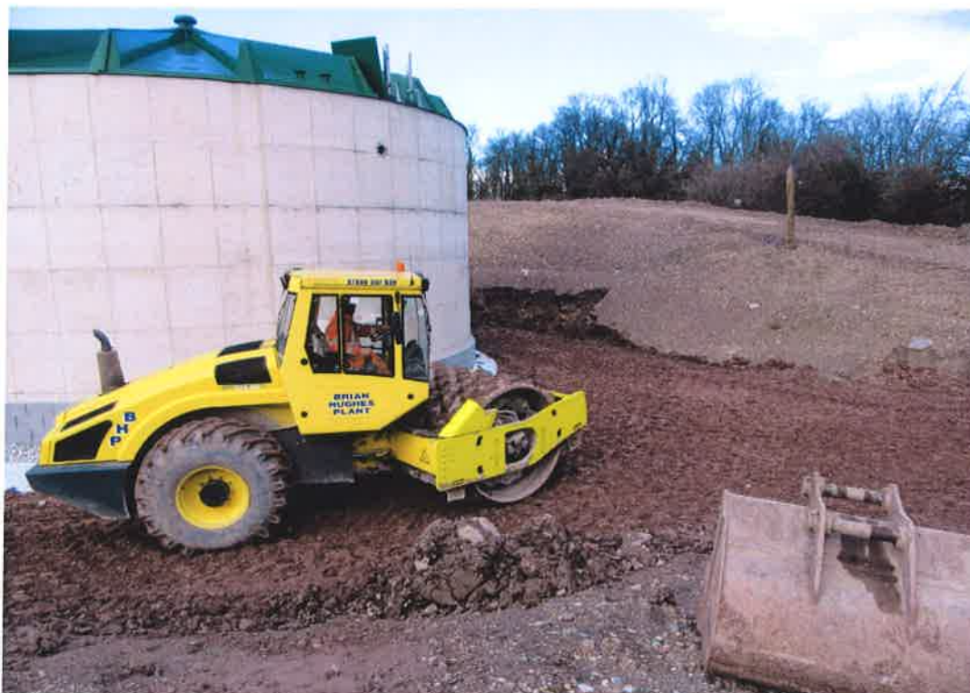
Compaction of engineering clay to apron around tank
