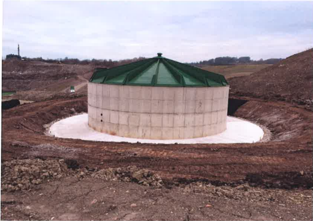
Clay containment bund and concrete apron completed
