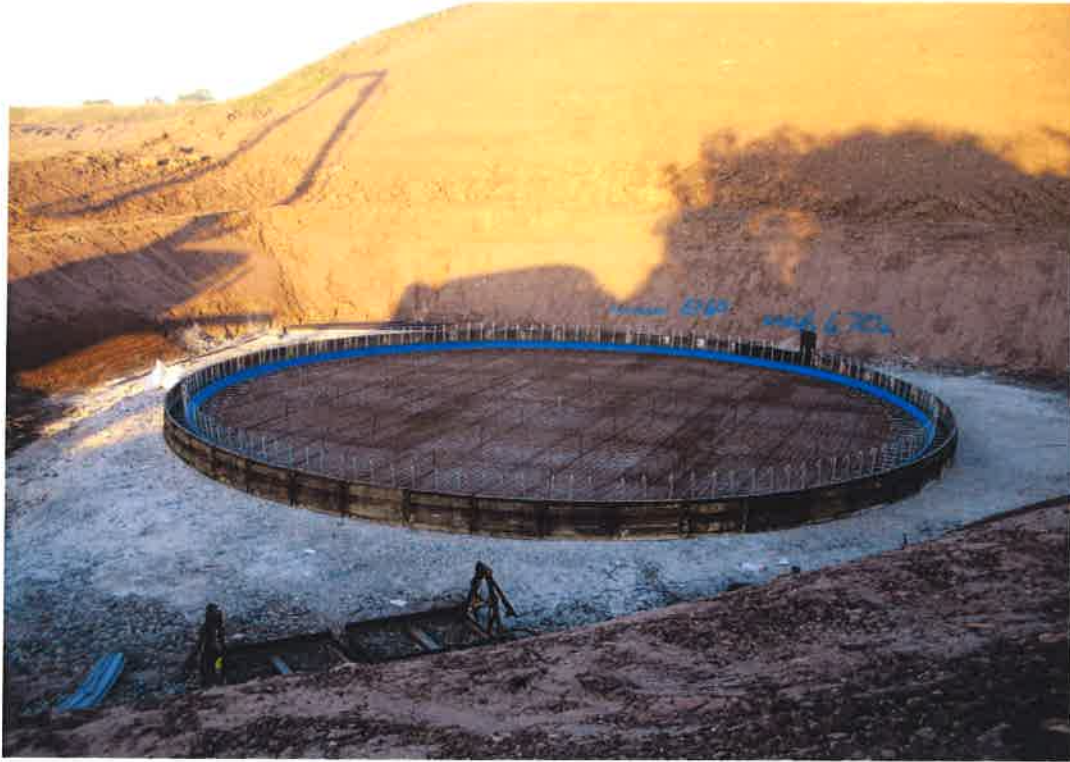
Basal formwork, waterstop and reinforcement prior to casting
