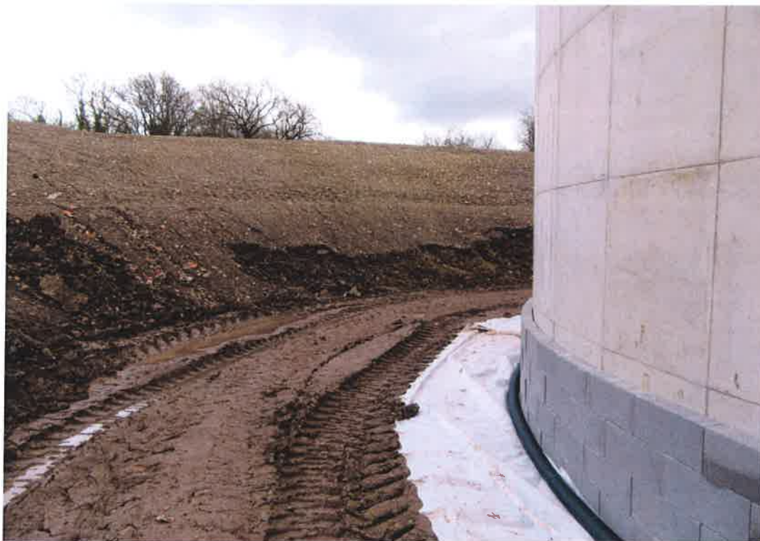
Installation of leak detection pipework to base of tank sidewall
