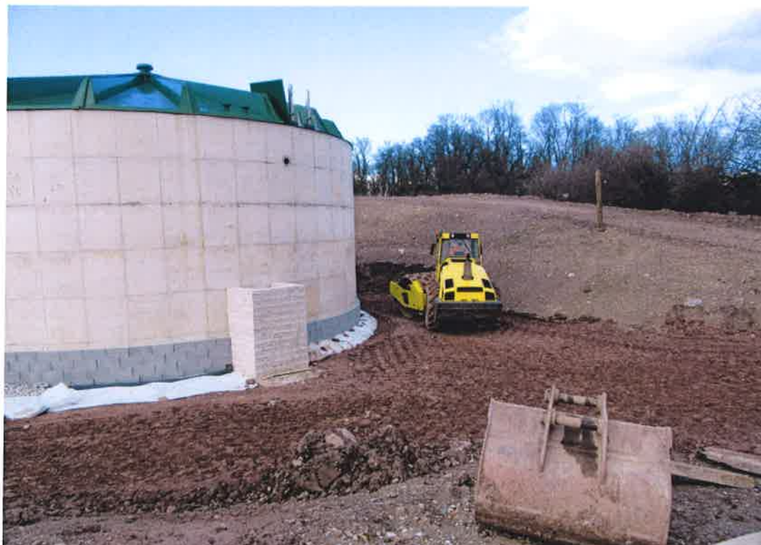
Leak detection chamber visible against tank sidewall
