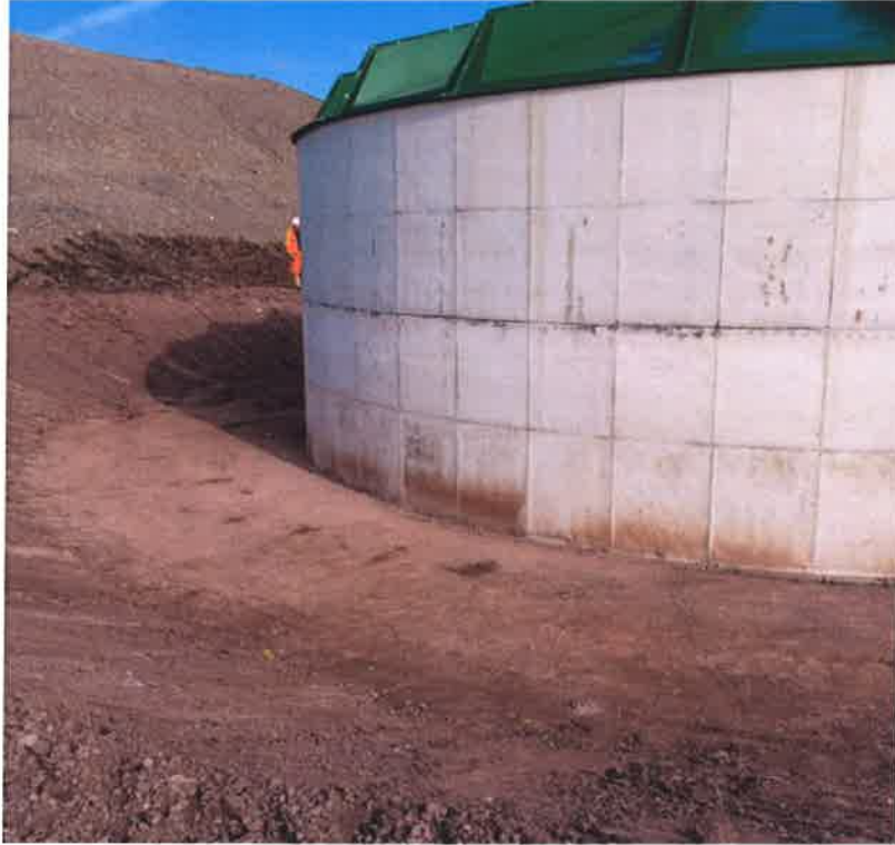
Clay placement and compaction completed, prior to concrete apron casting
