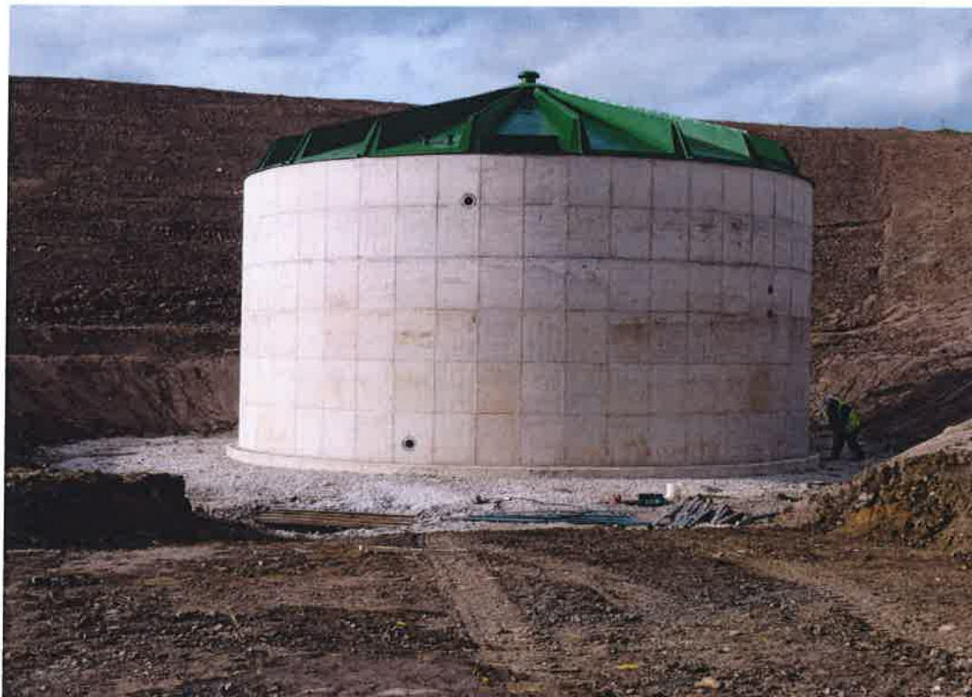
Completed tank construction; clay containment incomplete
