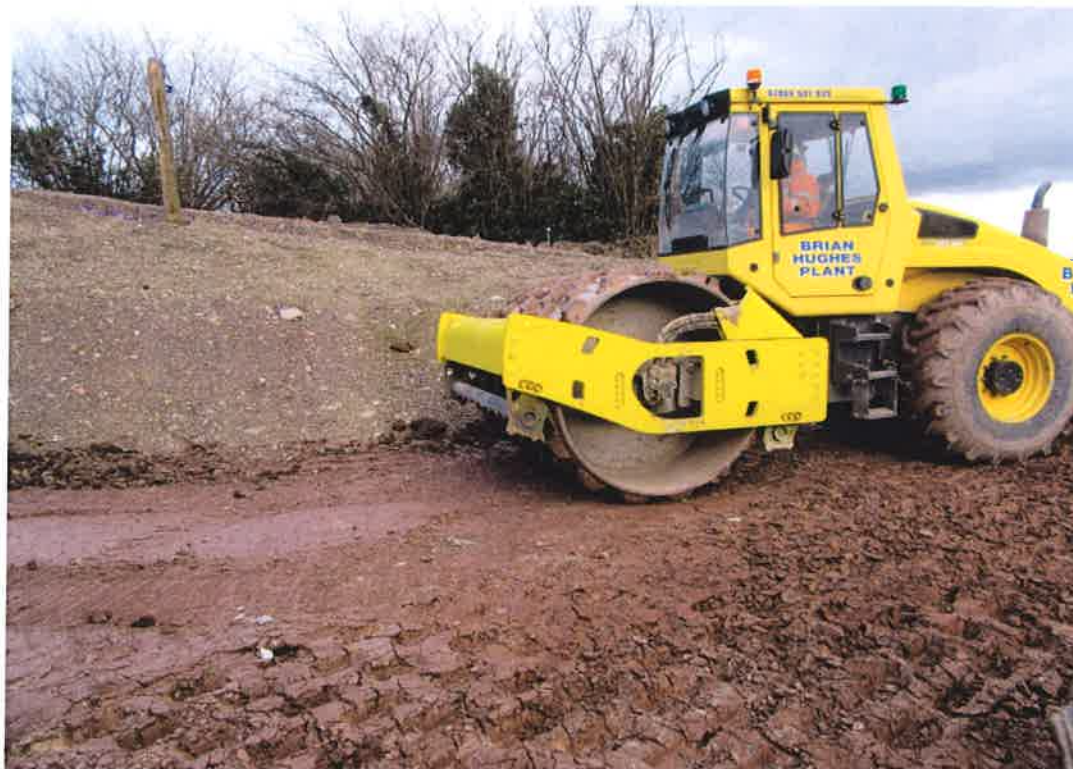
Padfoot roller utilised for construction of tank containment (Bomag BW213 DH)
