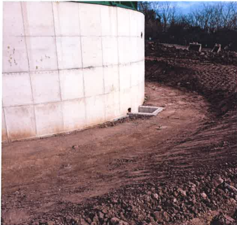
Leak detection chamber now flush with top of containment clay, prior to casting of apron
