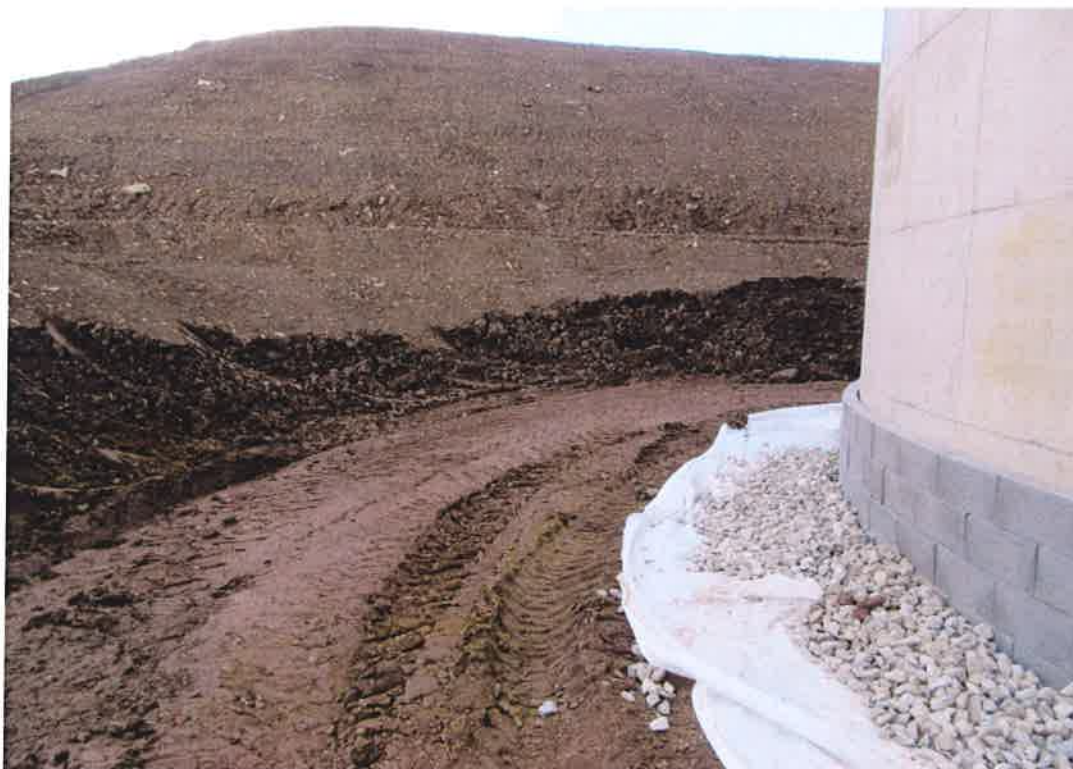
Gravel surround and separation geotextile to leak detection drain
