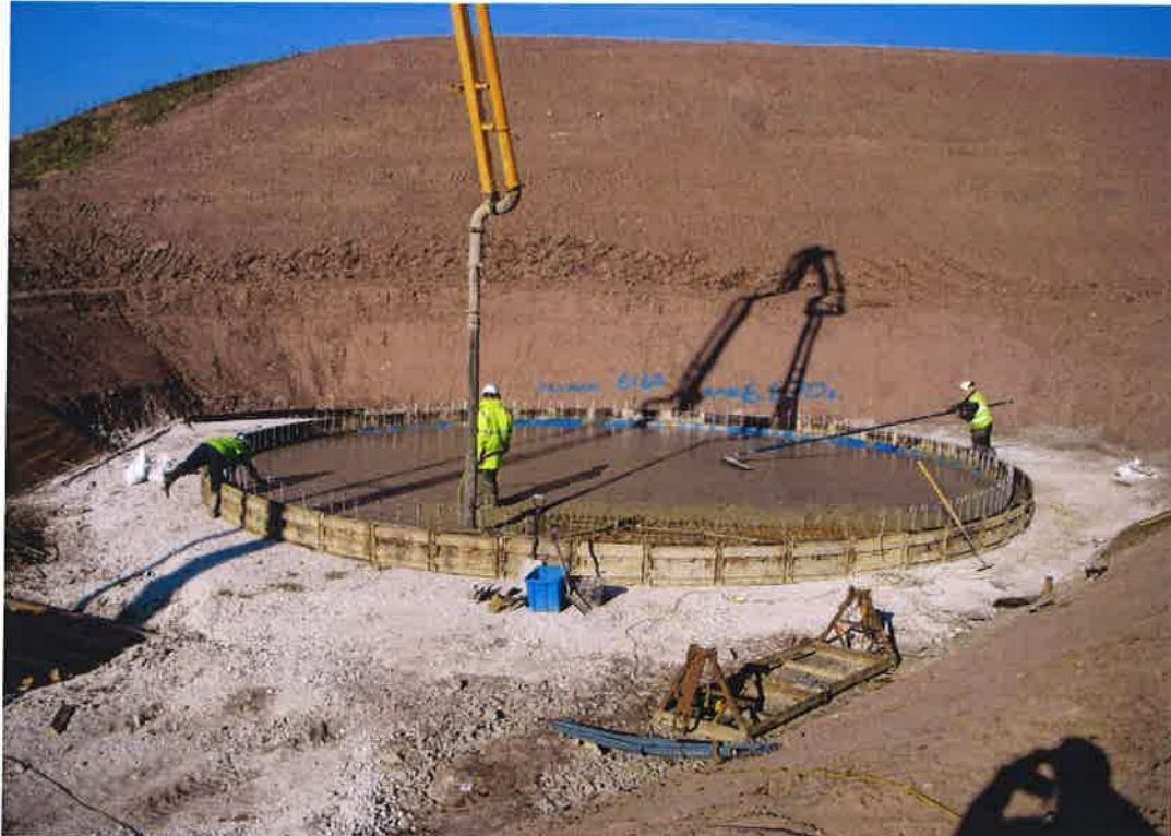
Basal slab being cast
