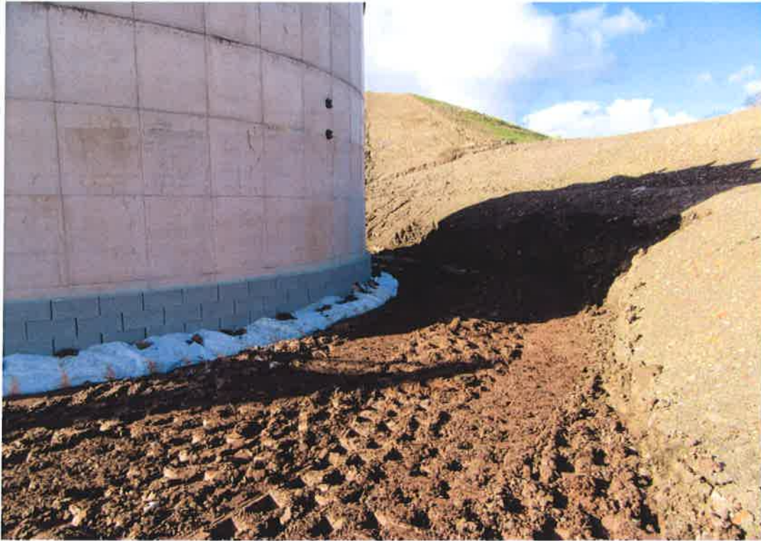
Leak detection drain installation completed; clay compaction under way
