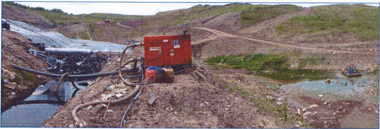
Photograph 1.5 showing (from left to right) the leachate sump, the containment bund and surface water sump. Methane rich gas bubbling in both the leachate sump and surface water sump.
