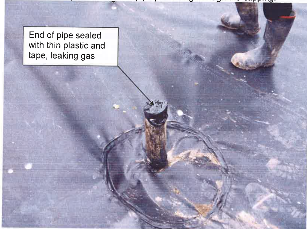
PHOTO 4 : Poorly sealed vertical pipe protruding through the capping.
