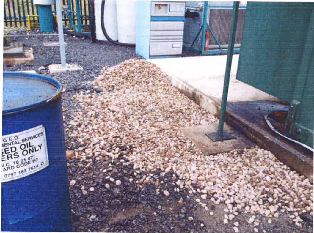
PHOTO 2- Oil Contaminated Ground Removed
