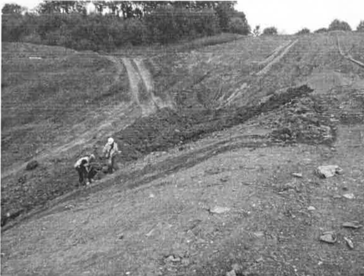
Photograph 1.1:- North Flank Cell 3, Eastern section. Showing area of flank in process of being regraded
