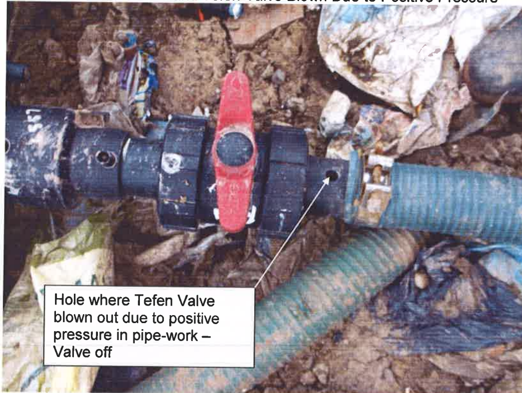
PHOTO 8: Valve Closed and Tefen Valve Blown Due to Positive Pressure
