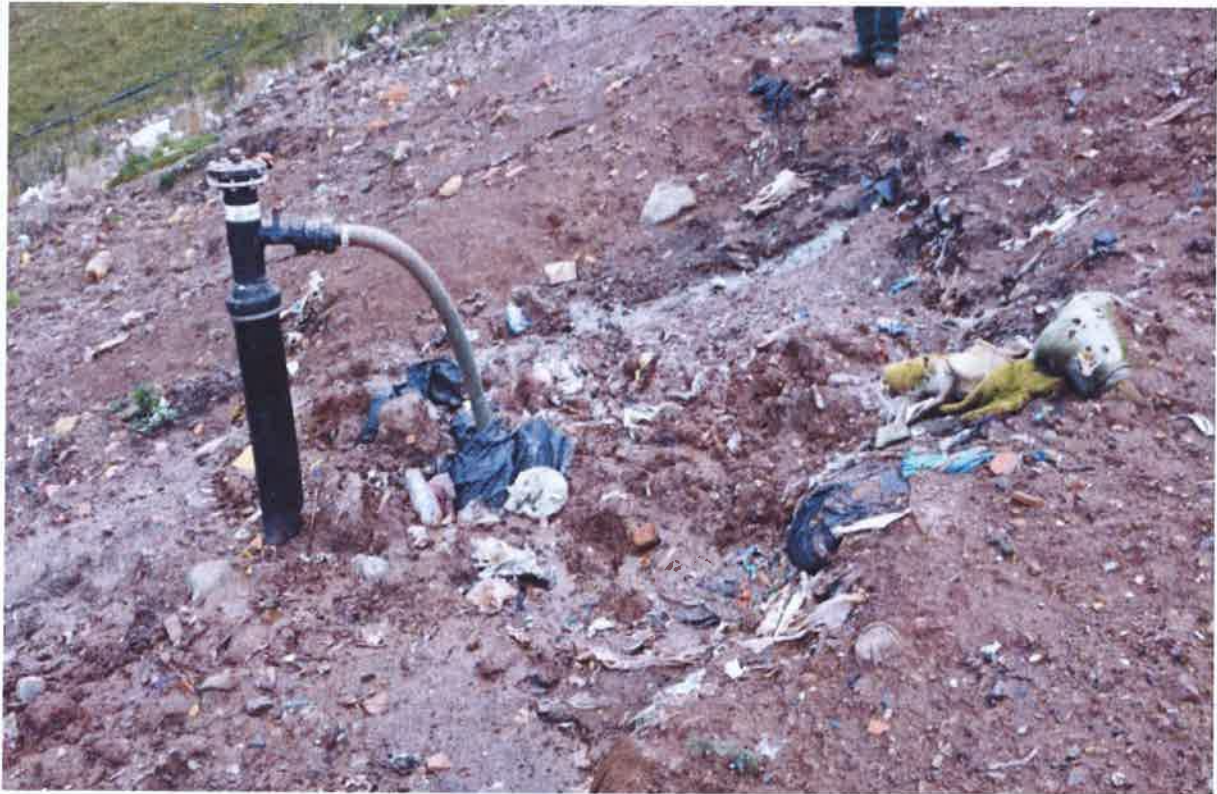
Fugitive Gas Emissions from gas well on flank, Point 13, Photo 06:
