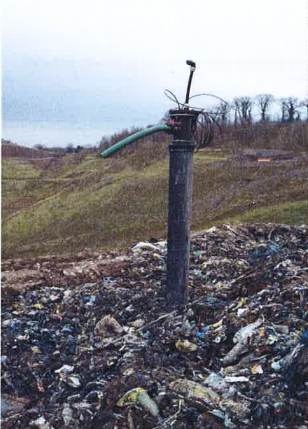
Unattached gas well, Point 9, Photo 04:
