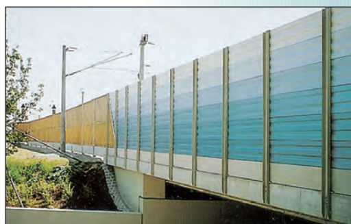
Lightweight aluminium panel system suitable for bridges and underpasses.
