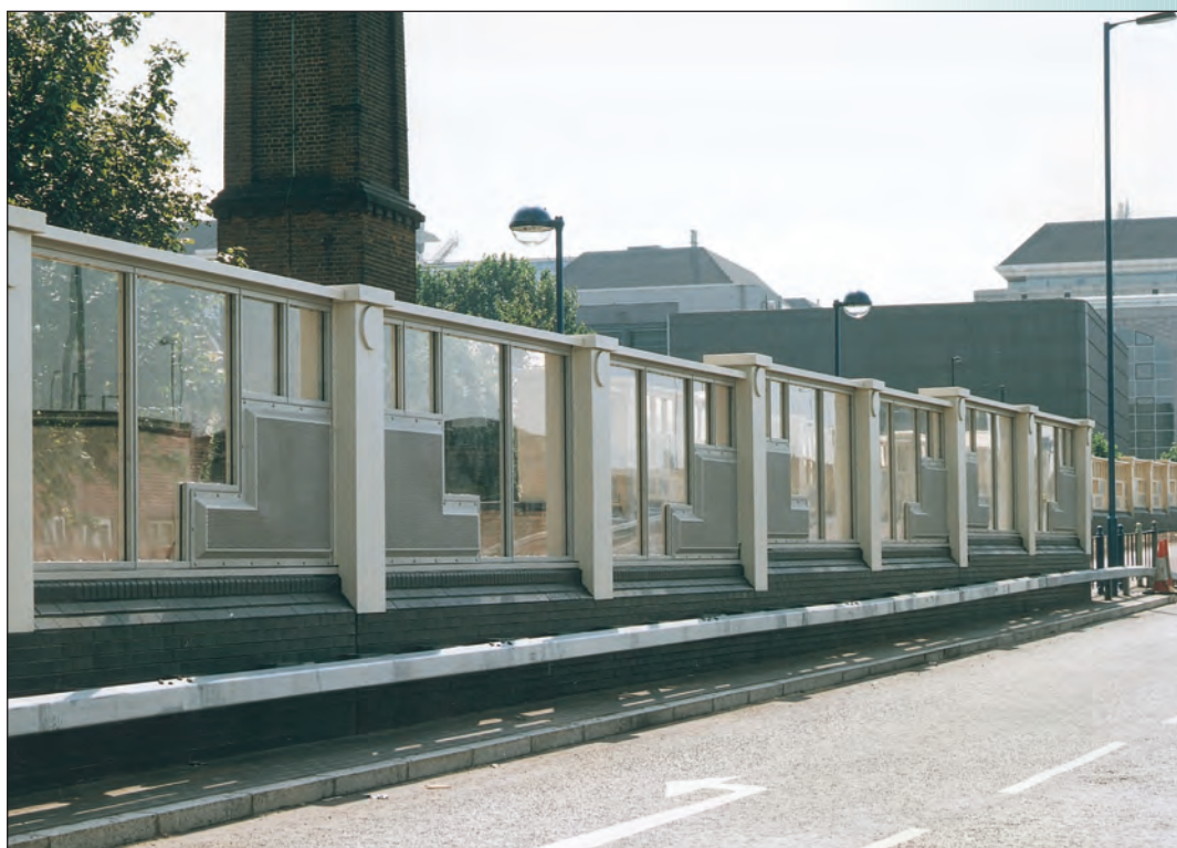
Combined aluminium absorptive and acrylic barrier system allowing bespoke architectural designs.
