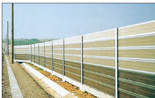
Aluminium modular system designed for easy installations on roads and railways.
