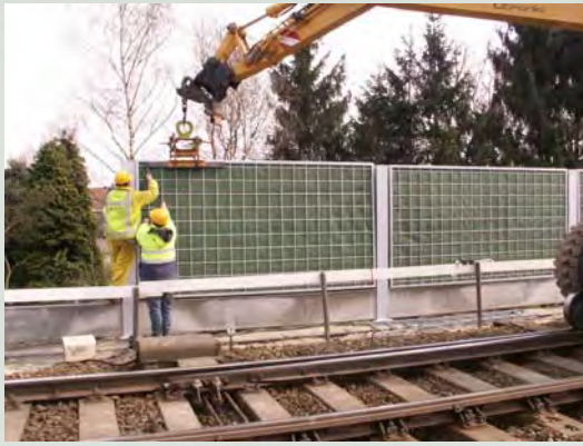
Installation of the pre assembled elements
