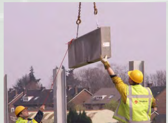
Installation of the concrete bottom part
