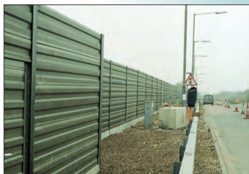
Steel galvanised and painted absorptive noise barriers designed for heavy traffic on main roads and motorways.
