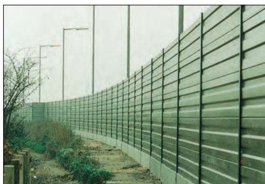
Steel galvanised and painted absorptive noise barriers designed for heavy traffic on main roads and motorways.
