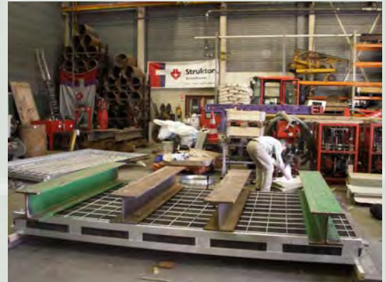
Windload test for NS-Railway
