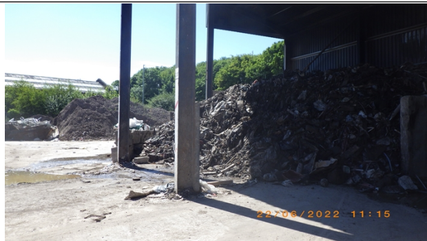
Fire damaged waste with runoff
