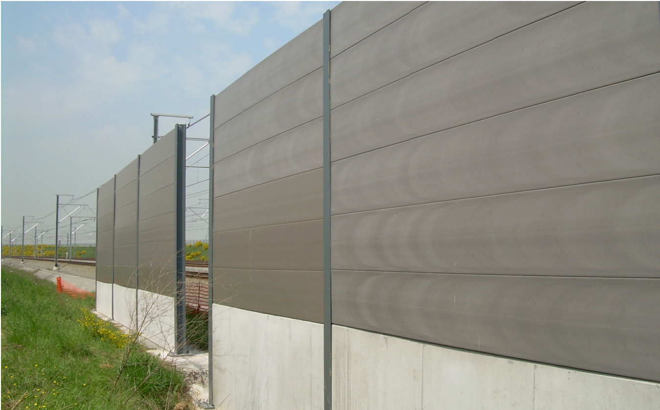
TYPICAL INSTALLATION ADJACENT RAILWAY
