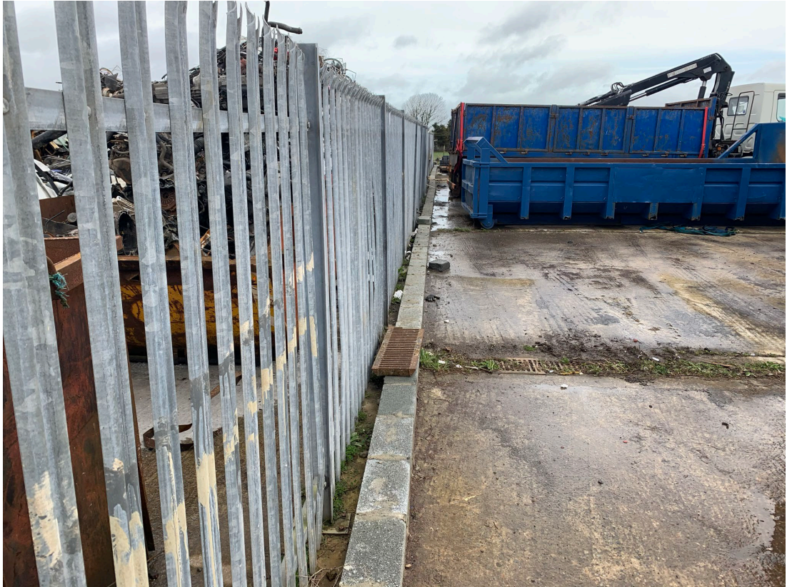
Plate 2-1 Site perimeter bunding
