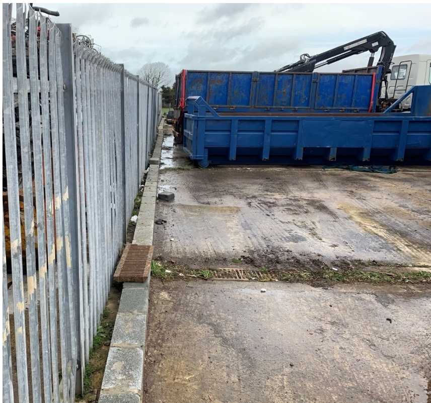
Plate 3-3 Concrete upstand around site perimeter
