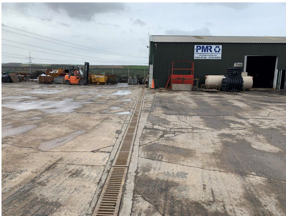
Plate 3-4 Part of the surface drainage network
