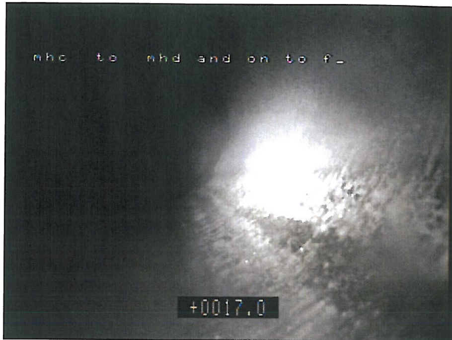
Photo: 38_6a, Tape No.: 01, 00:03:30 17m, General Observation, Remark: START OF MH D
