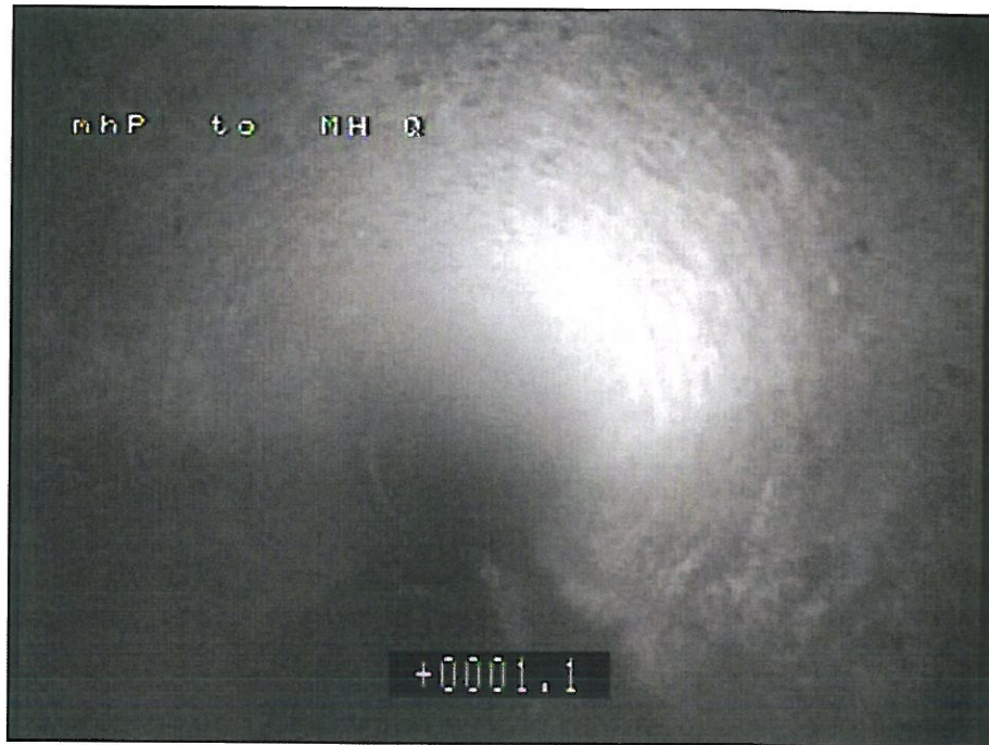
Photo: 104_3a, Tape No.: 01, 00:00:00 0m, Water level, 05 % height/diameter
