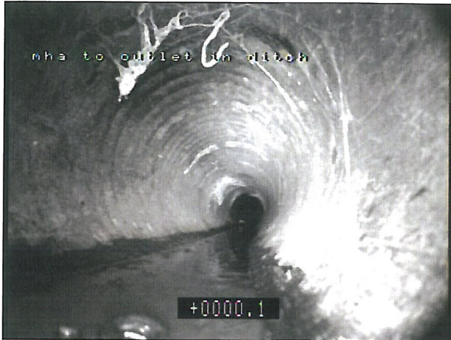
Photo: 2_2a, Tape No.: 01, 00:00:00 0m, Manhole Remark: MH A
