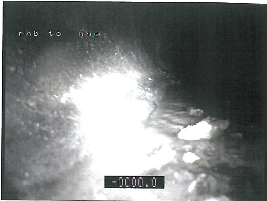
Photo: 15_2a, Tape No.: 01, 00:00:00 0m, Manhole Remark: MH B
