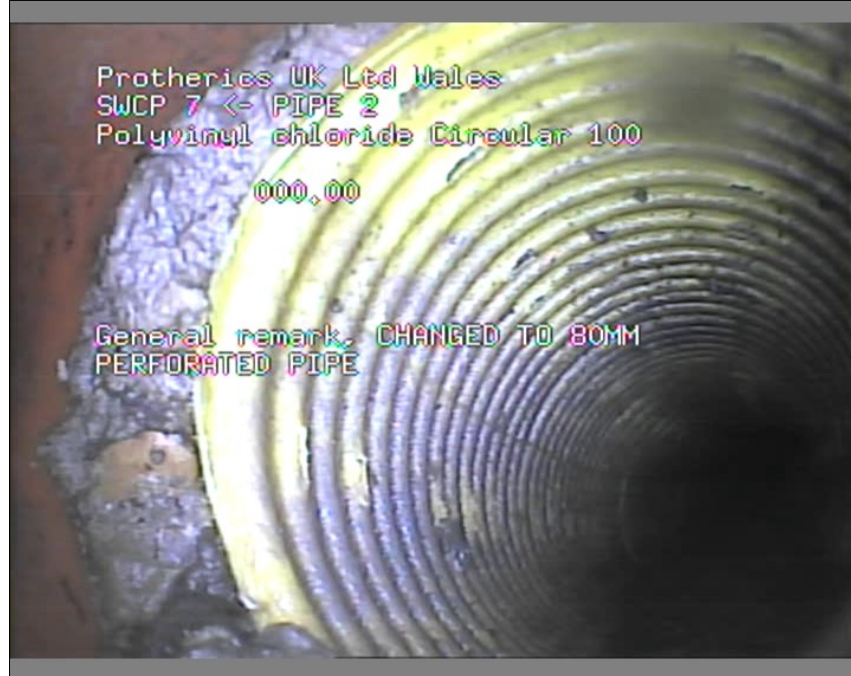
Photo: 44_44_269_A.JPG 0m, General remark
