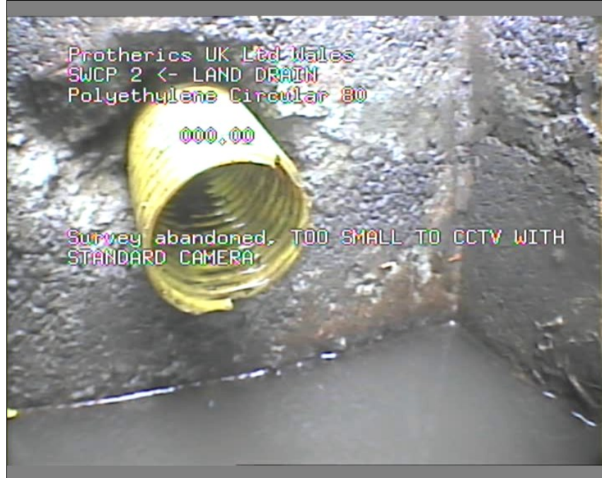
Photo: 25_25_143_A.JPG 0m, Survey abandoned
