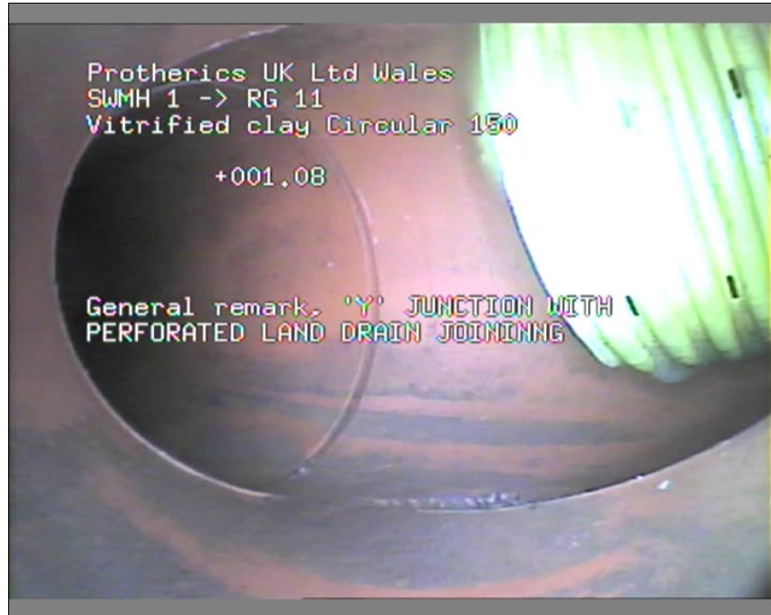
Photo: 22_22_129_A.JPG 1.08m, General remark
