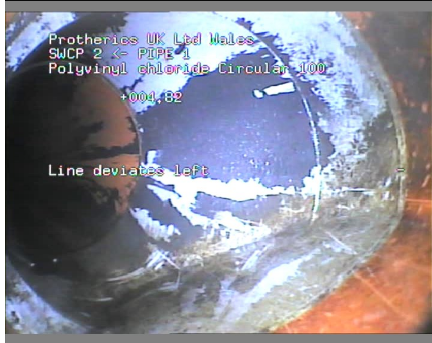
Photo: 26_26__A.JPG 4.82m, Line deviates left
