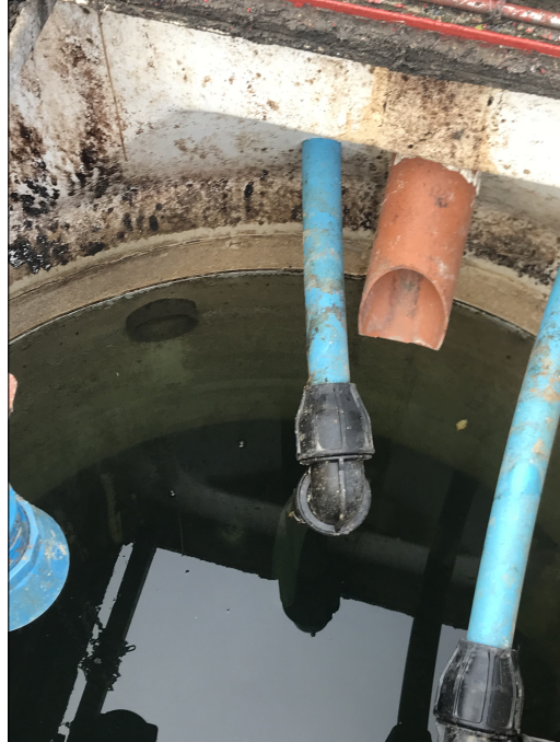
Photo: TANK Pipe from NRV Underwater.JPG 0m, General remark
