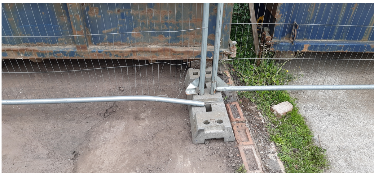
Photo 3 - Close up of Photo 2 regarding section of fencing not secured and damaged
