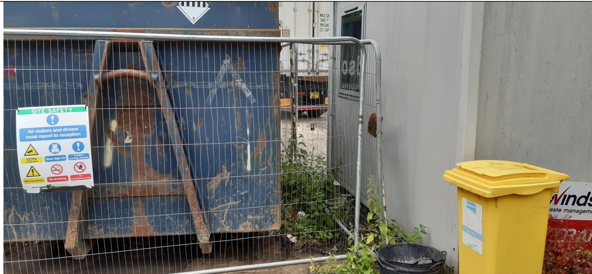
Photo 2 - Section of fencing not secured and damaged (bottom right)
