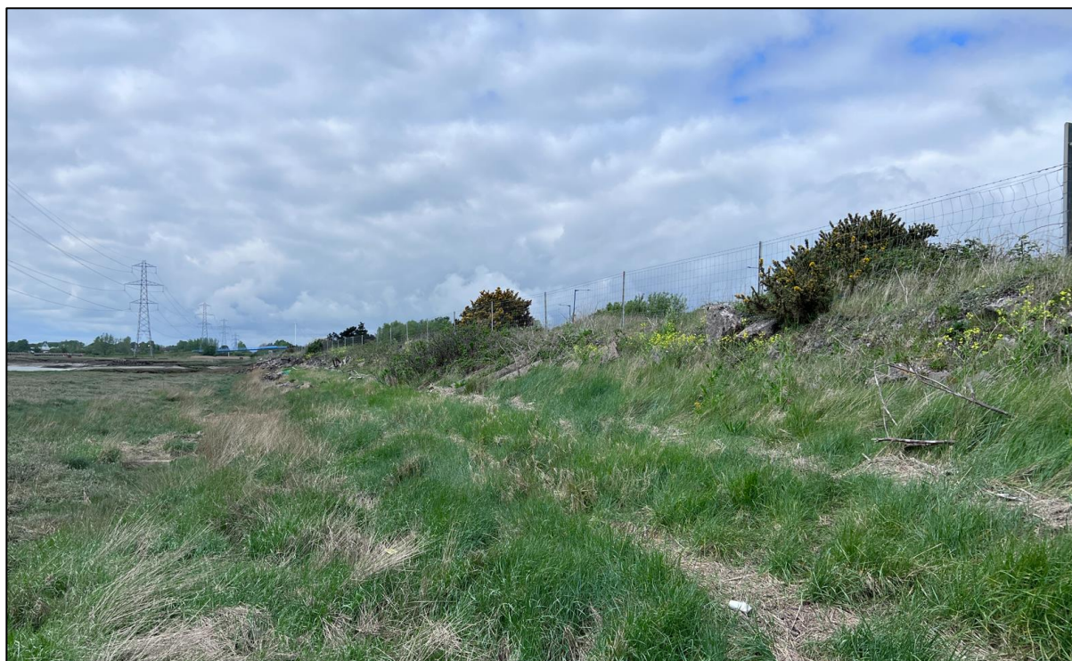
Figure 6: Section A embankment facing west.
