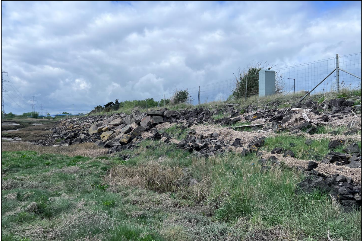
Figure 7: Section B rock armour and small loose embankment material.
