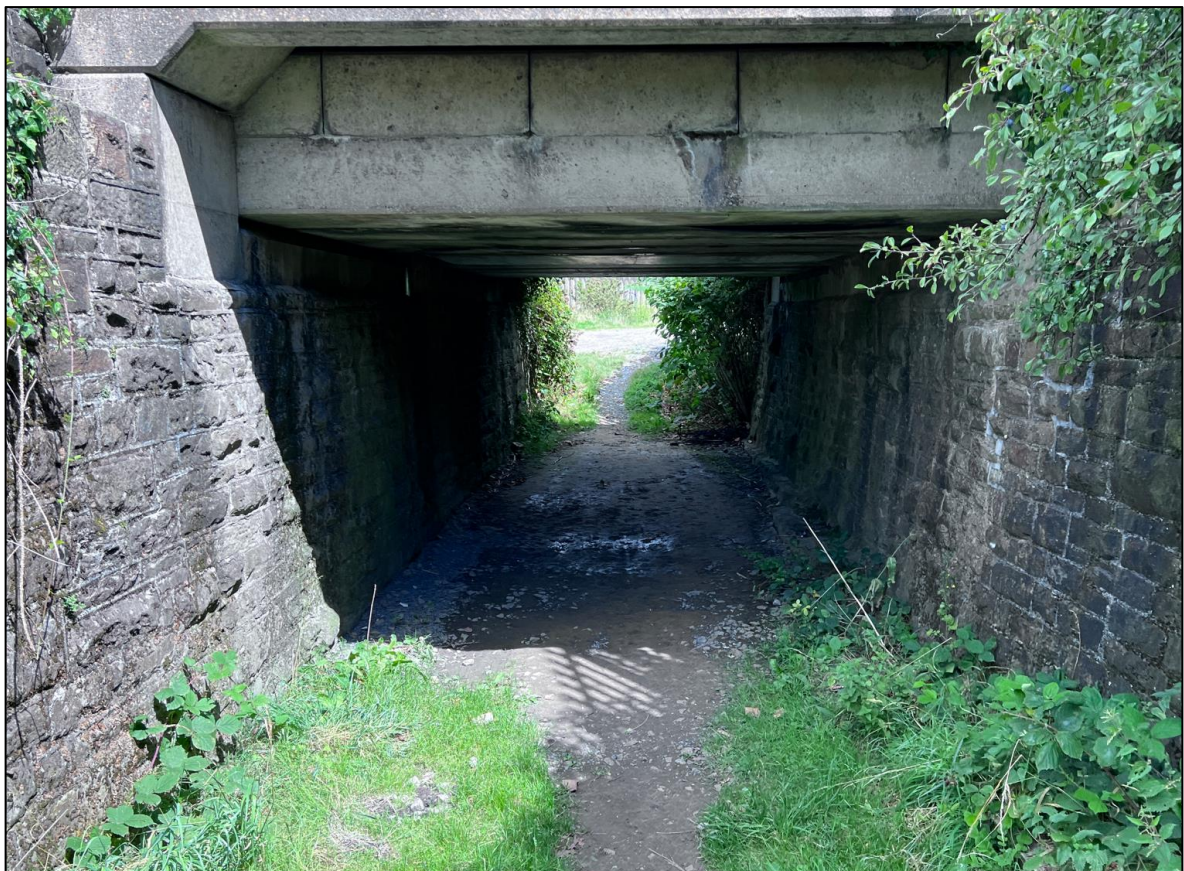
Figure 11: Underpass to be used.
