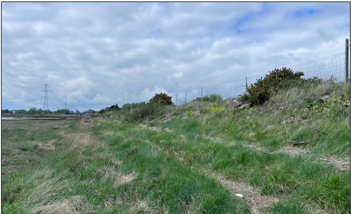
Figure 7: Section A embankment facing west.
