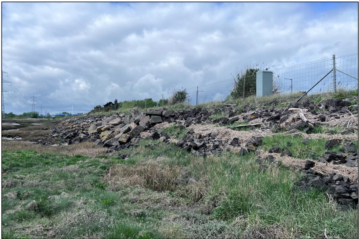
Figure 8: Section B rock armour and small loose embankment material.
