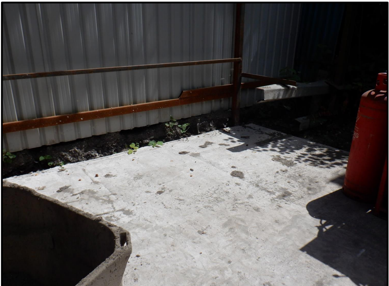
Photograph 7. Potentially contaminated rainfall dependent surface water may escape the edges of the impermeable pad and evading the drainage system.
