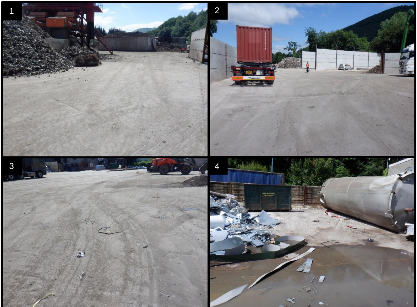
Photographs 1-4. Areas of newly constructed engineered concrete impermeable surface
