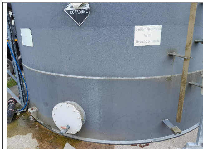
Suspect leak of possible contents
