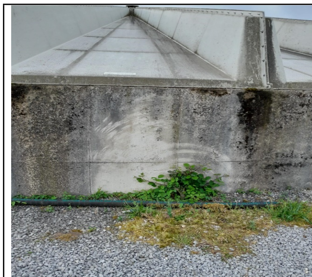
Suspect leak of possible contents
