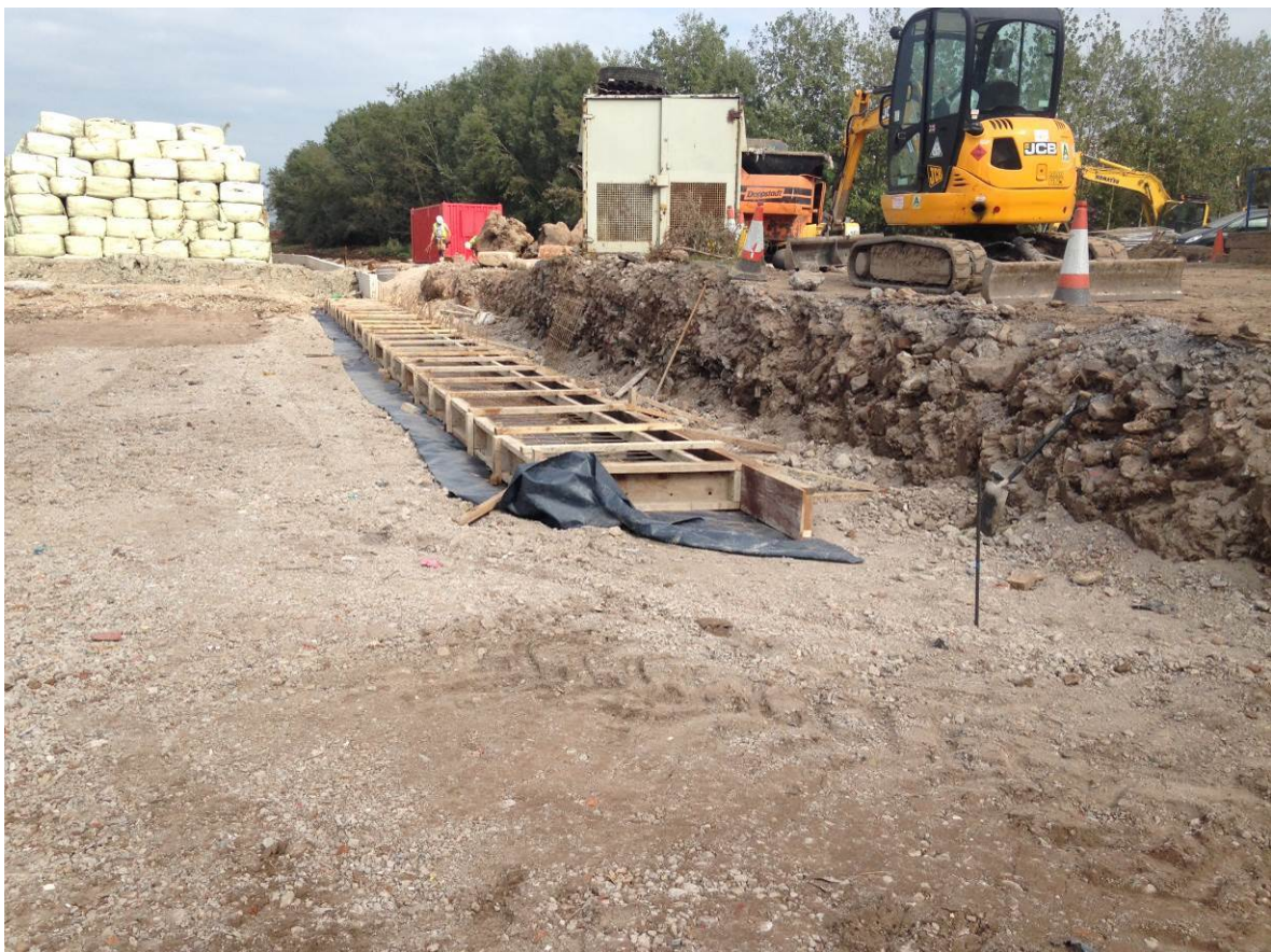
Shuttering for culvert base
