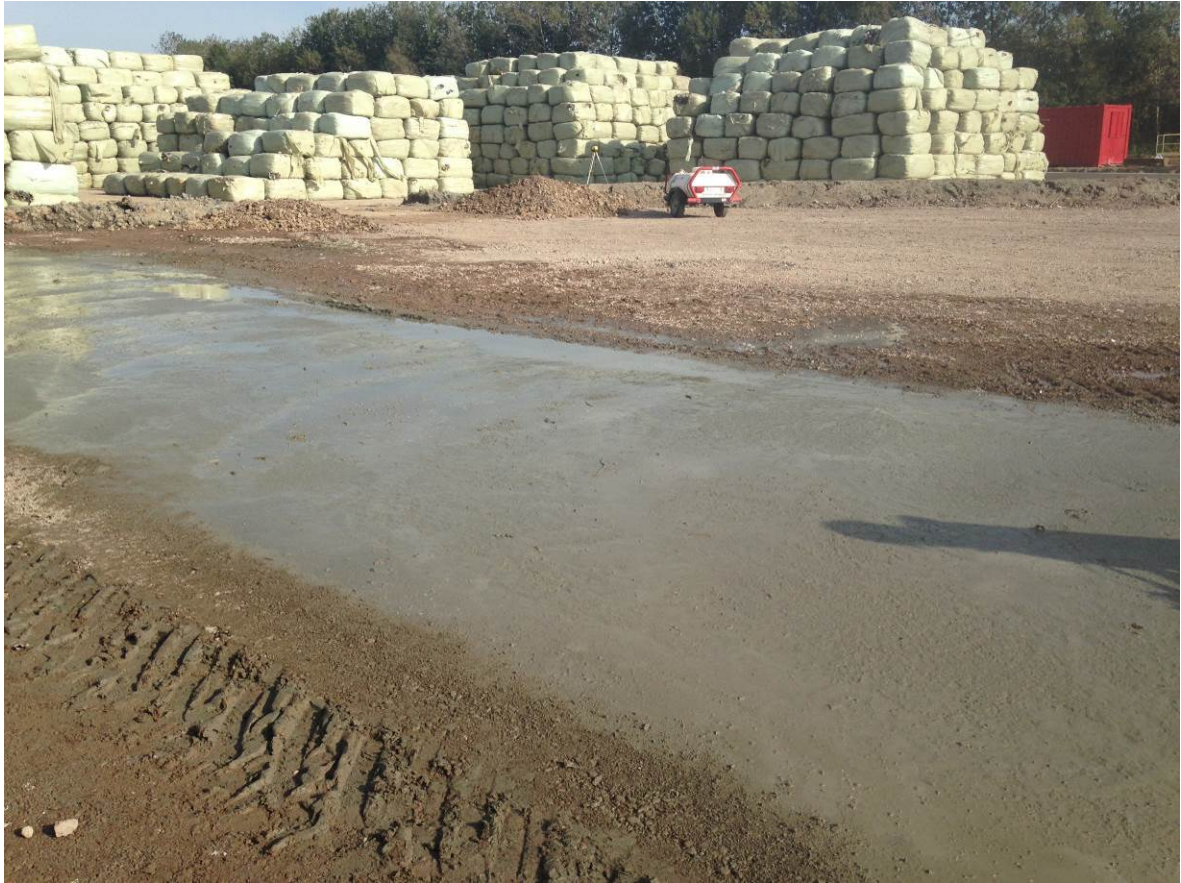
Finished Surface on Trial Pad
