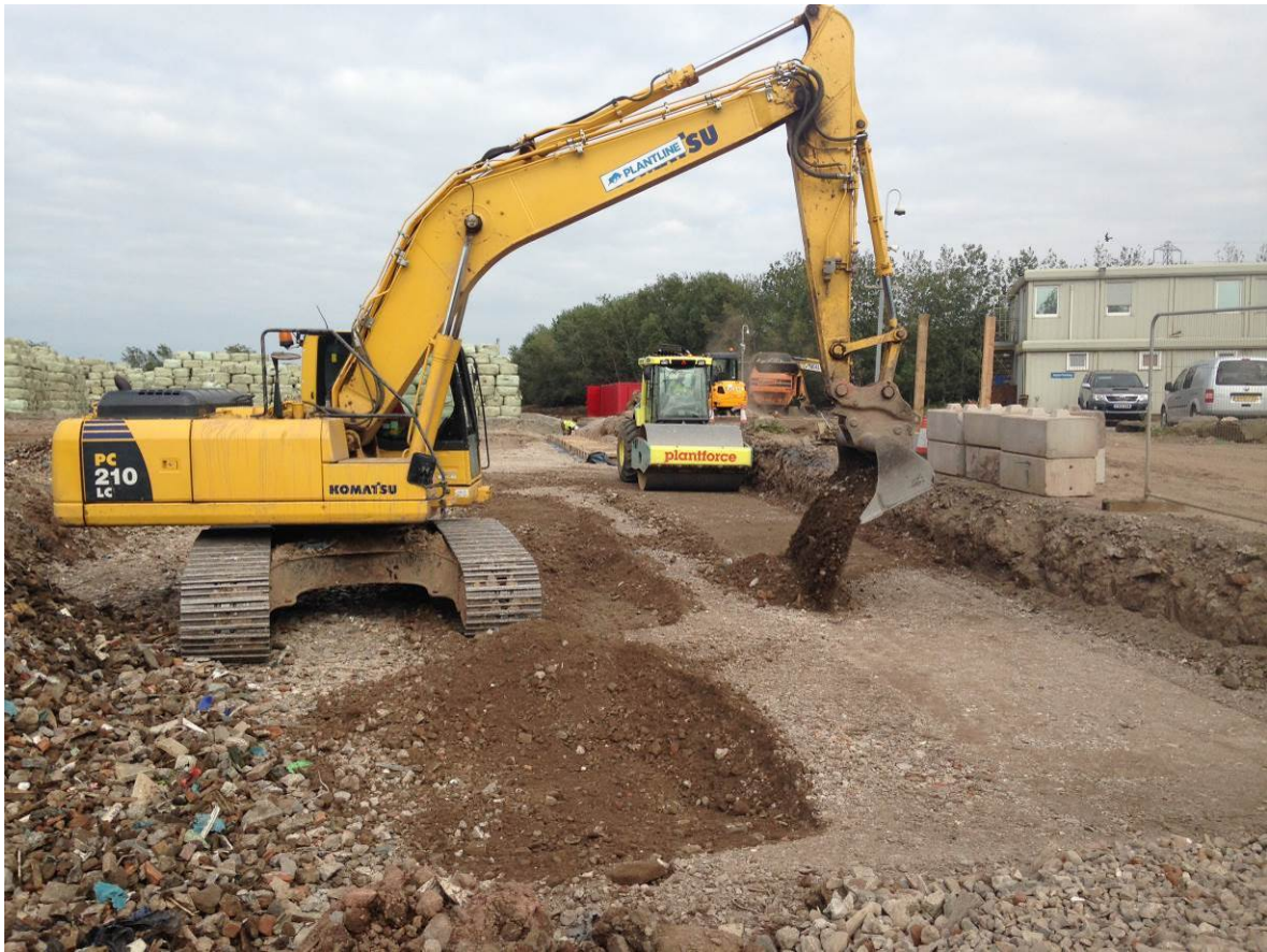
Preparation of subgrade for culvert
