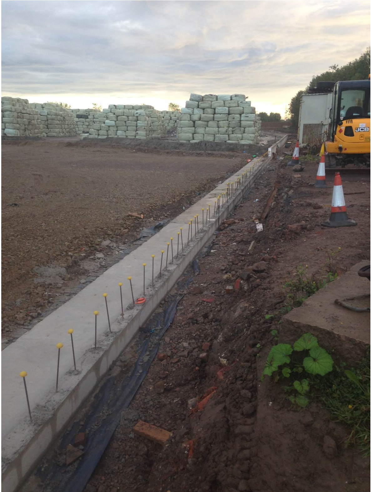
Culvert base with rebar upstands for headwall
