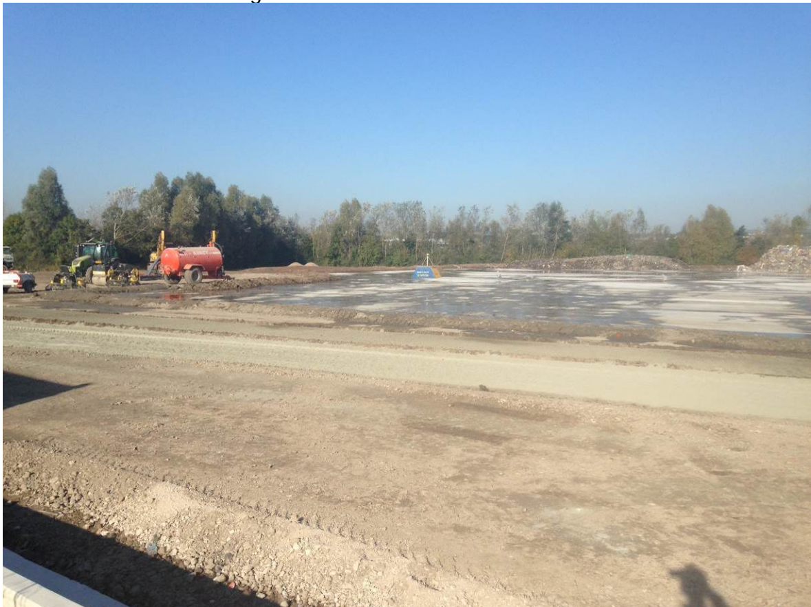
Spinning laser for control of levels/leachate held on pad surface
