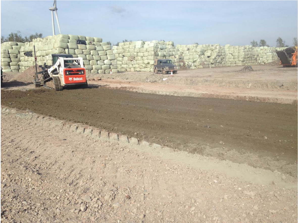
Trial Pad Construction
