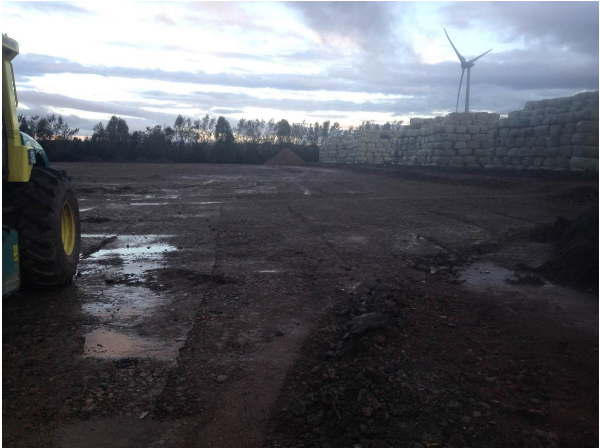
200mm Unbound Aggregate Layer
