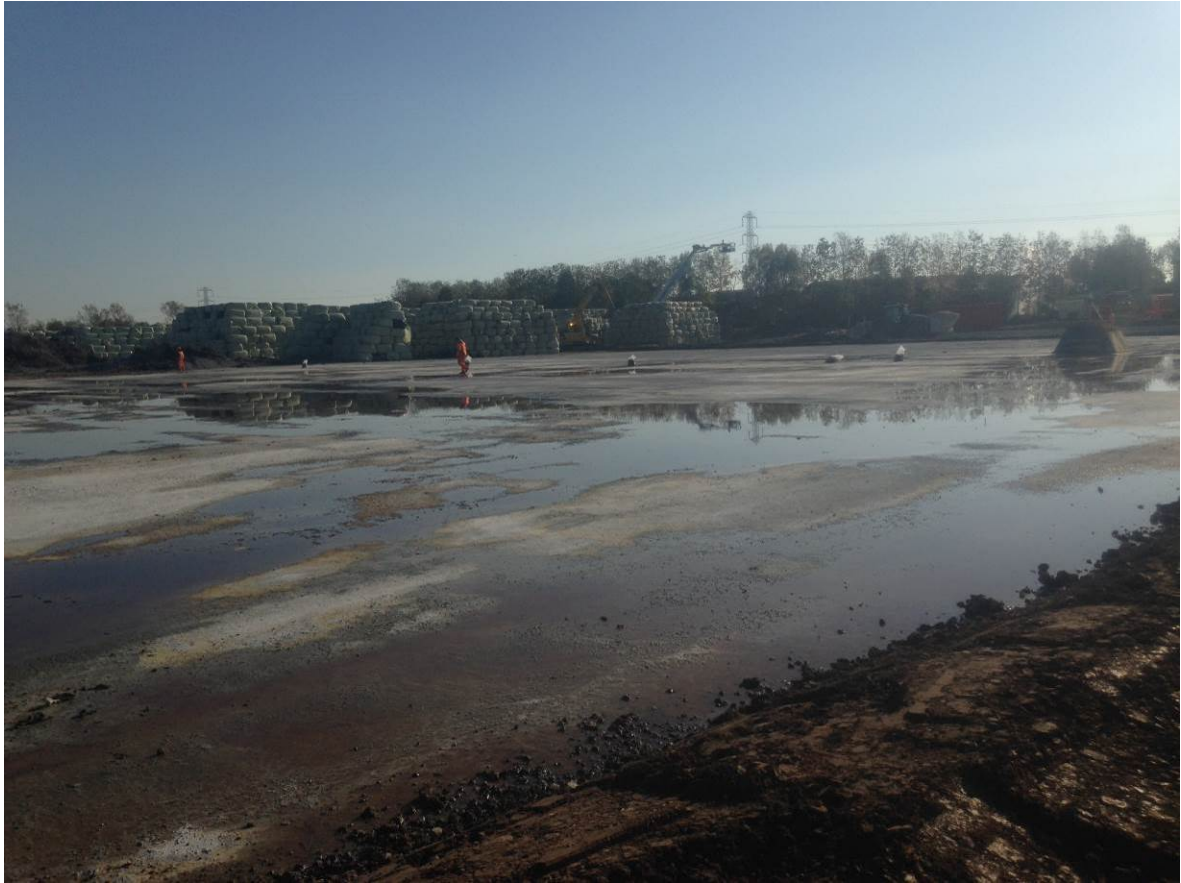
Temporary bund & leachate held on pad surface
