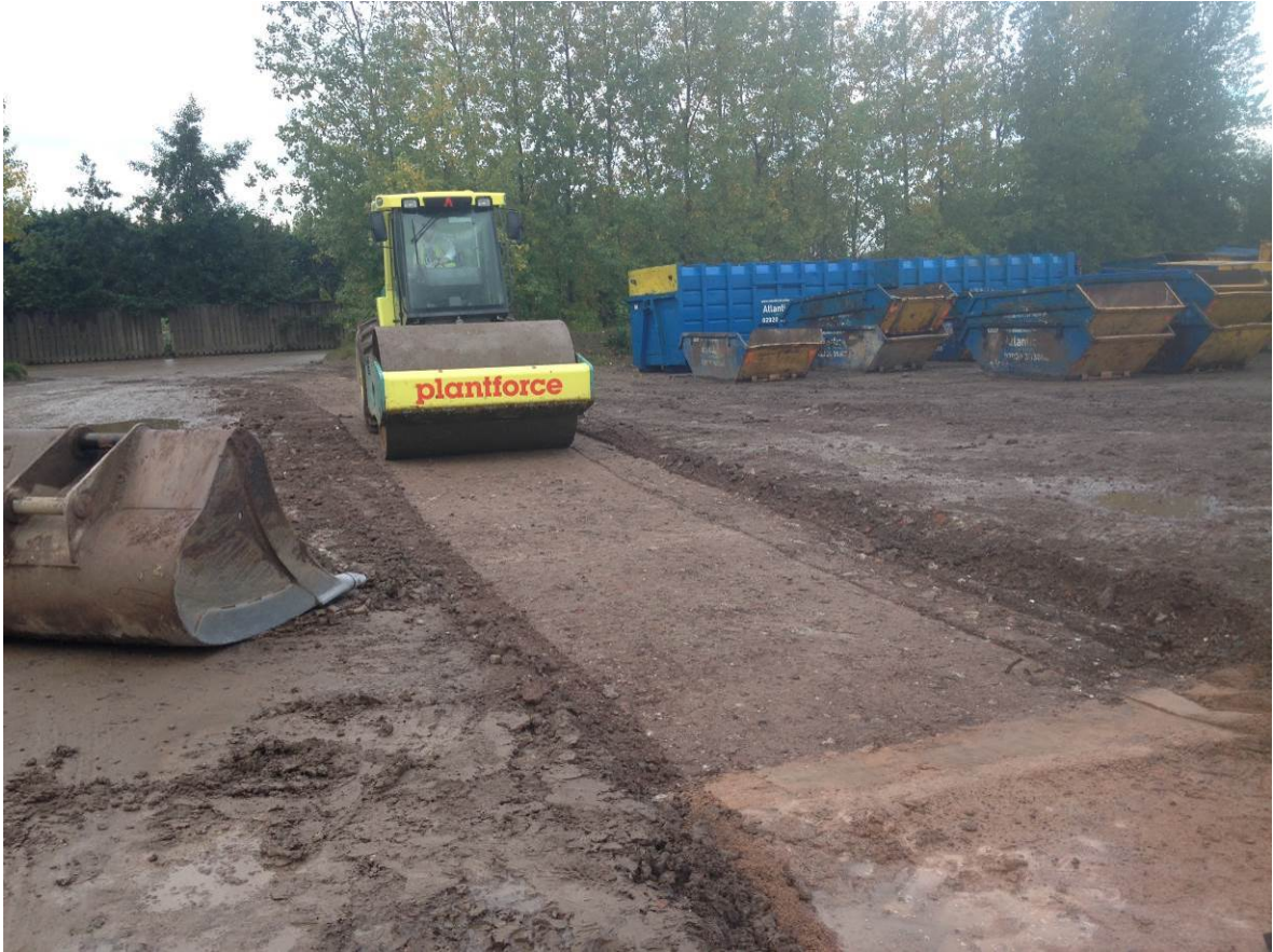
Preparation of subgrade for final culvert section
