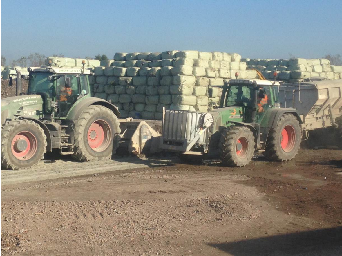
Left: Crushing aggregate & mixing cement powder Right: Placement of Cement Powder
