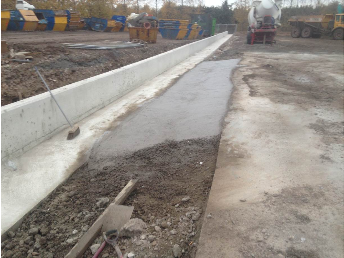
Connection of pad to culvert
