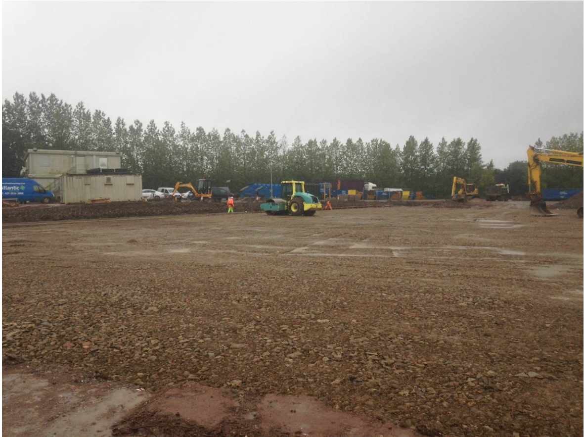
Placement of 200mm unbound layer
