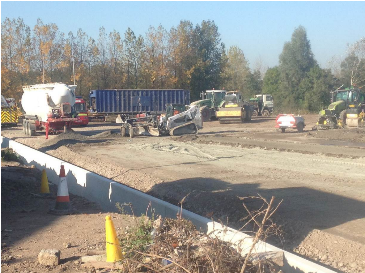
Bobcat with grading blade
