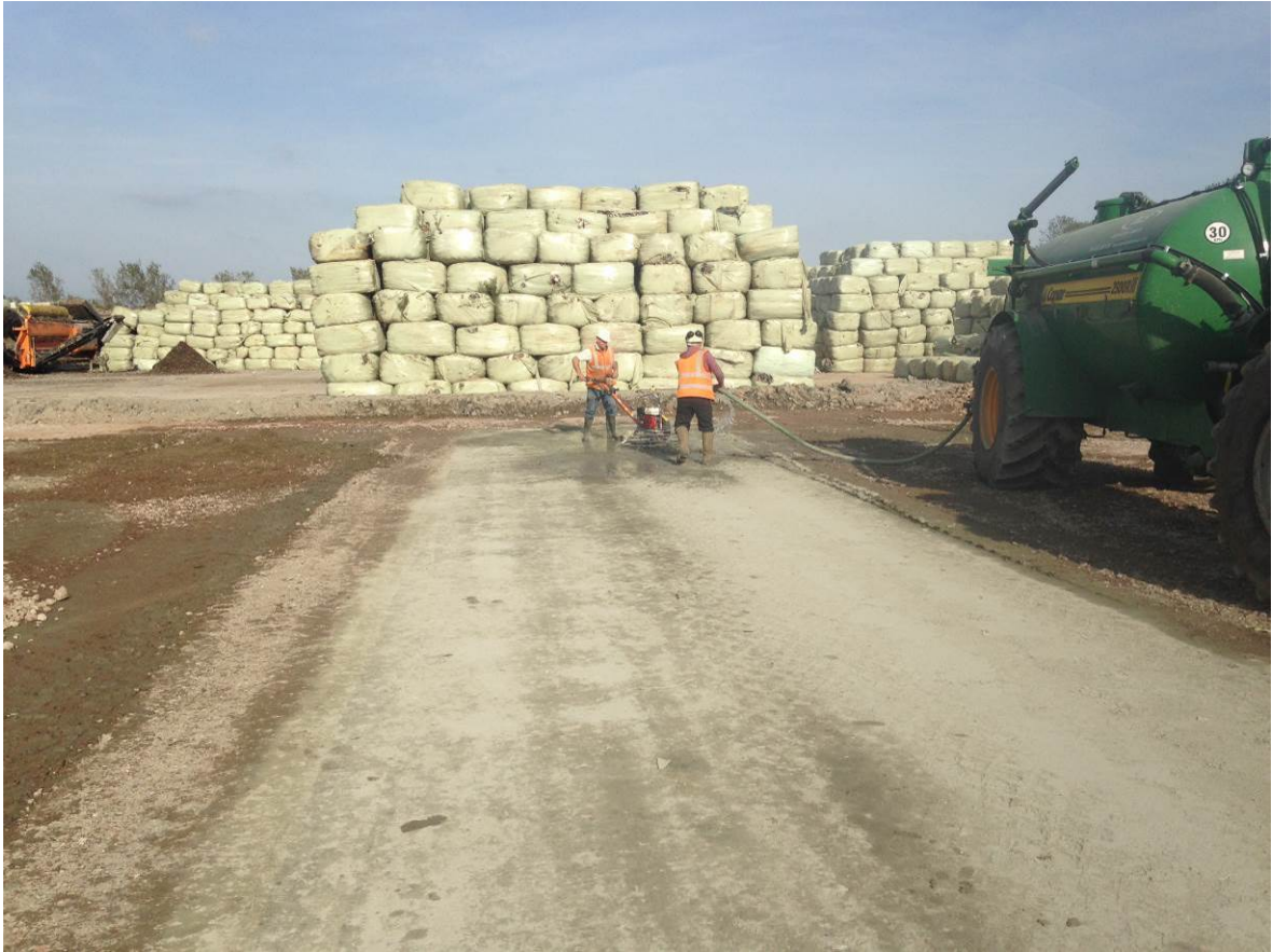
Power-floating to achieve finished surface
