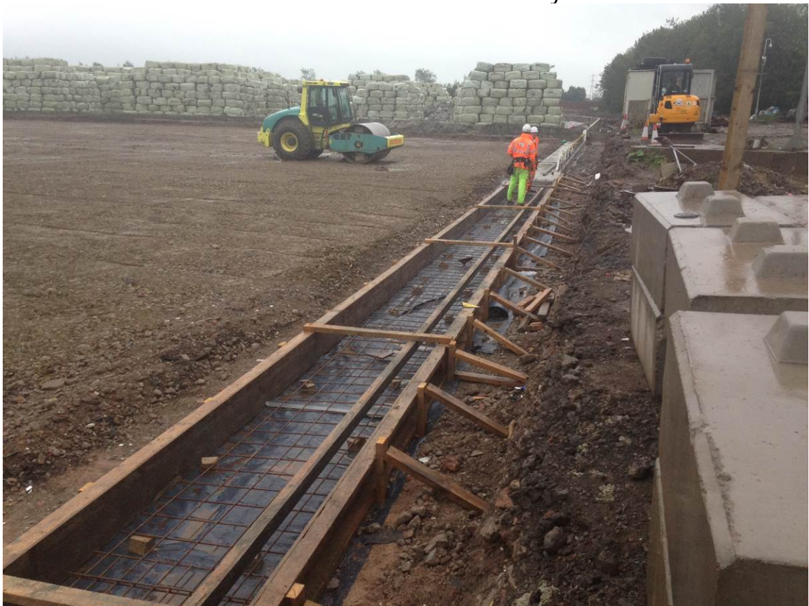
Shuttering with reinforcement bars for culvert base
