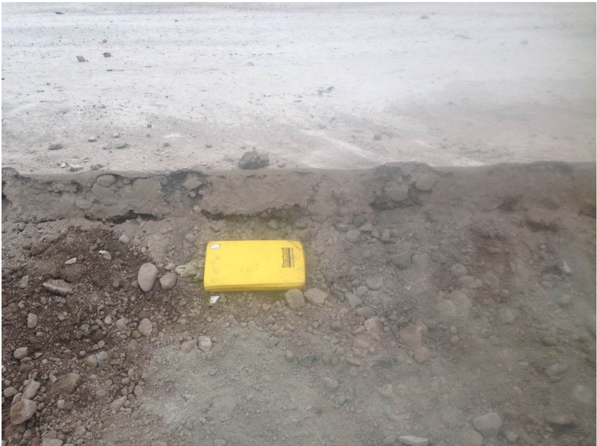
Exposed edge of pad after 1 st cut
