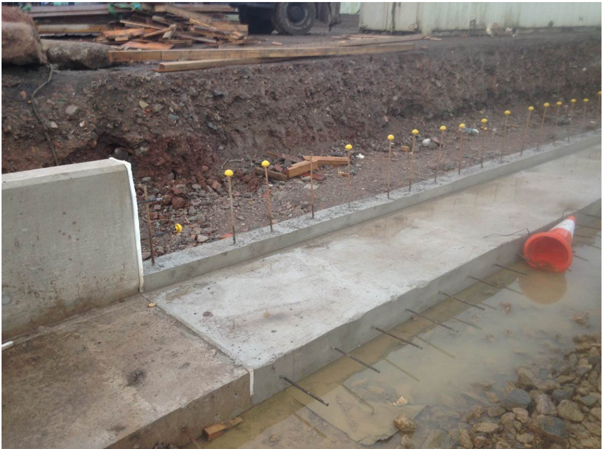
Connection between Phase 1 & Phase 2 Culvert
