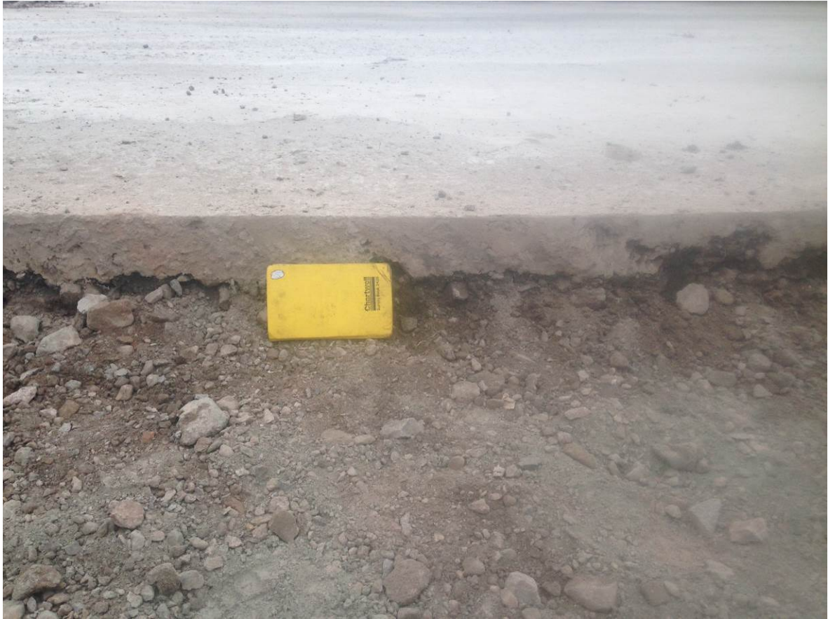
Exposed edge of pad after 1 st cut
