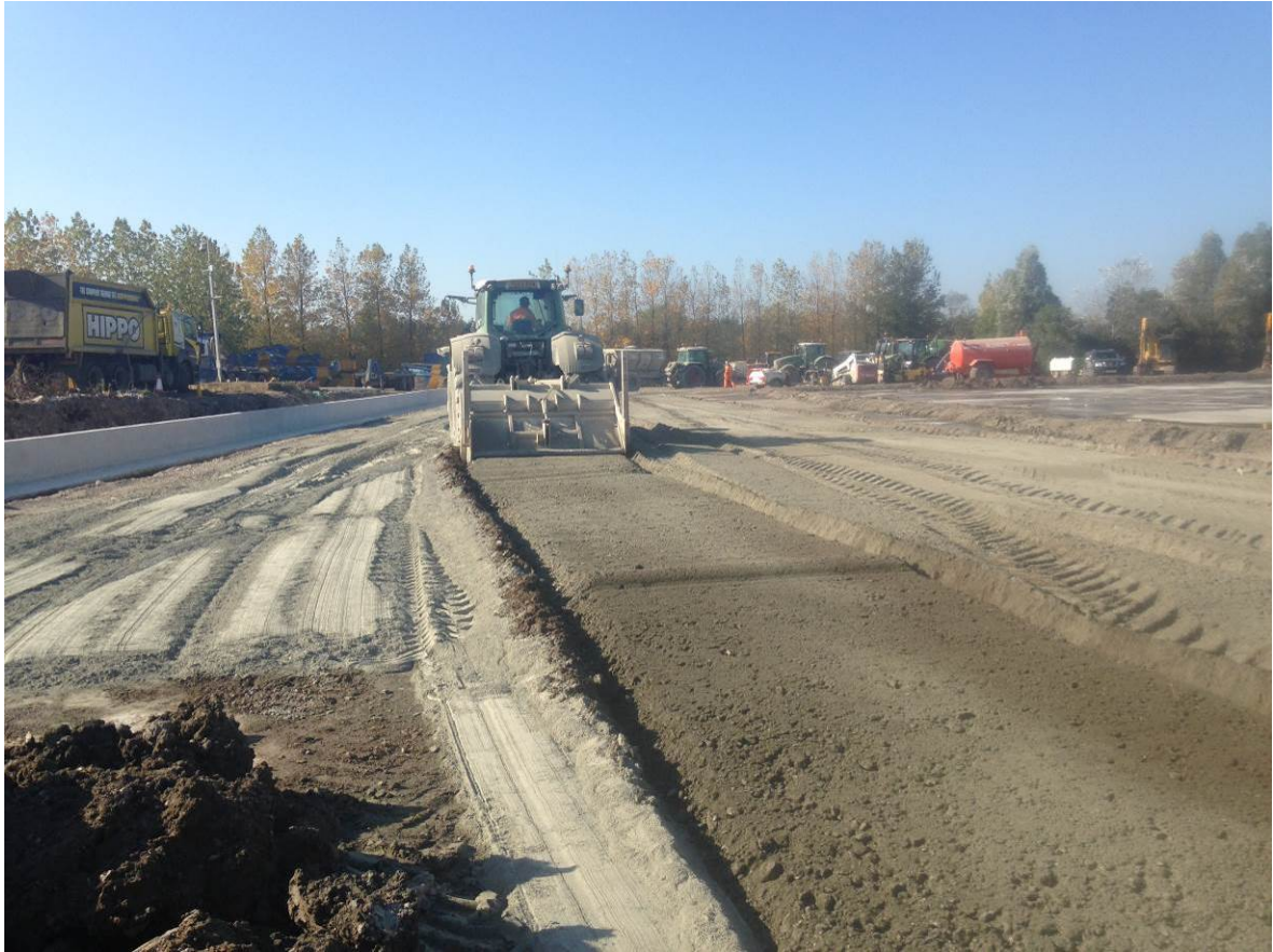
Crushing aggregate & mixing cement powder
