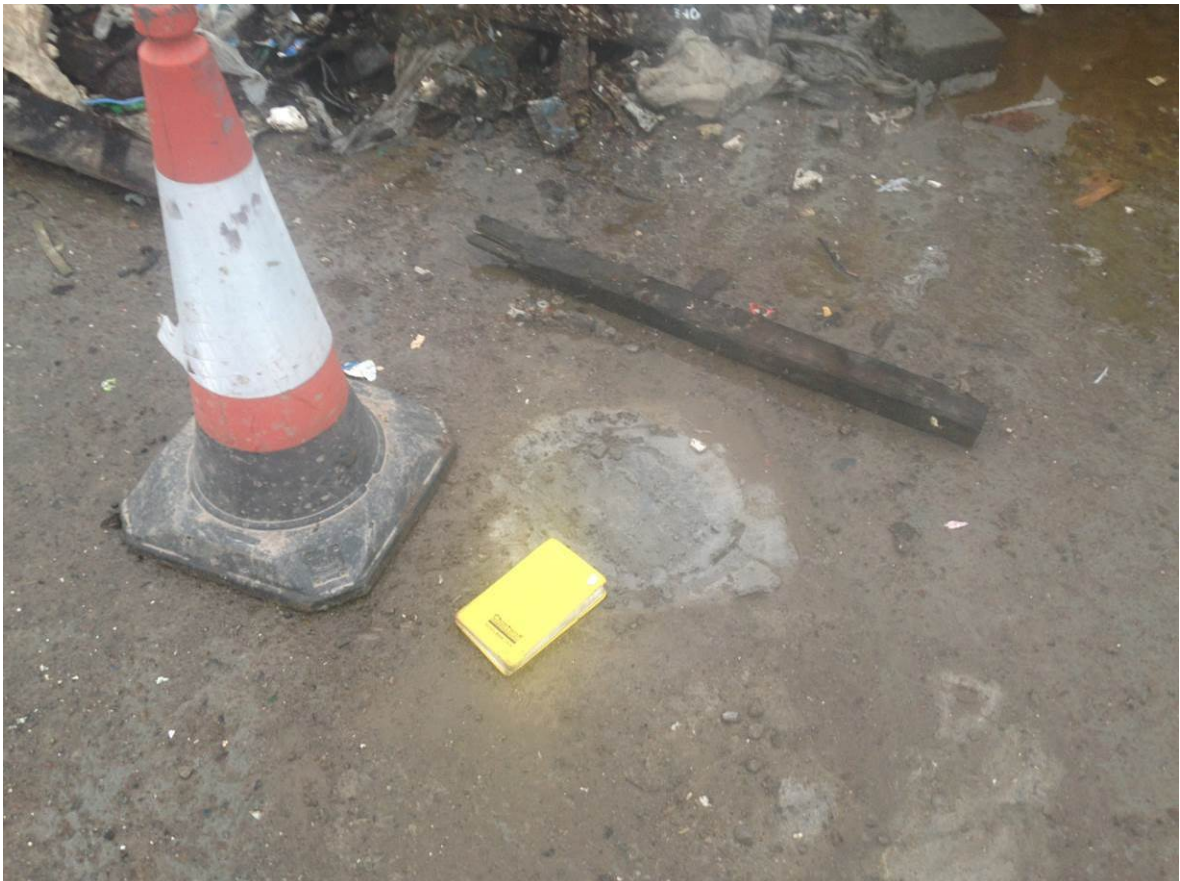
Backfilled borehole
