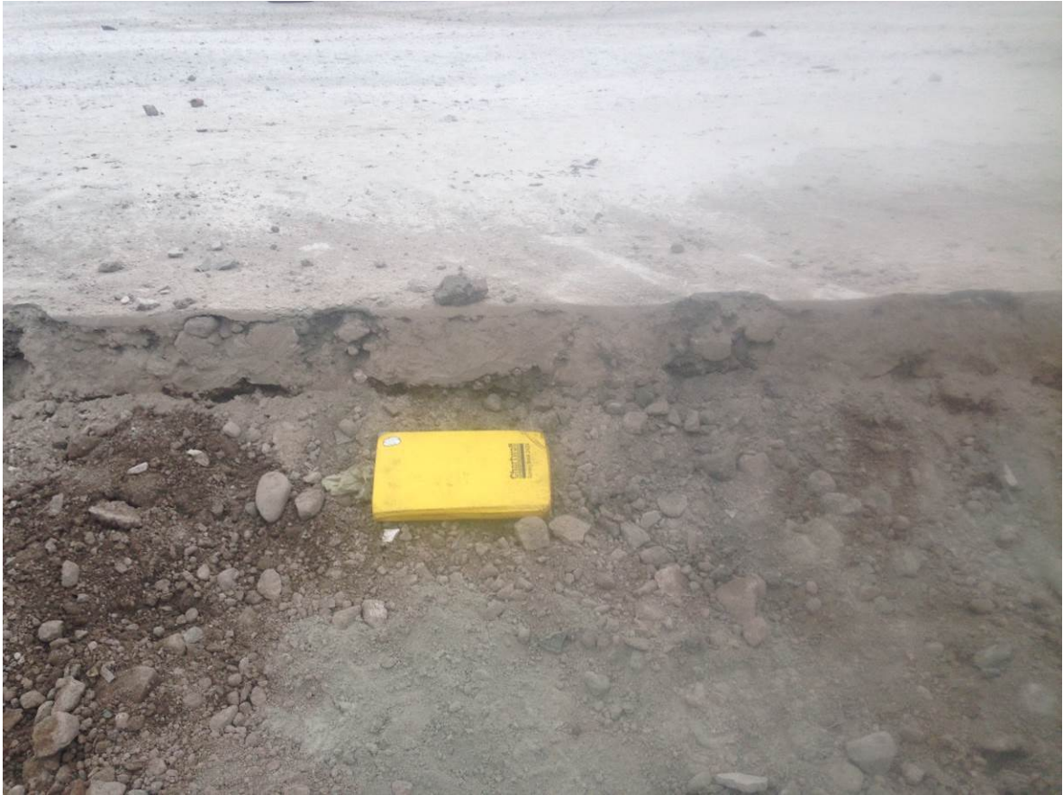
Exposed edge of pad after 1 st cut
