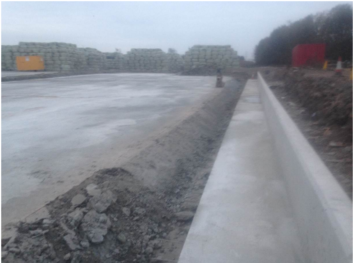
Edge of pad to be cut away
