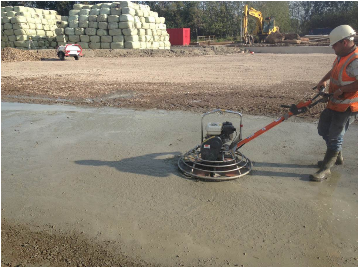
Power-floating to achieve finished surface
