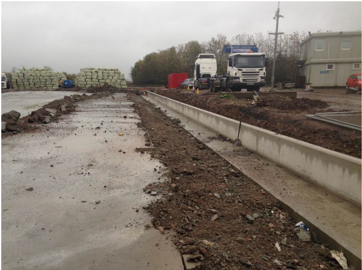
Edge of pad after 2 nd cut
