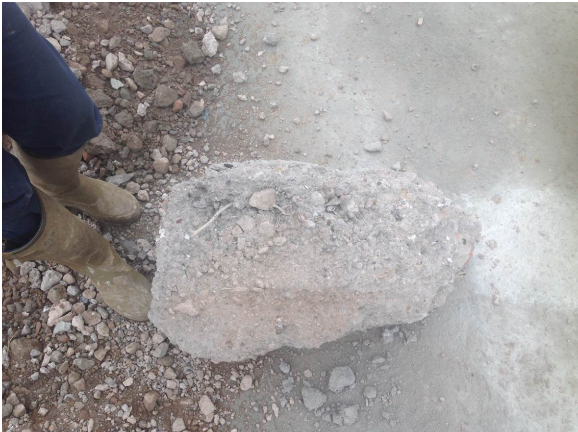
Bound aggregate excavated from edge of pad
