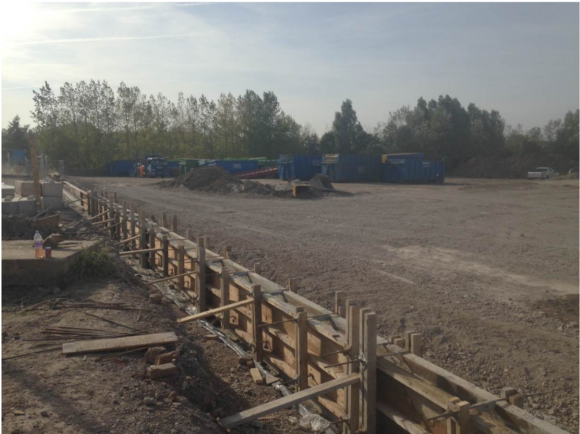
Shuttering for headwall
