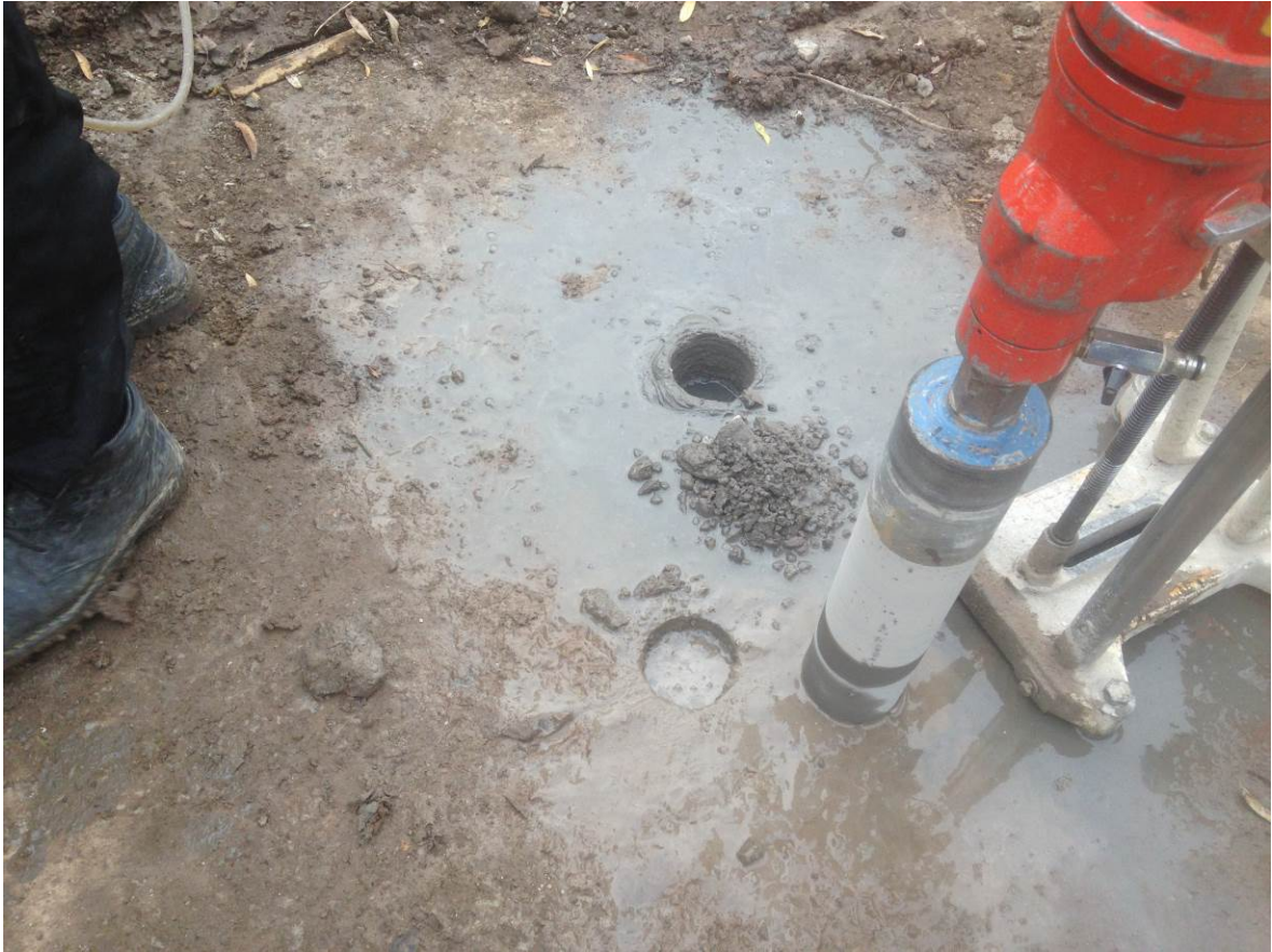
Coring of Phase 2 – Core 4A&B
