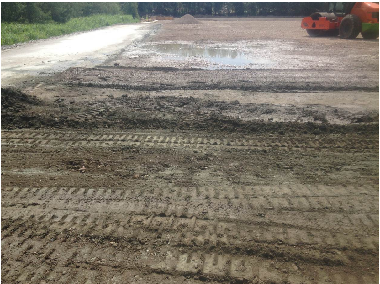
Crushing/Mixing of aggregate and cement
