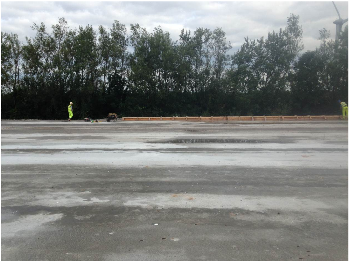
Shuttering for Kerb construction
