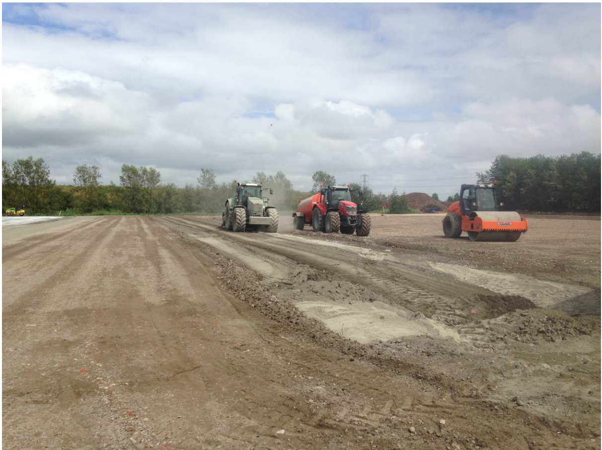
Wetting of surface and placement of cement
