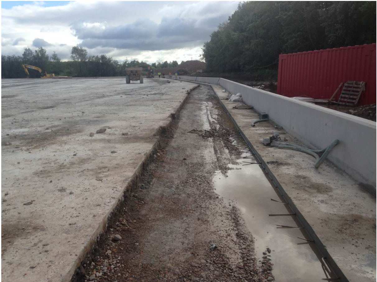
Prepared slab/drainage channel connection
