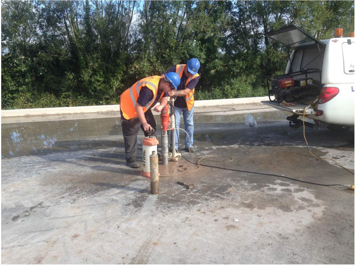
Coring carried out by Apex Testing Solutions
