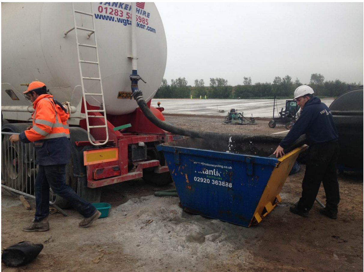
Dust suppression measures
