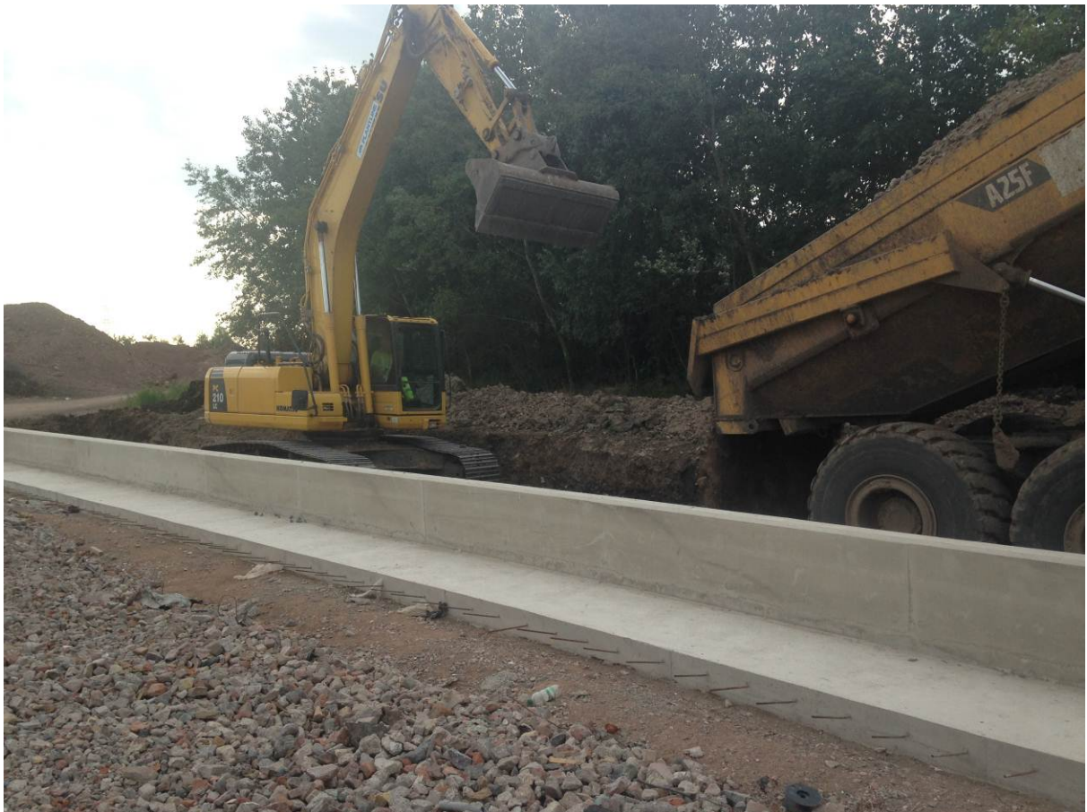
Construction of haul road
