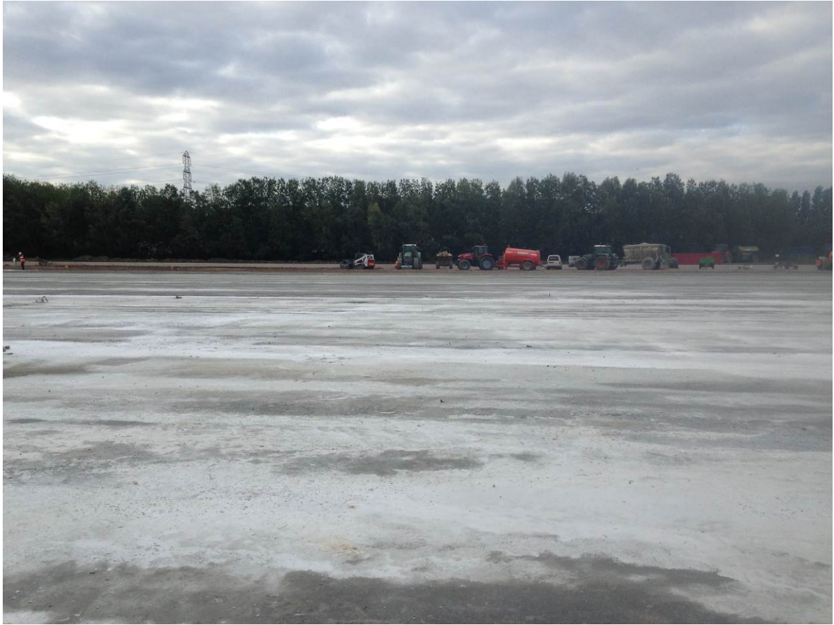
Final slab surface
