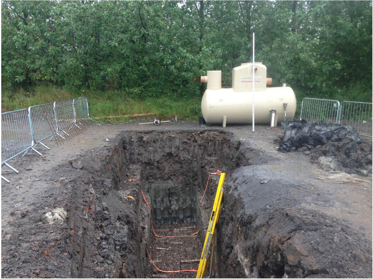
Excavation for oil interceptor installation
