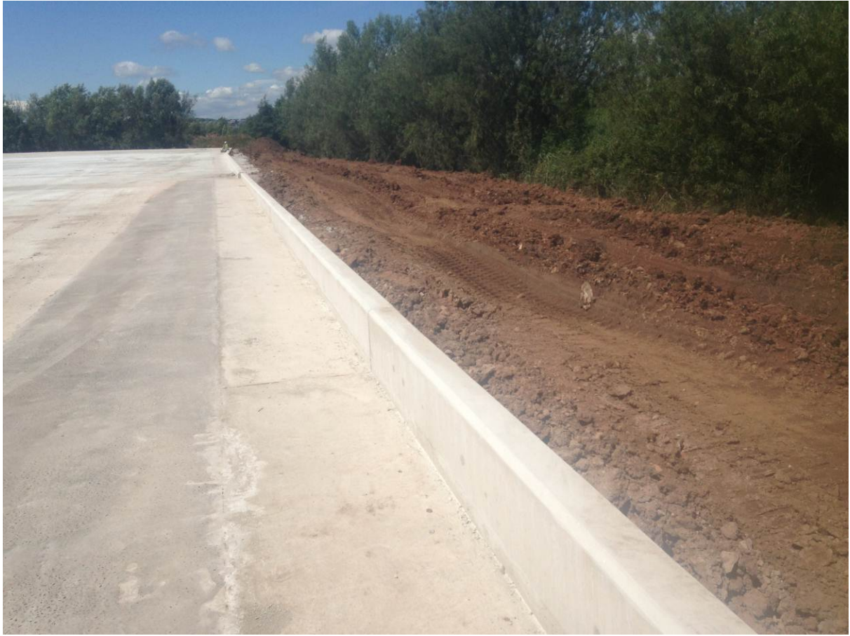
Connection of headwall return to slab
