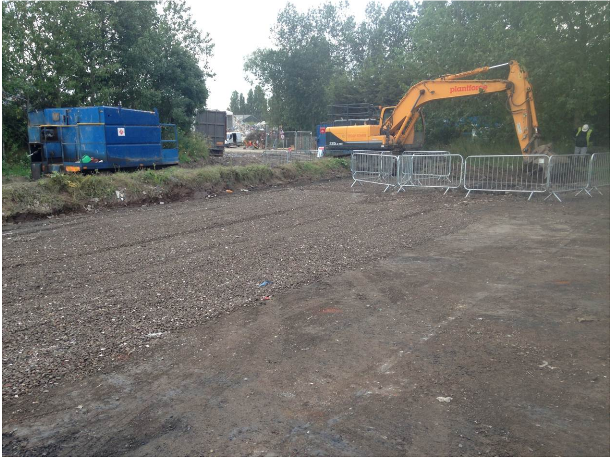
Reinstated car park area
