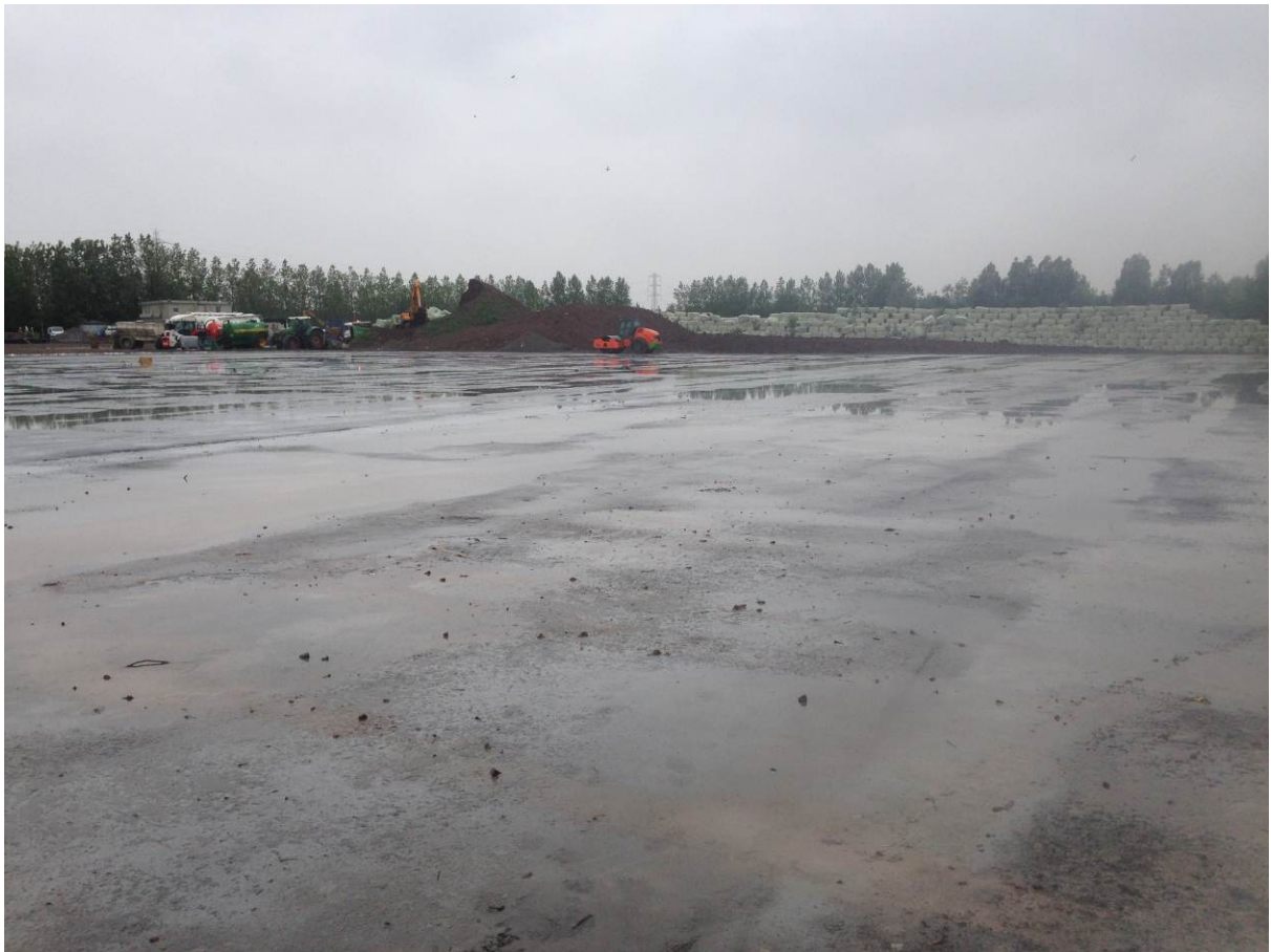
Final slab surface
