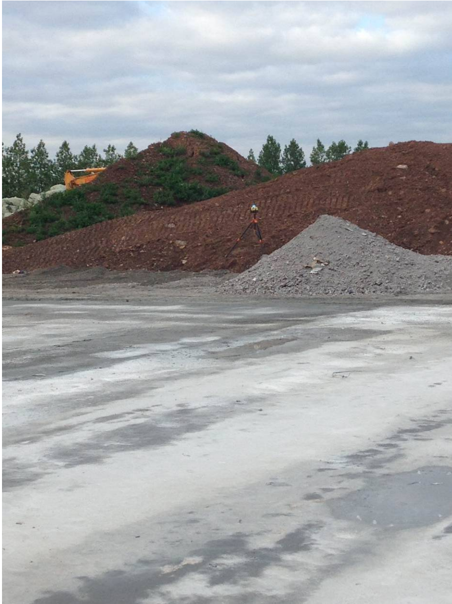
Spinning laser setup at change point of slab
