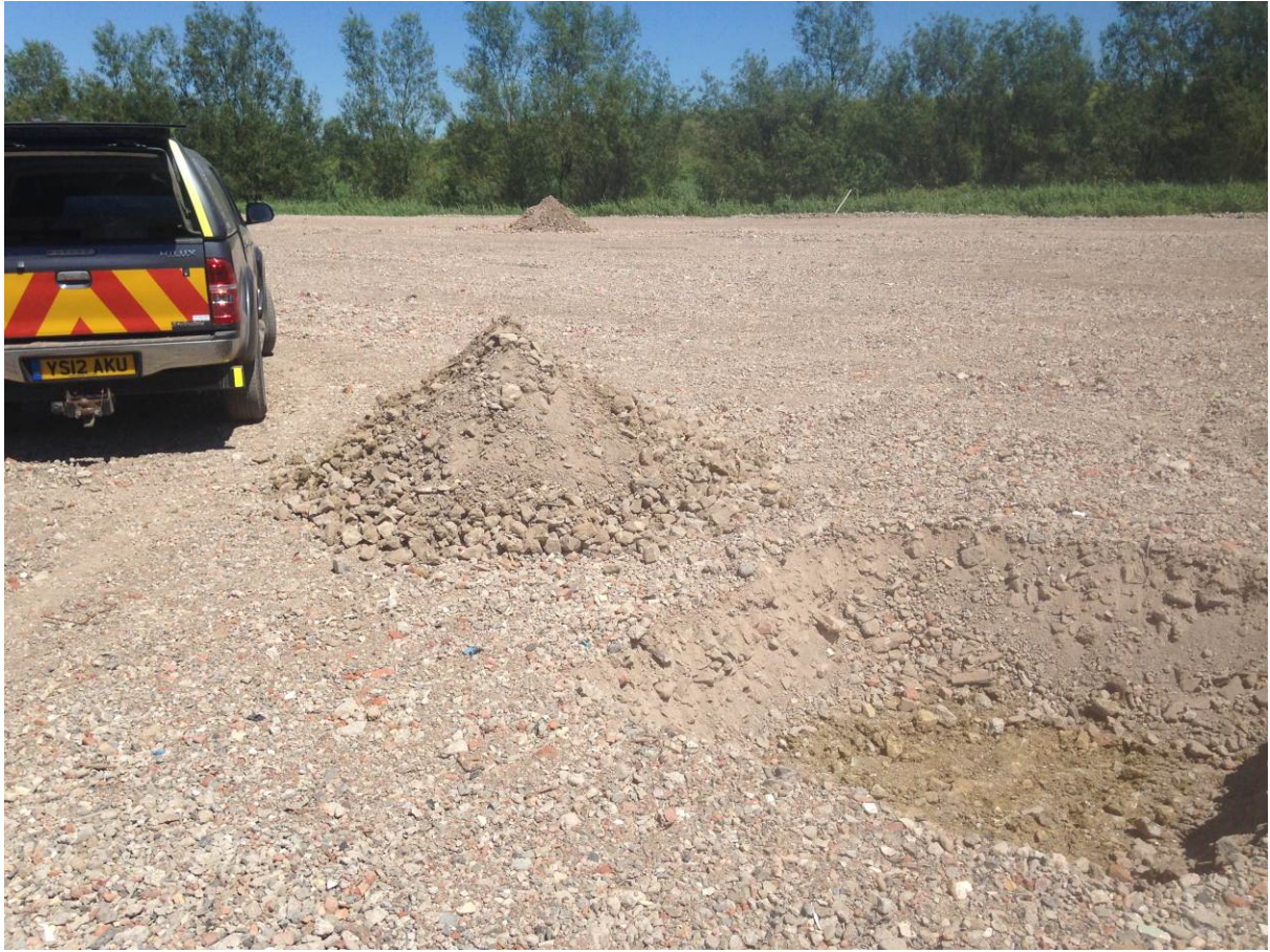
Trial Pit for CBR Testing
