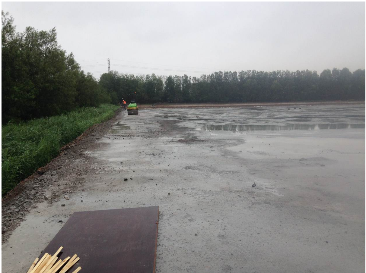
Final slab surface
