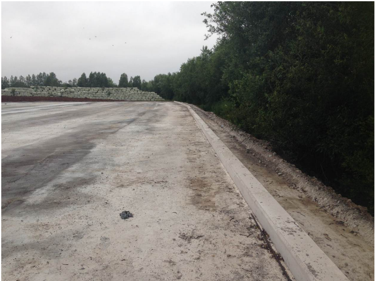
Finished Kerb on Northwest edge
