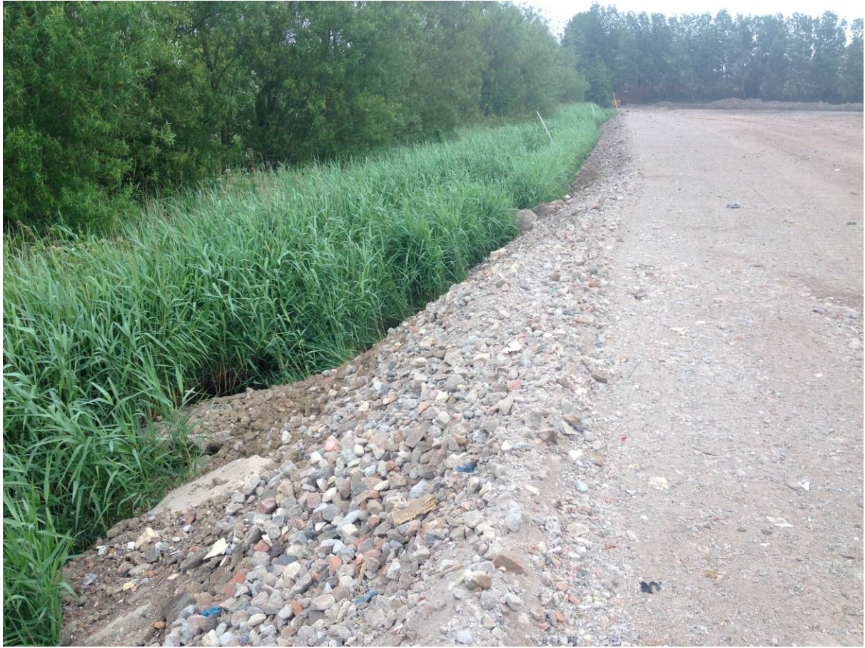
Northeast edge of prepared slab
