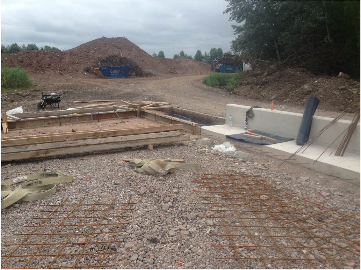
Shuttering in Eastern corner
