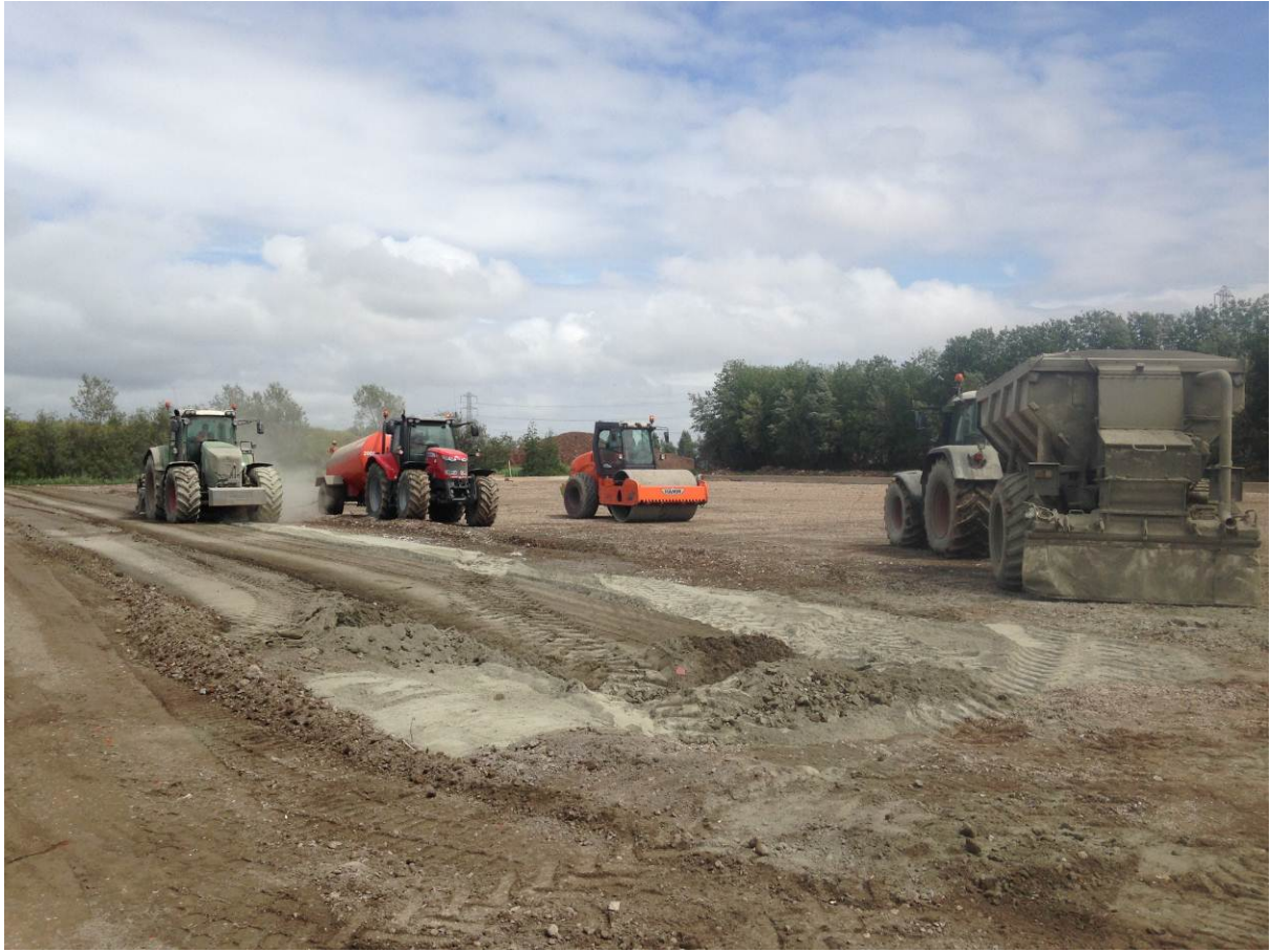
Wetting of surface and placement of cement
