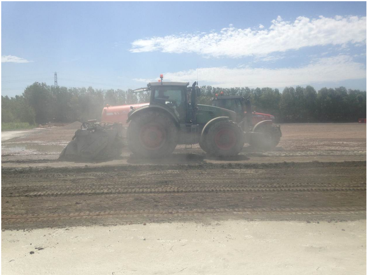
Crushing/Mixing of aggregate and cement
