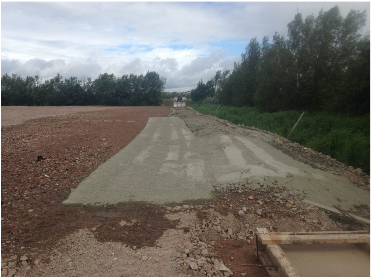
Cement powder placement on Northeast edge
