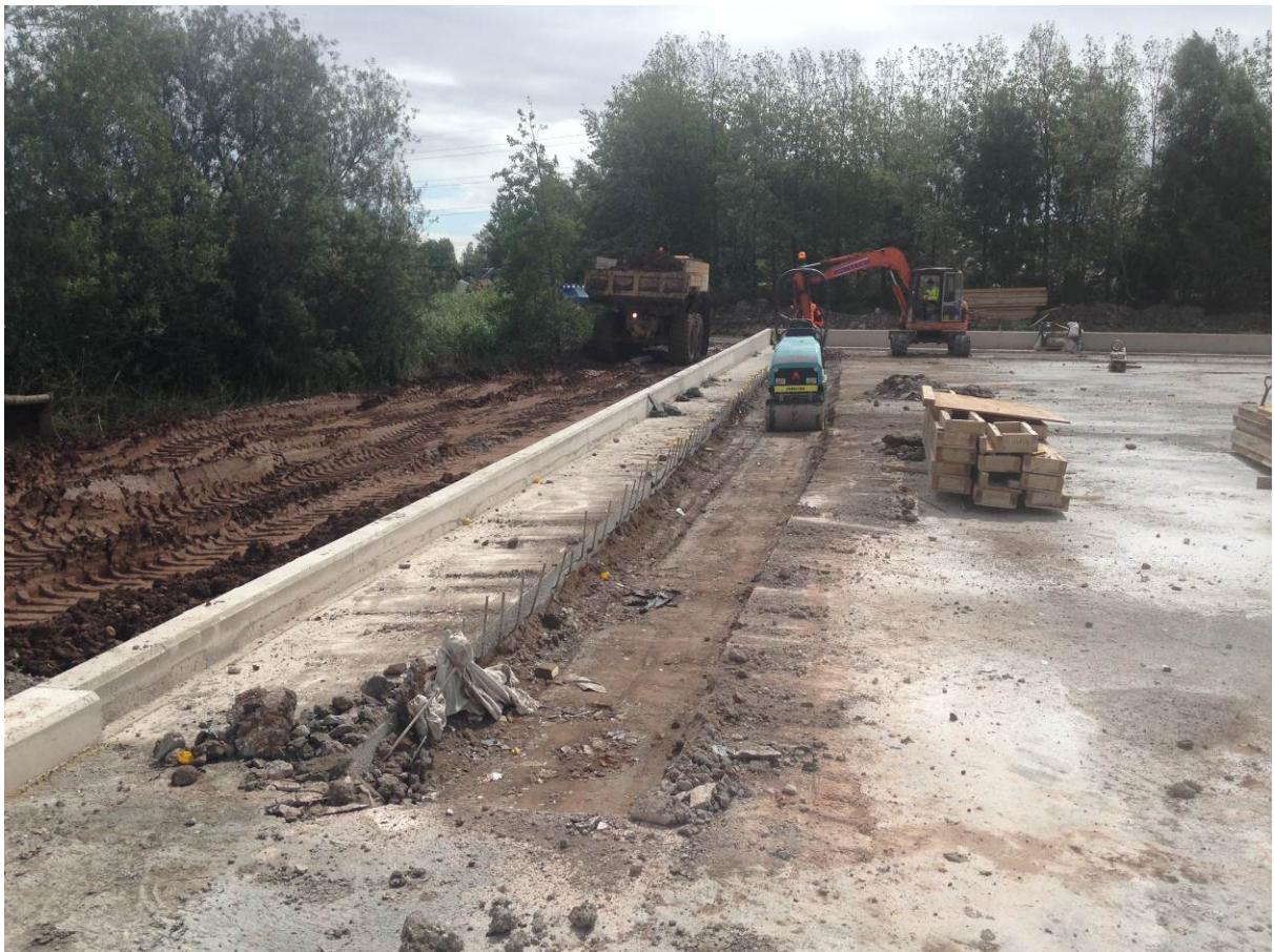
Preparation of drainage channel/slab join
