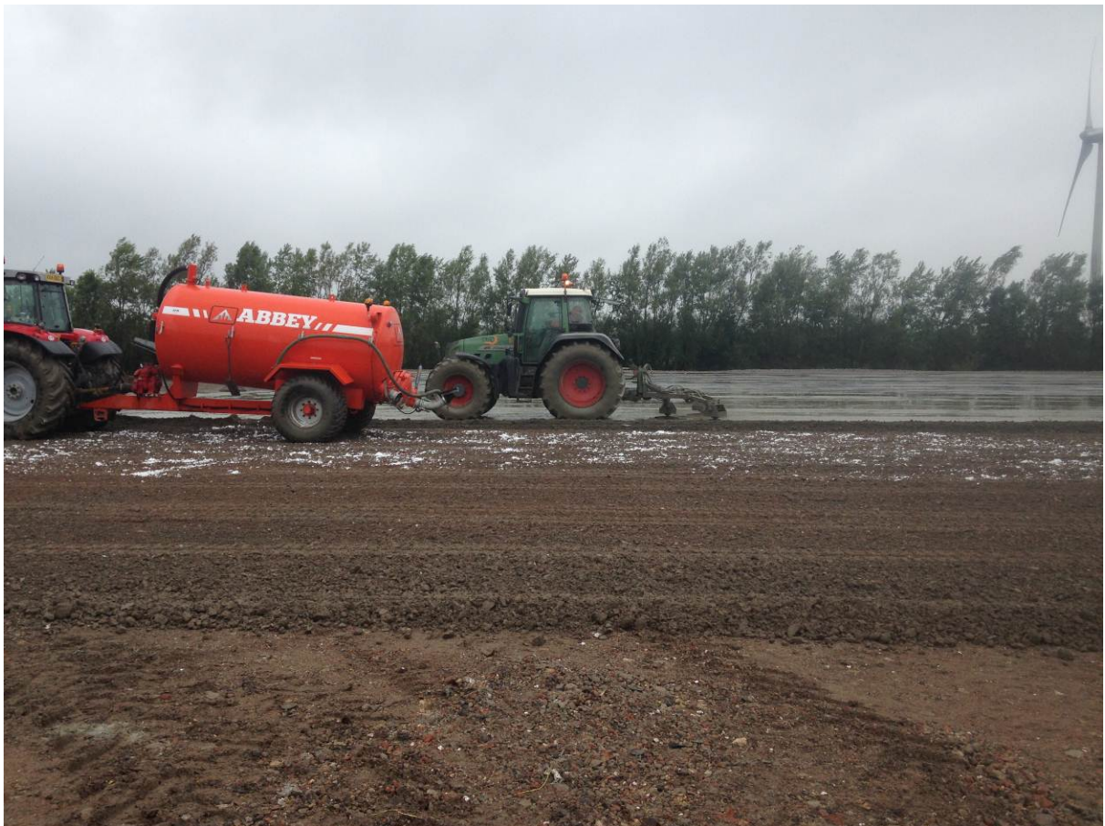
Wetting of surface and power floating
