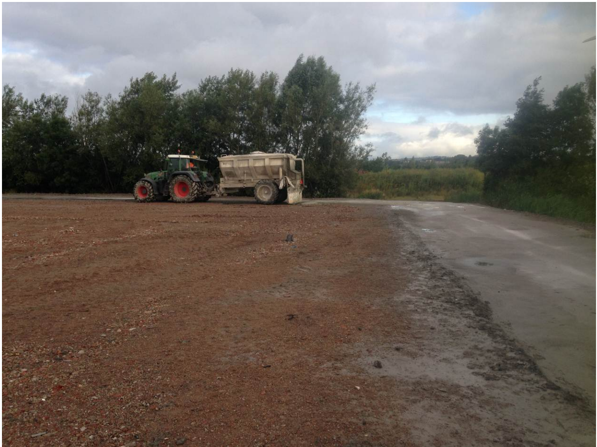
Spreading of cement powder
