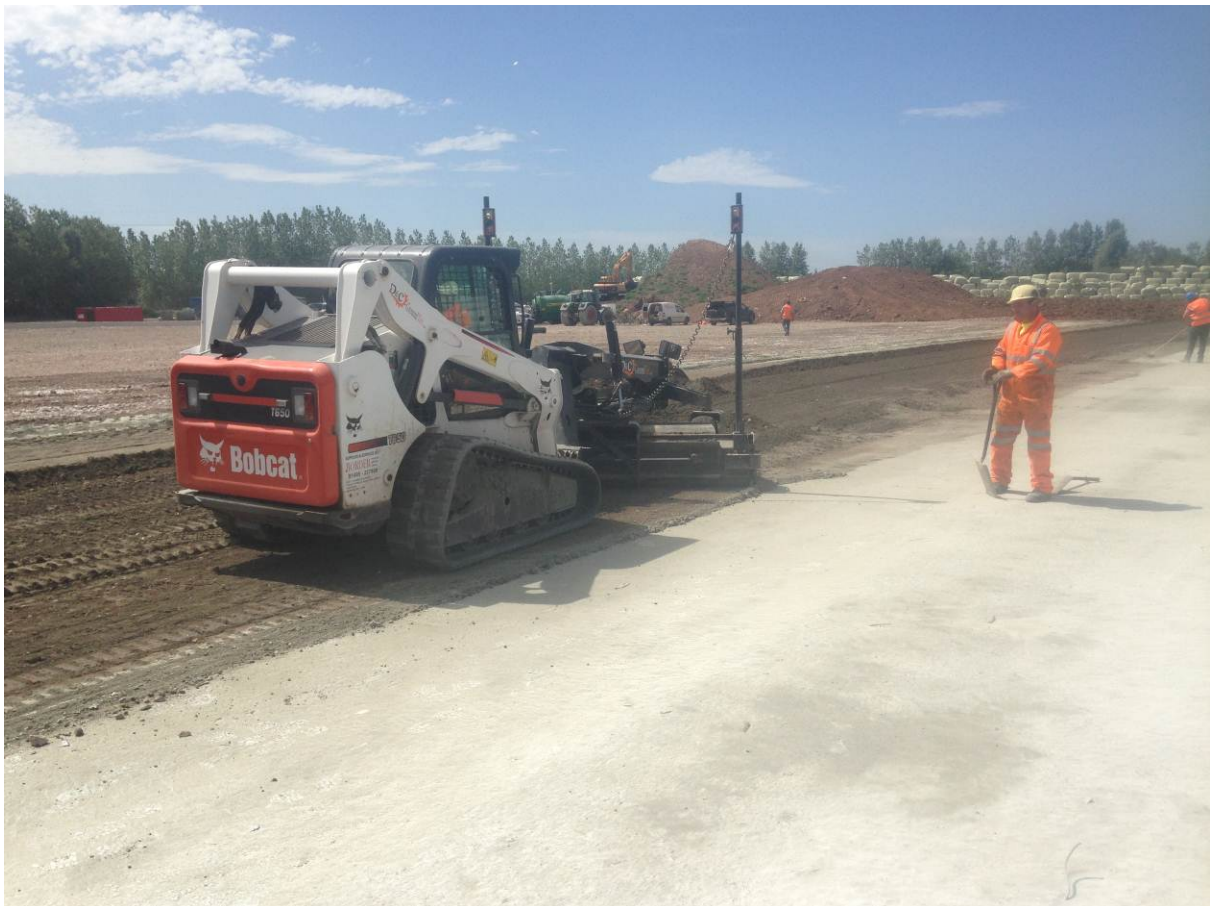
Grading of cement aggregate mix
