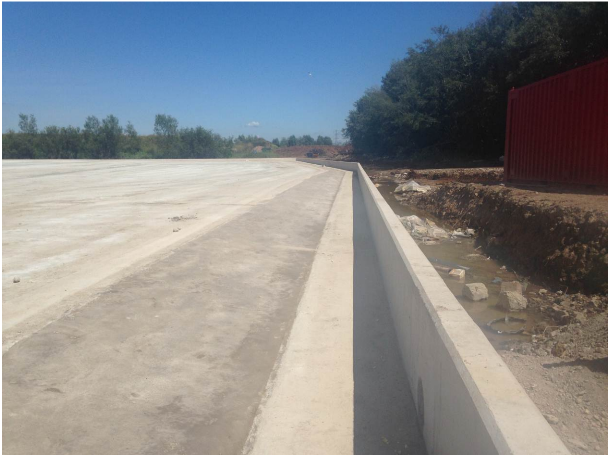
Connection of drainage channel and slab
