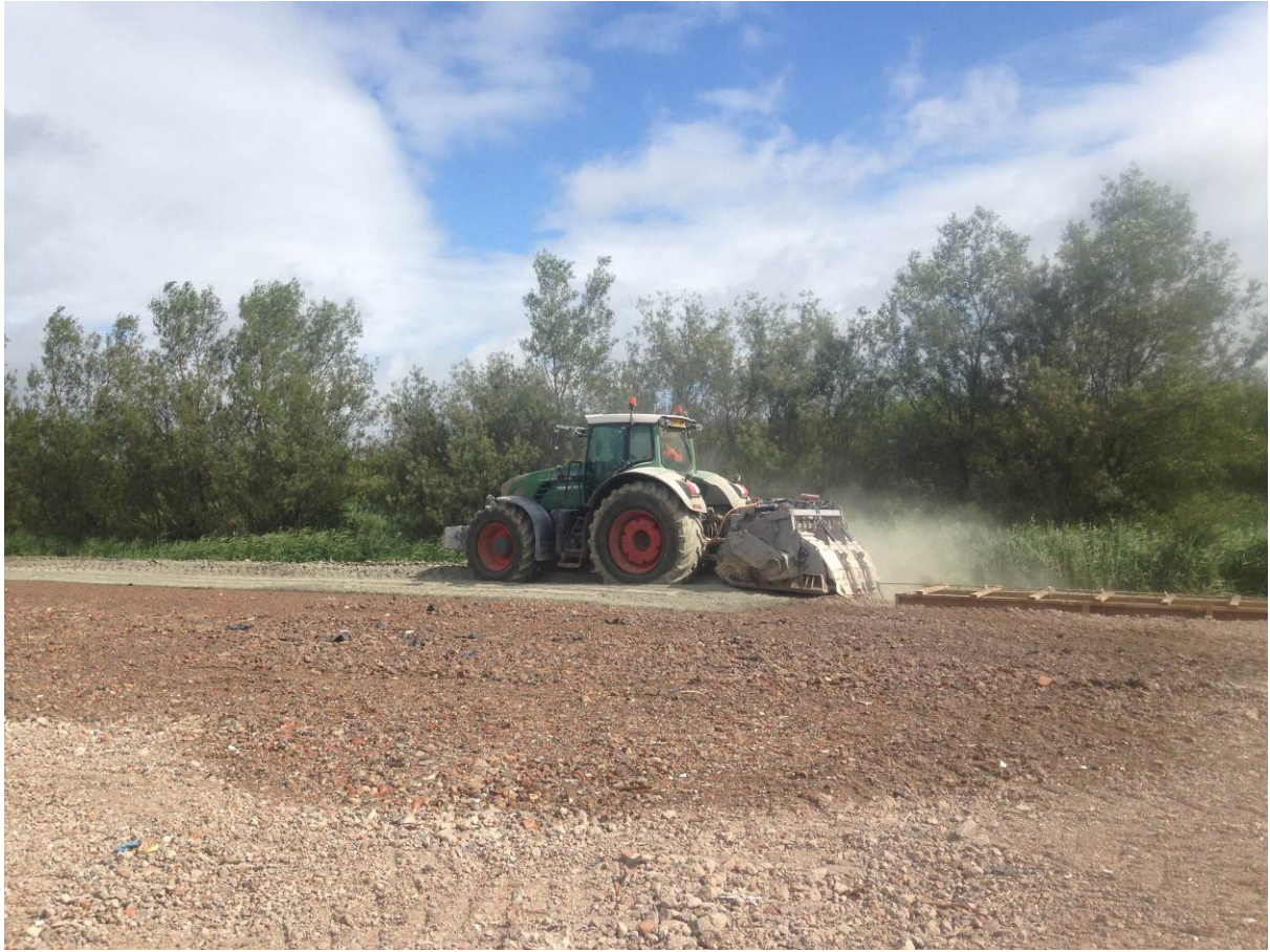
Crushing and mixing of aggregate with cement powder
