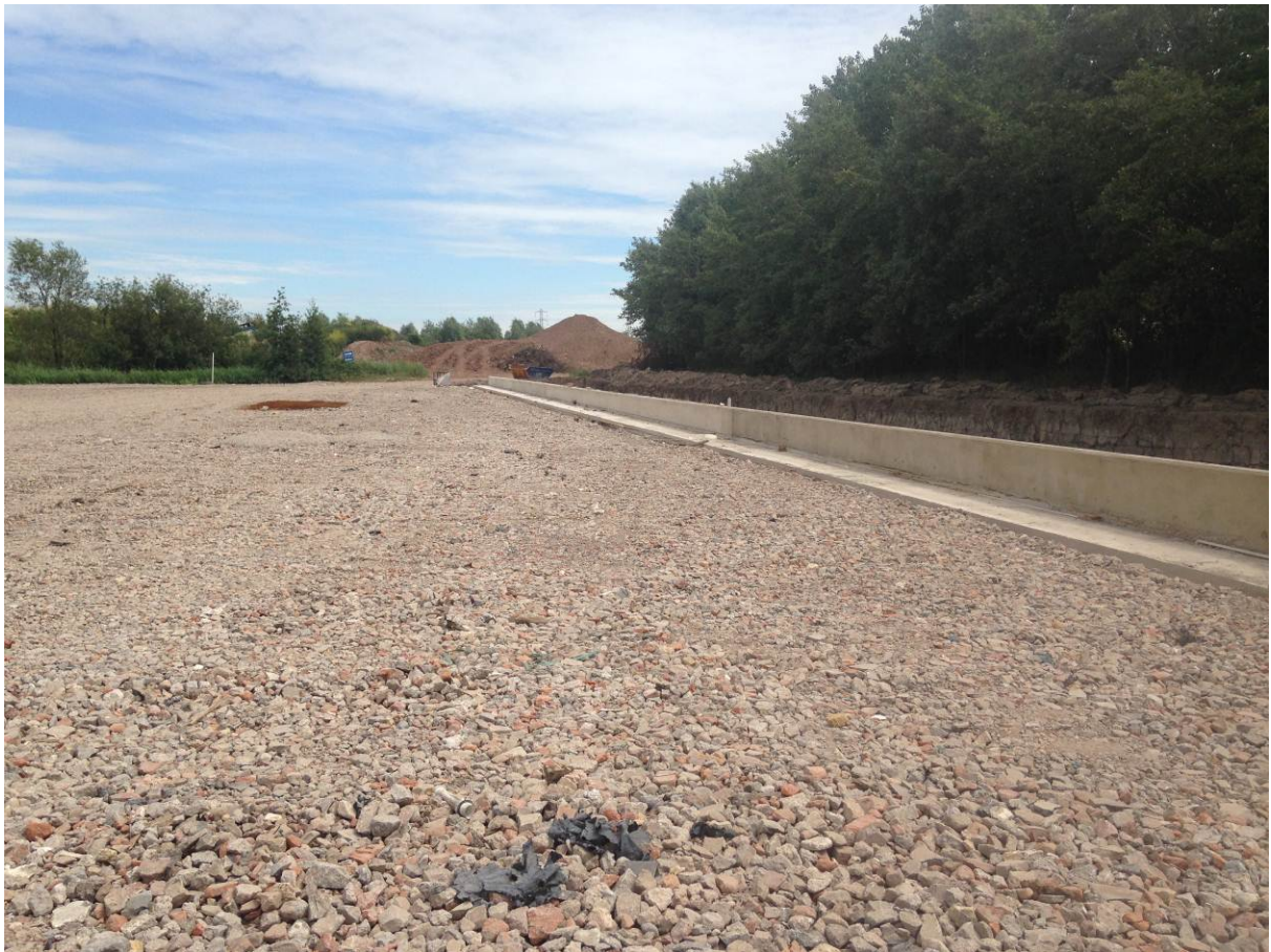
Concrete drainage channel and headwall
