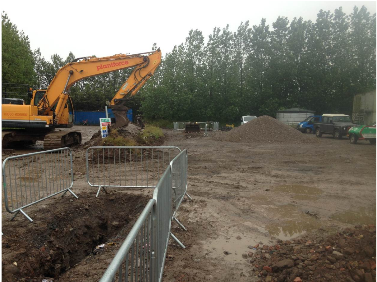
Excavation for drainage pipe
