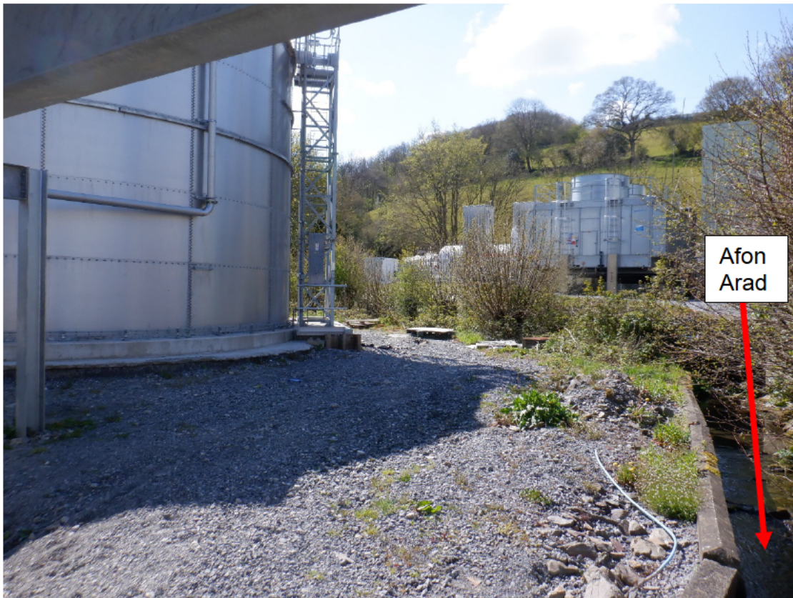
Photograph showing the proximity of the single skinned (unbundled) balance tank of the new ETP, to the Afon Arad watercourse.
