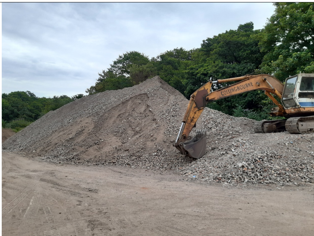
Photo 2 – processed material, estimated to be around 3000 tonnes.
