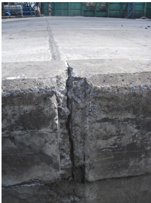
Photograph 1.11, Close Up Of External Face Of West Wall
