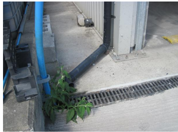
Photograph 2.3, View of “Aco” type drainage currently installed to prevent water ingress into the building.
