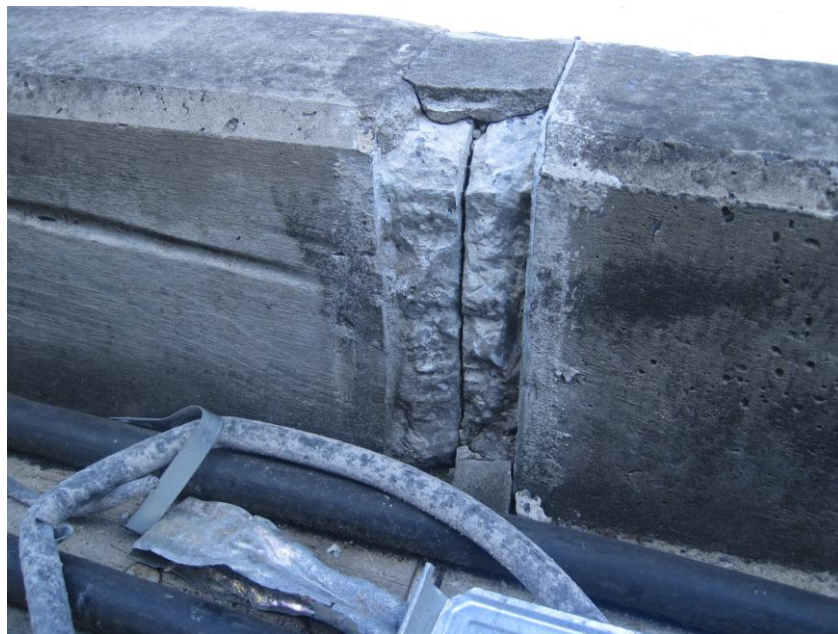
Photograph 1.8, Close Up Of Construction Joint
