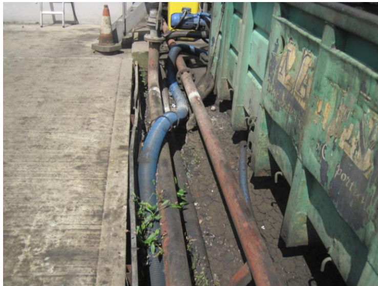
Photograph 1.10, View Of Intermediate Bund Wall Looking North
