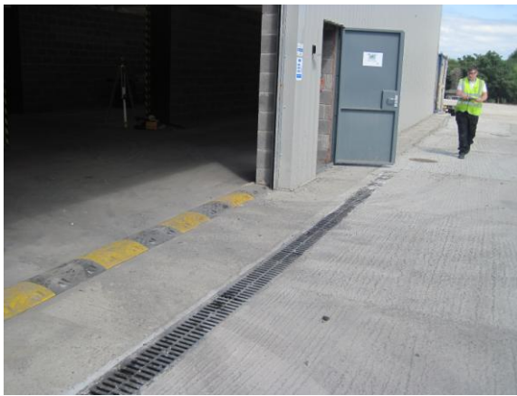
Photograph 2.3, View of “Aco” type drainage currently installed to prevent water ingress into the building.
