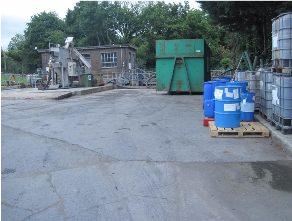
Photograph 4.1, View of Sewerage Off Loading Area Looking North
