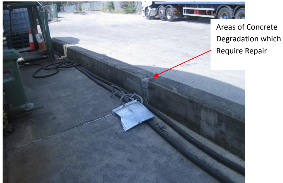
Photograph 1.7, Internal Face of North Bund Wall
