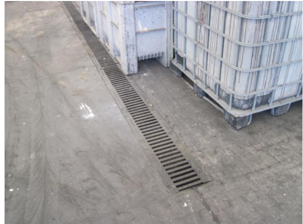
Photograph 2.2, Views Of The Steel Gully Covers And “Aco” Drains Present In The Transfer Building
