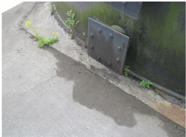
Photograph 1.6. View Of Joints At The North End Of The Oil Storage Bund
