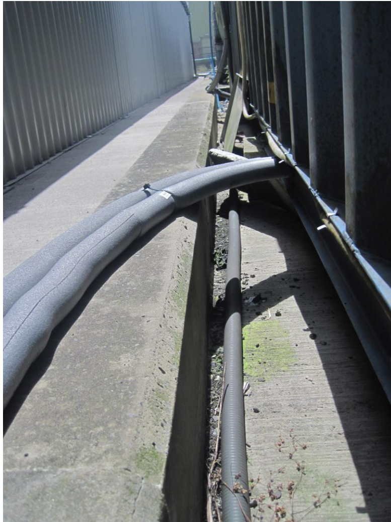
Photograph 1.9 View of East Bund Wall
