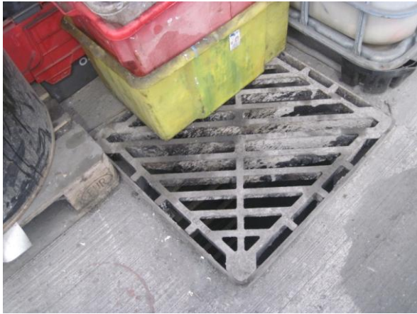
Photograph 2.2, Views Of The Steel Gully Covers And “Aco” Drains Present In The Transfer Building
