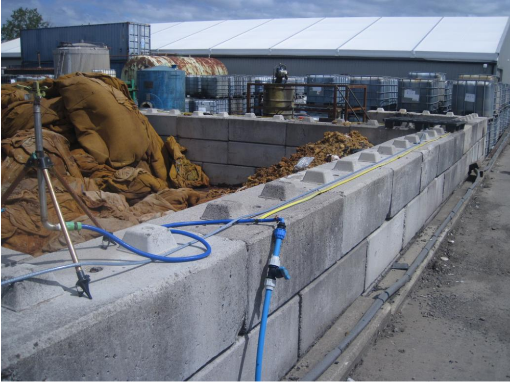
Photograph 1.12, View Of Concrete Block Wall At The South West Corner
