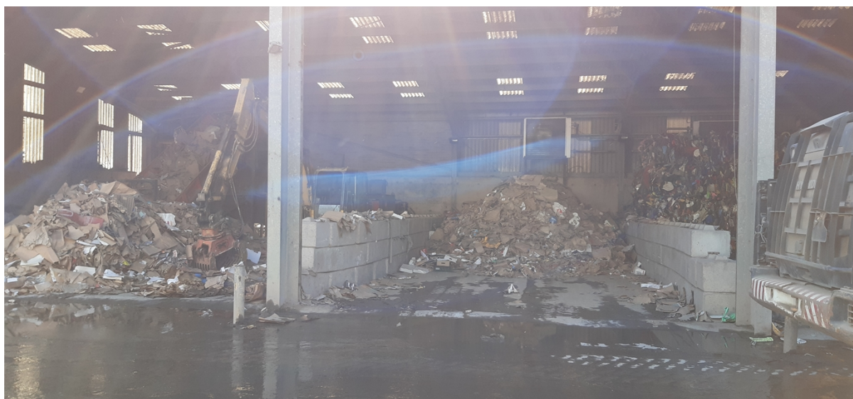
Photo 2 - View inside waste transfer station building
