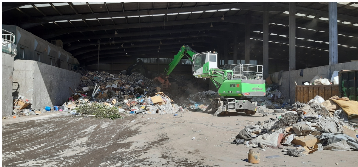
Photo 1 - View inside waste transfer station building
