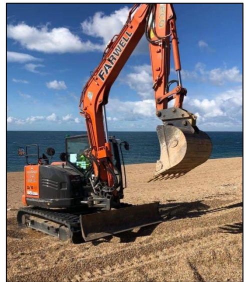
Figure 4: 9 tonne plant machine.
