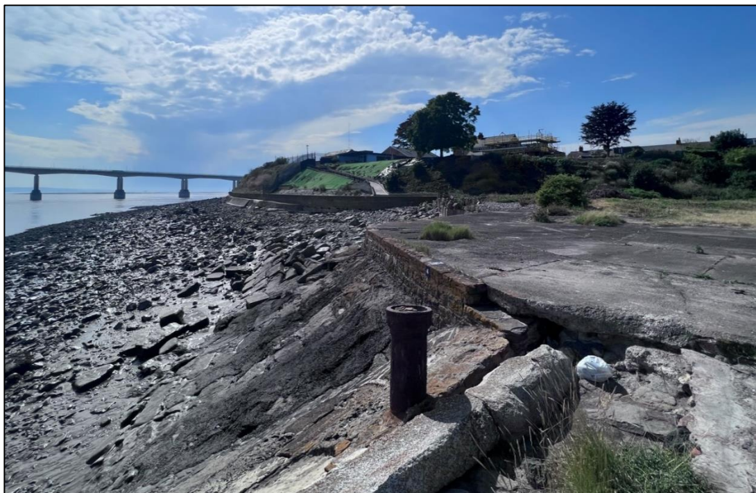
Figure 2: Sudbrook pier facing south at the defences downstream protecting the pumping station.
