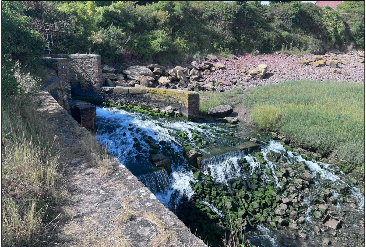
Figure 9: Headwall and wingwalls of Sudbrook tidal flap.
