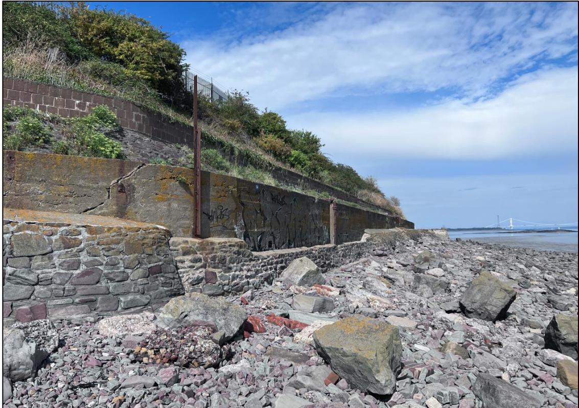
Figure 7: Tiered masonry and concrete cast wall defence, with masonry embankment above.
