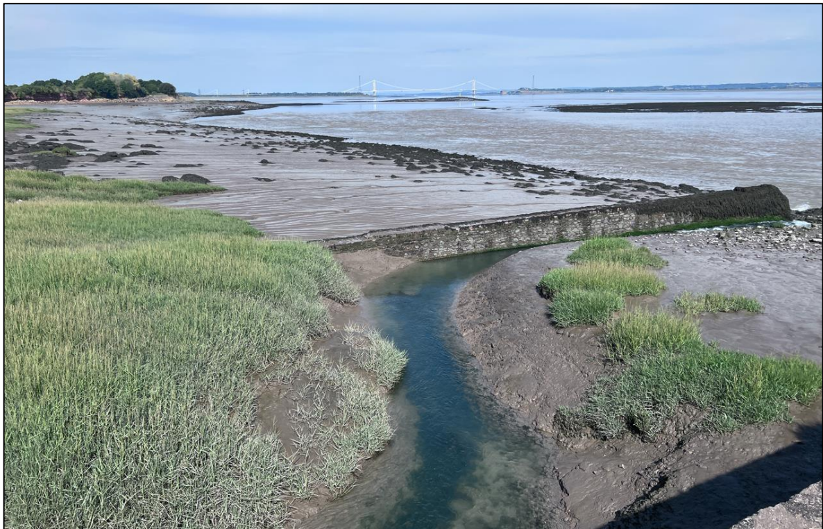
Figure 10: Dwarf wall directing the flow of water from the tidal flap.
