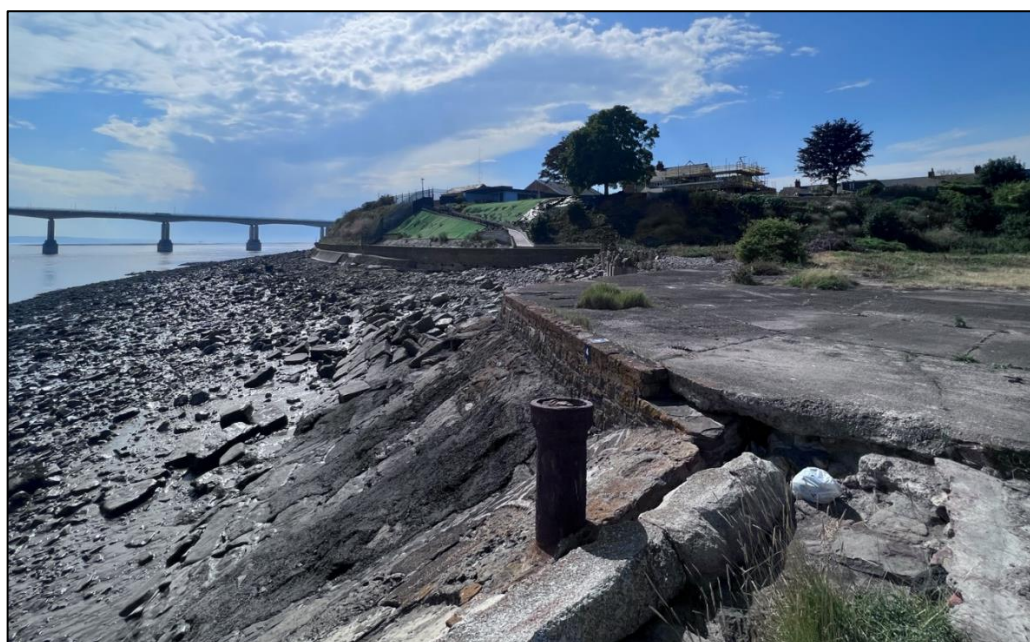
Figure 1: Sudbrook pier facing south at the defences downstream protecting the pumping station.
