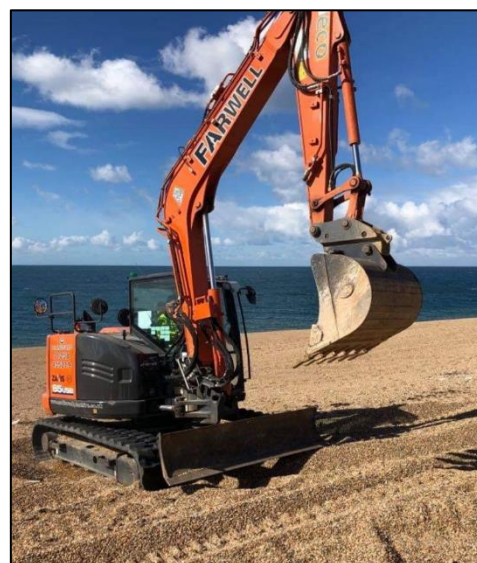
Figure 4: 9 tonne plant machine.
