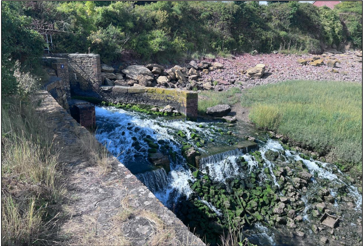
Figure 9: Headwall and wingwalls of Sudbrook tidal flap.
