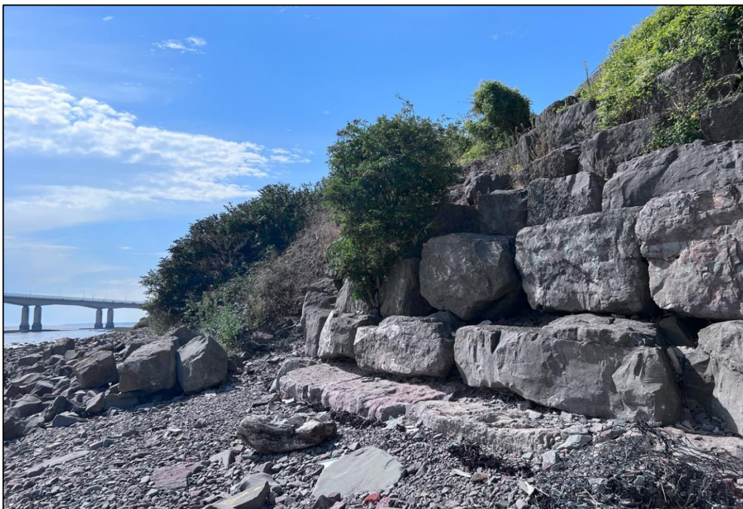
Figure 6: Rock armour along the southern portion of the defence line, below a small public park.
