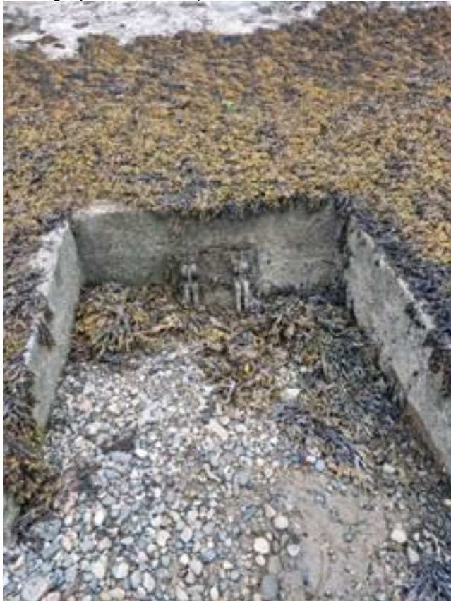
Photograph 4 – tidal flap valve
