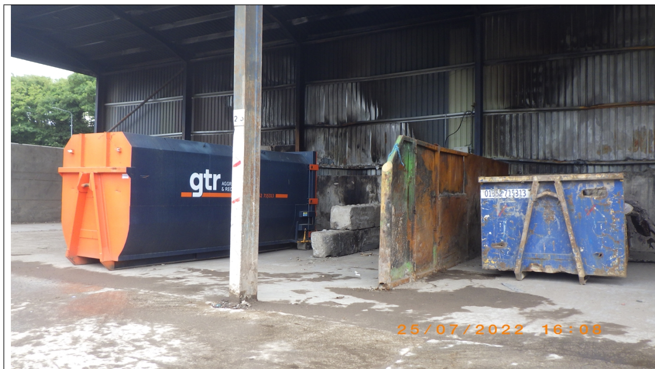
Photographs showing the transfer building
