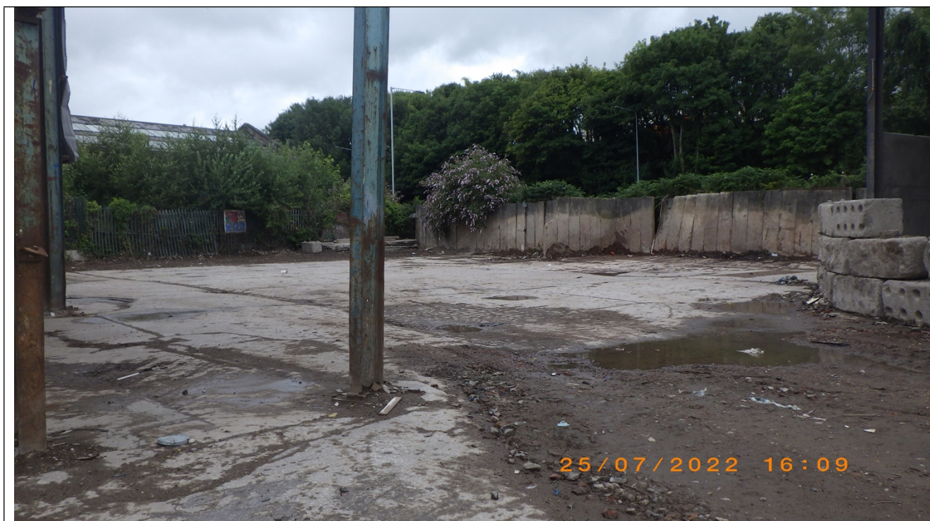
Photographs showing the Recycling Building and yard adjacent to the transfer building.
