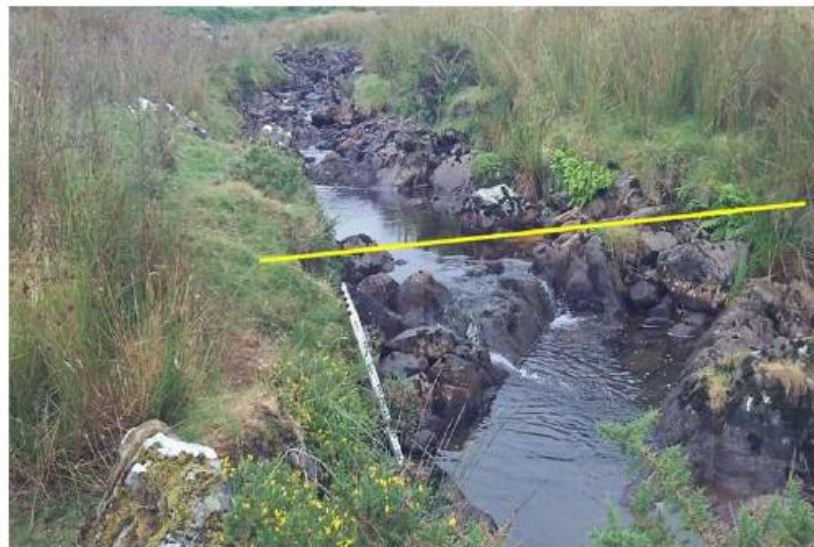
Weir location SH80247 20191
