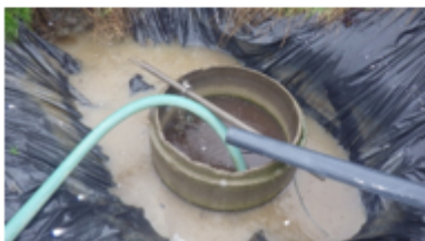
Photograph 6 – Sump below leachate treatment lagoon.
