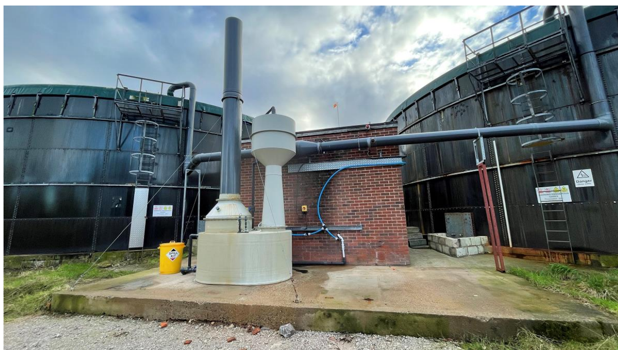
Photo 1: The Existing Effluent Balance and Diversions Tanks and the Odour Scrubber and Stack
