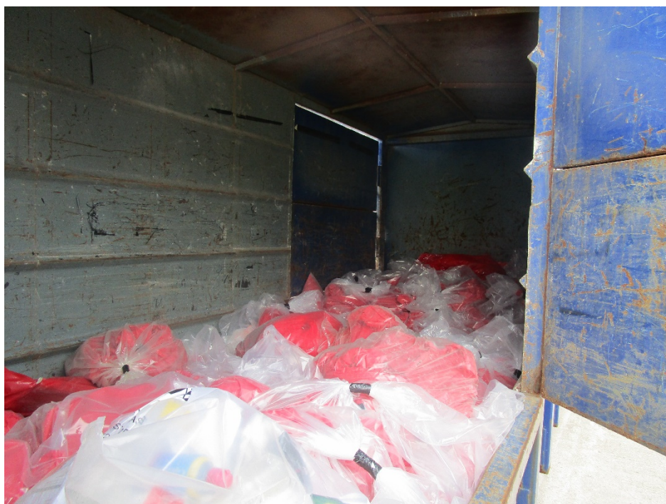
Figure 2. Double bagged asbestos waste inside the secure skip
