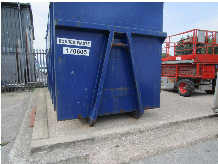
Figure 1. Locked and labelled asbestos waste skip stored on an impermeable surface
