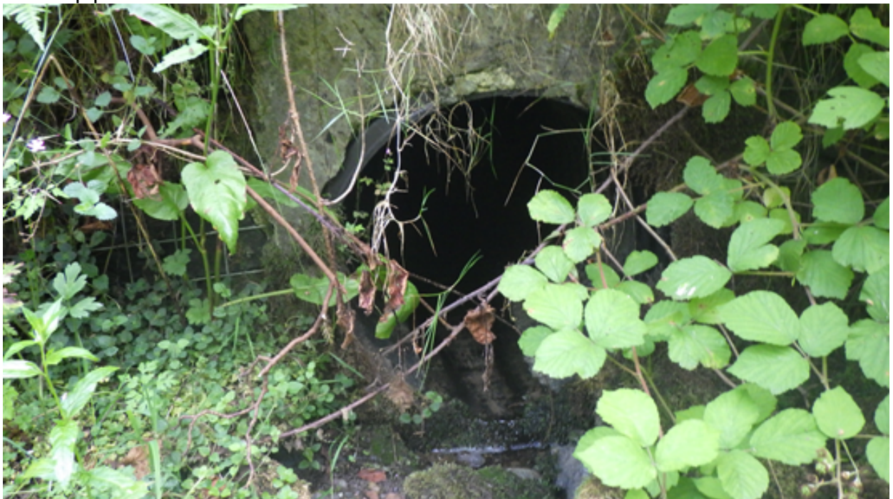
Outfall pipe - no bars fitted
