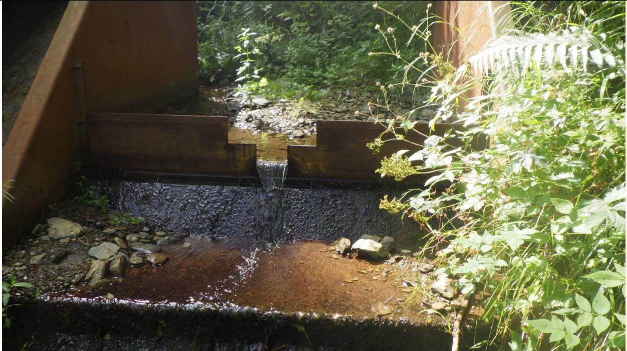
Outfall pipe - no bars fitted
