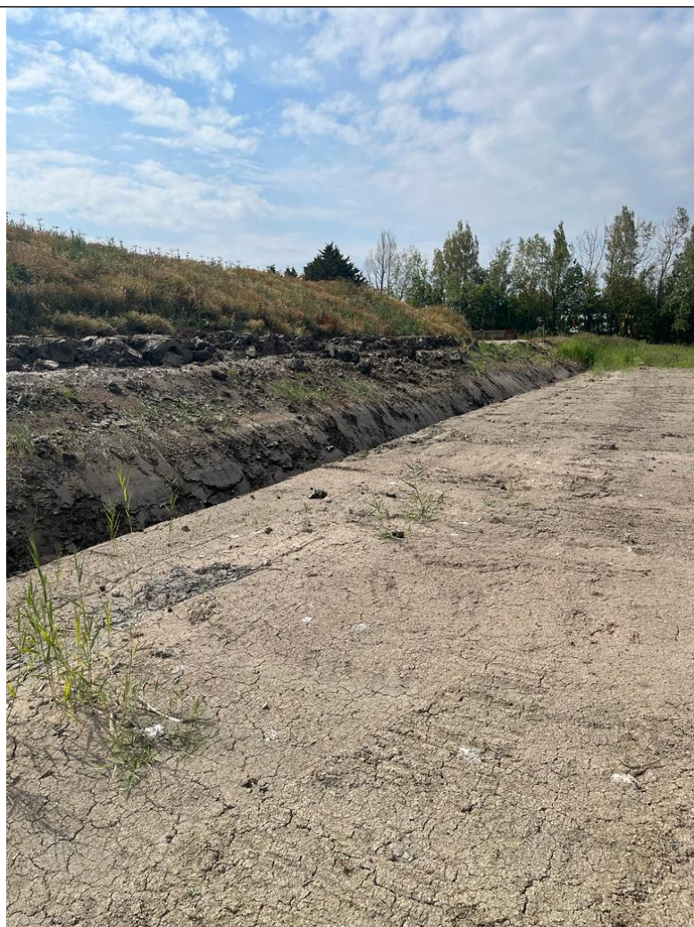
Picture 7 - Image showing the interceptor ditch with the large soil stockpile in the background in the same location with vegetation growing.
