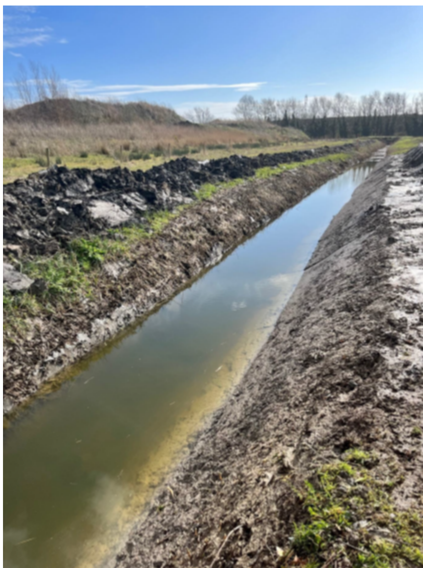
Picture 4 (above) and Picture 5 (below) - Images of the completed remediation works on the SSSI Reen.
