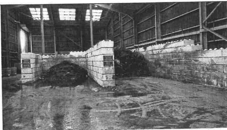
(L to R) Sweepings and Greens Stored in Western section of IVC building
