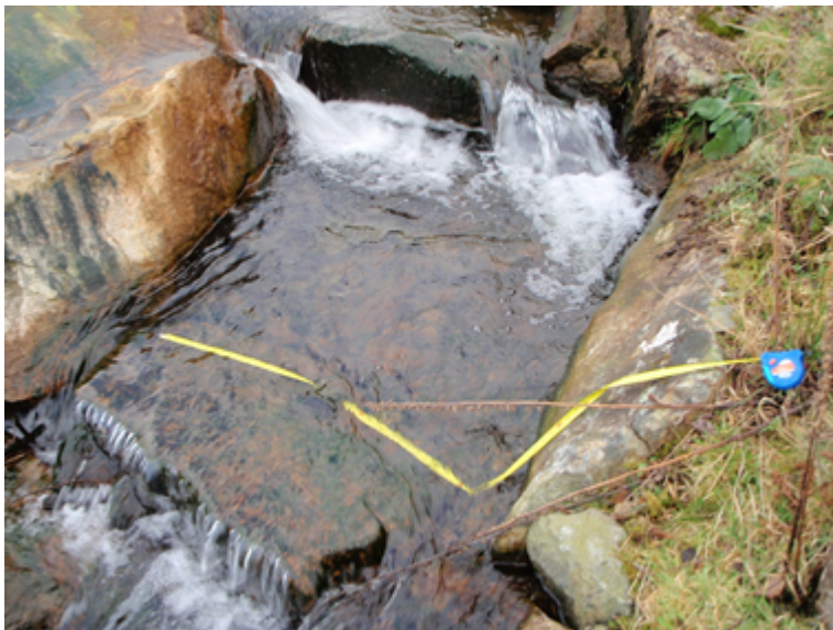
Picture 4 - The width of the fish pass. Measured approximately.
