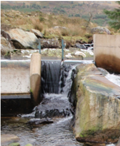
Picture 6 - Concrete slab which is higher than the river bed in-between the screen intake and the rocky ramp fish pass.
