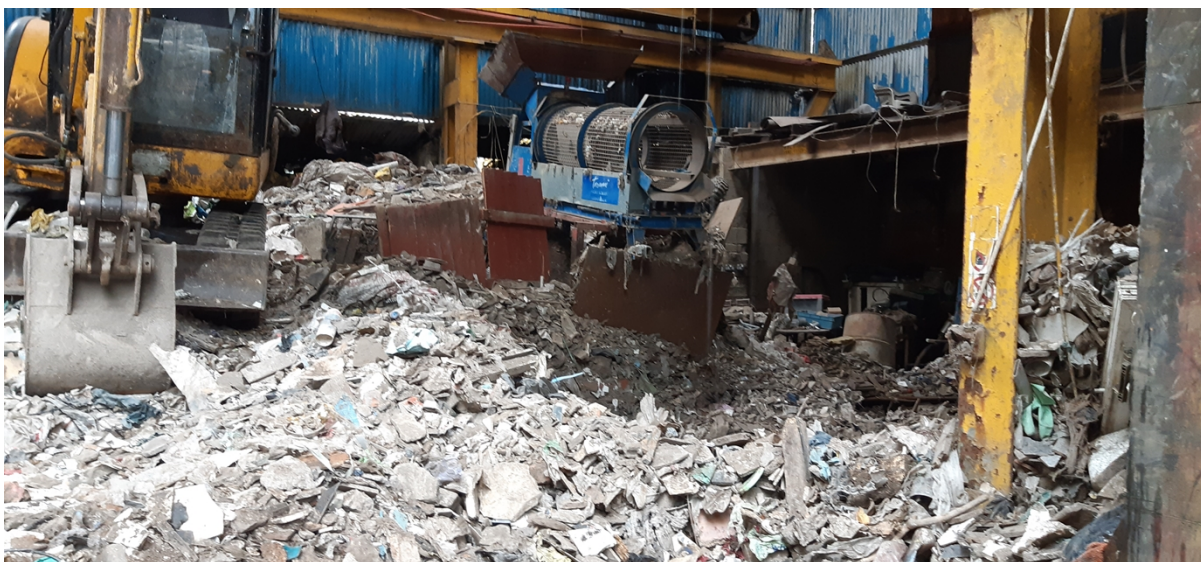
Photo 1 - Waste stored within permitted area of ADJ Skip Hire
