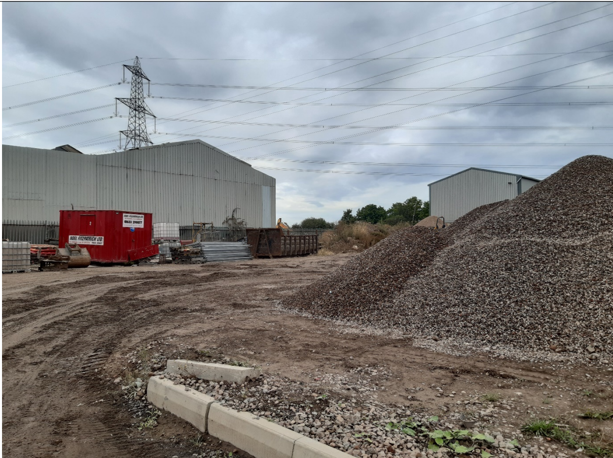
Photo 2 – area showing where incoming vehicles enter and turn right into processing area
