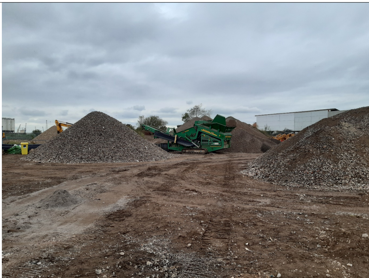
Photo 1 – area showing material processing with screening equipment
