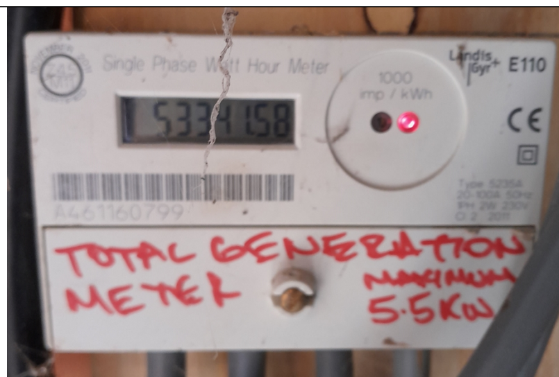
ED4 - Photo of meter: serial number A461160799 Reading: 53341.58
