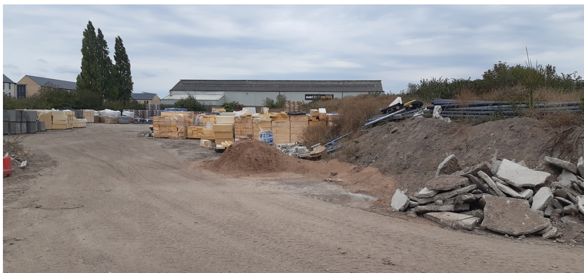
Photo 1 - Overview of site containing building materials
