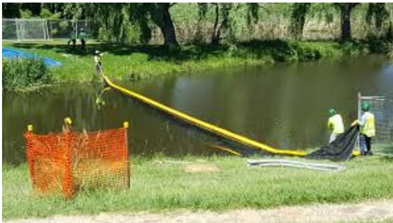
Figure 13: Silt curtains being used- for illustration purpose only
