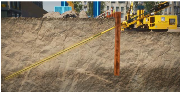
Fig 10. : Grouting the driven bolts
