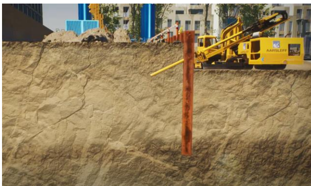
Fig.8 : First bolt section being driven
