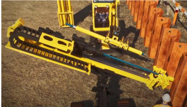
Fig.6 : Indicative drilling and loading of bolt sections
