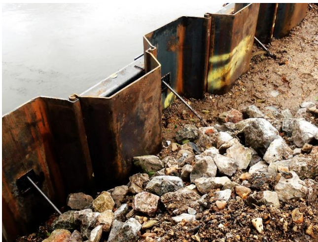
Fig. : 12 – Backfilling and reinstatement
