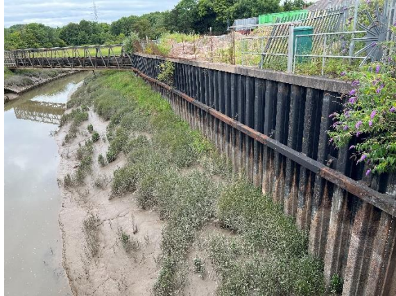
Original Newport Rd. / River Rhymney works within watercourse
