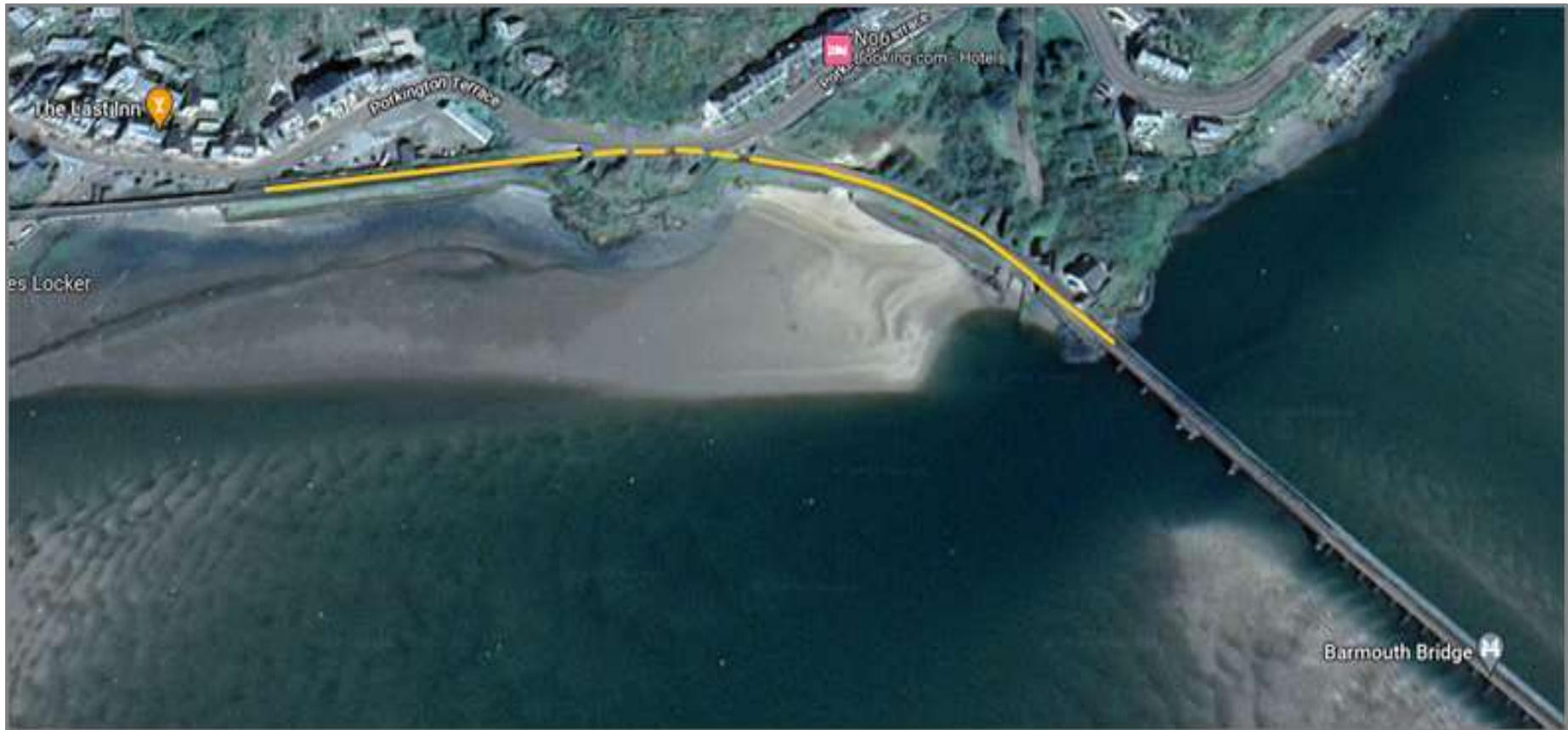
Barmouth Viaduct worksite
