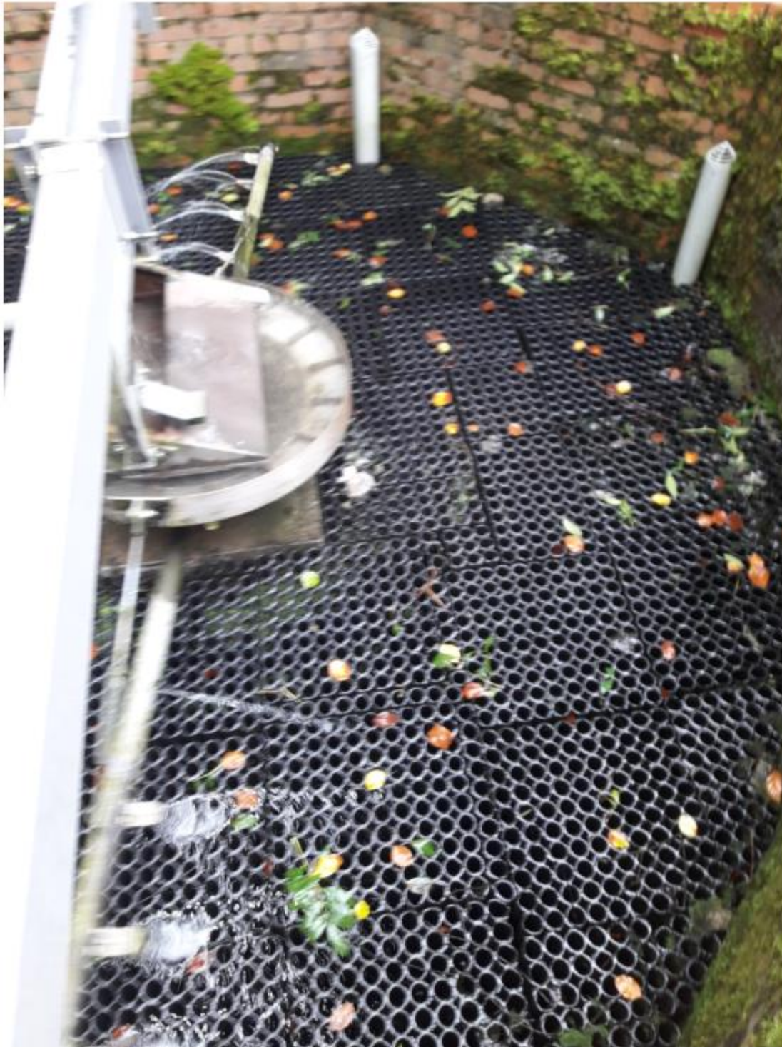
Sanitary waste on filter media.
