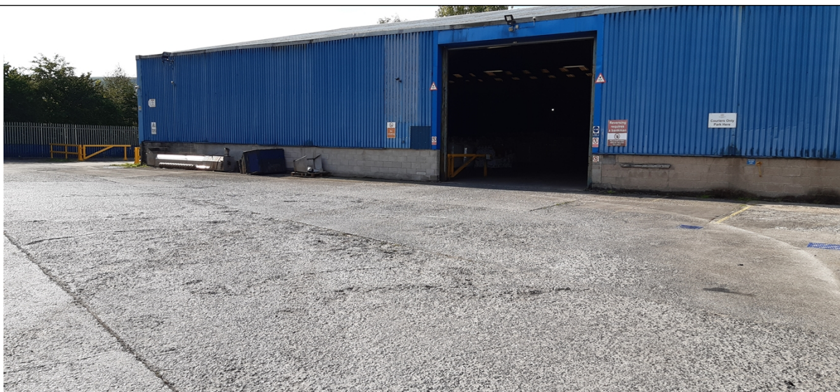
Photo 3 - Litter netting located along perimeter of security fencing (background left)
