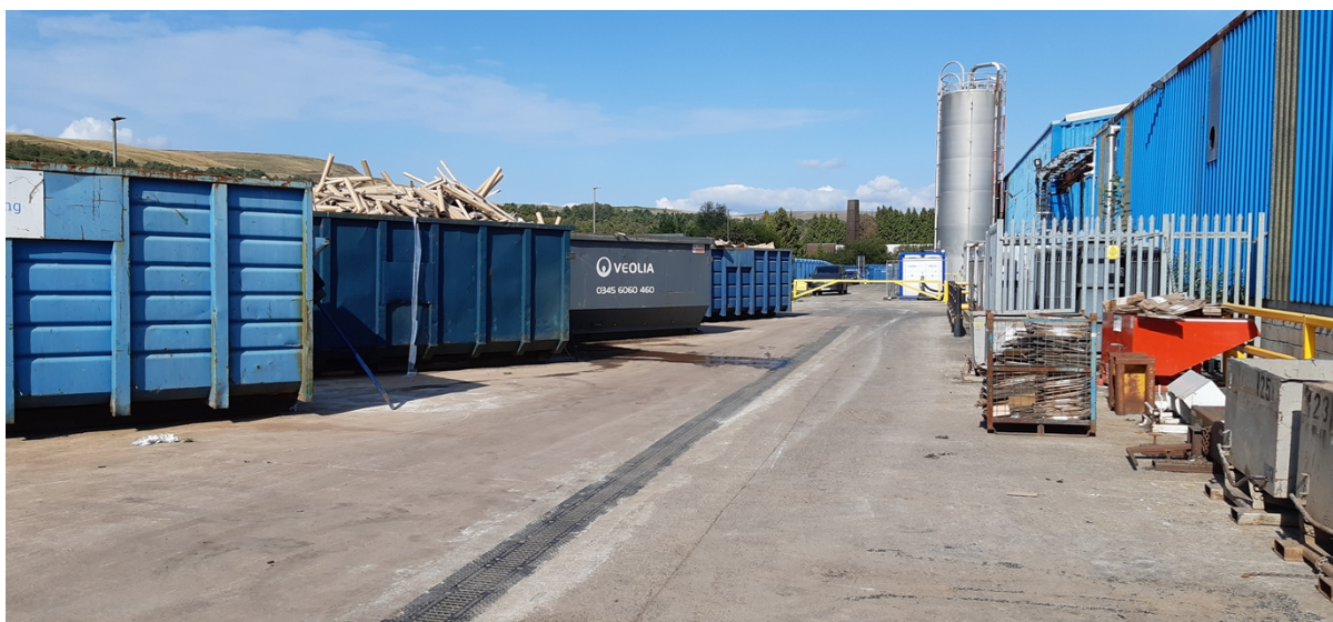
Photo 4 - Infrastructure improvements on site and storage of large waste skips
