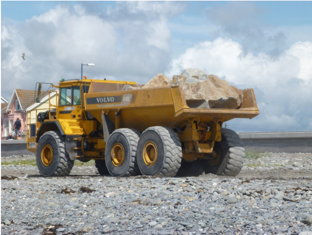
Figure 1-5 - Wheeled Dumper Transporting Rock
