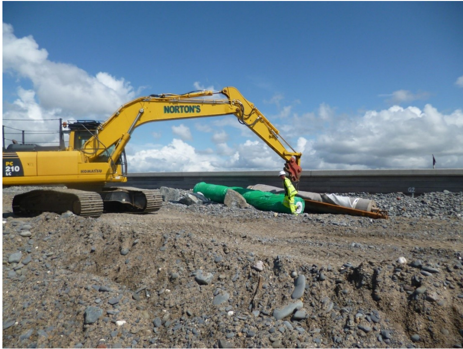
Figure 1-4 - Tracked Excavator with Grab to Pick Up and Place Rock
