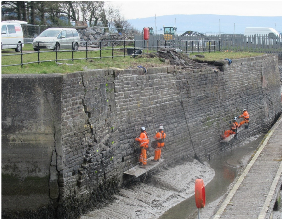
Figure 1-11 - Repointing and Wall Repairs by Rope Access
