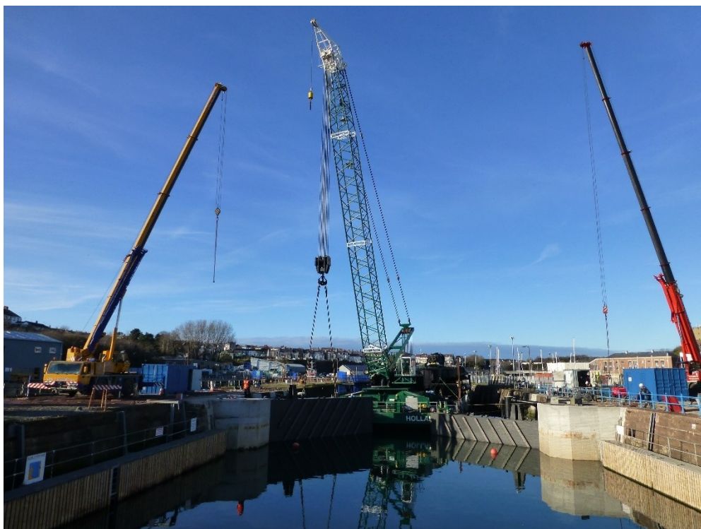
Figure 1-13 Barge, Crane and Gate at Milford Marina
