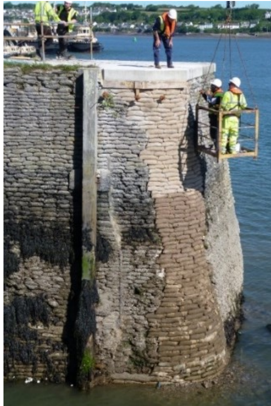
Figure 1-11 - Repointing and Wall Repairs by Rope Access
