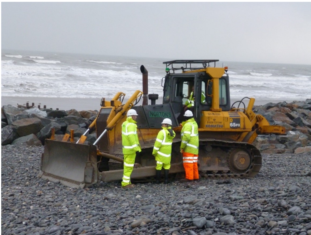
Figure 1-6 - Dozer to Spread out the Imported Shingle
