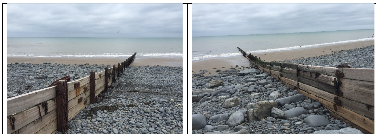
Figure 2-11 - Existing timber groynes on South Beach
