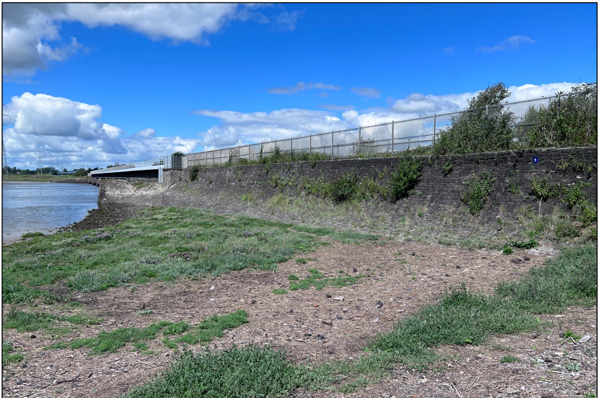
Figure 6: Section of wall on the eastern shore of the project.
