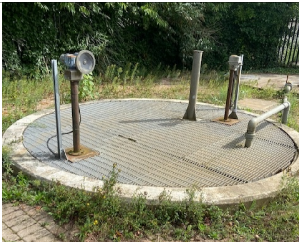
Photo 1: Pumping station C – leachate collection tank
