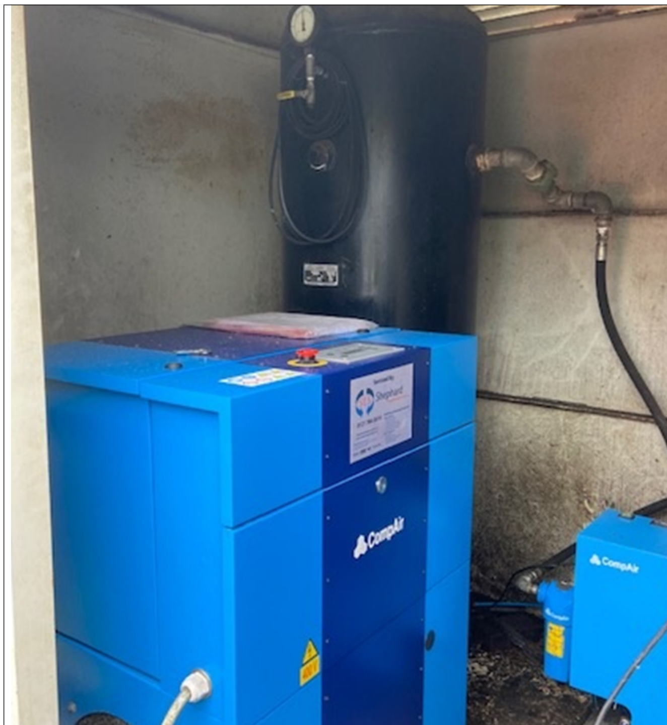
Photo 2: Compressor pump for pumping station D – located at the landfill flare compound
