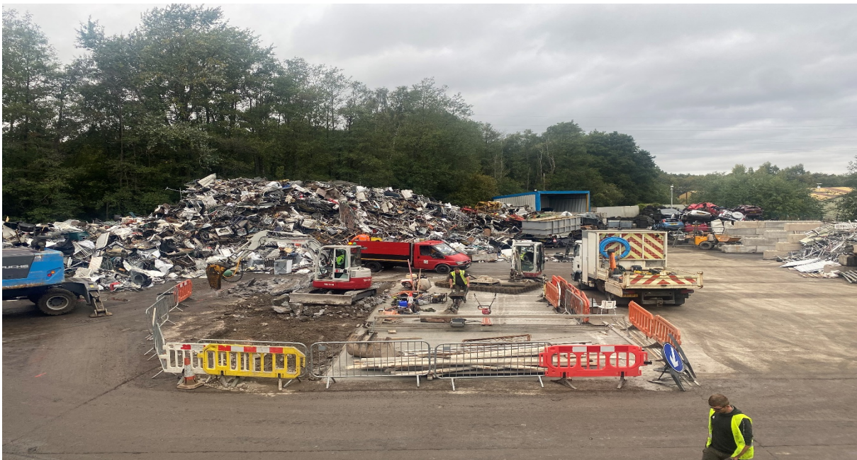
Image 1 - Picture showing the yard being resurfaced with the primary metal stockpile moved along the site boundary
