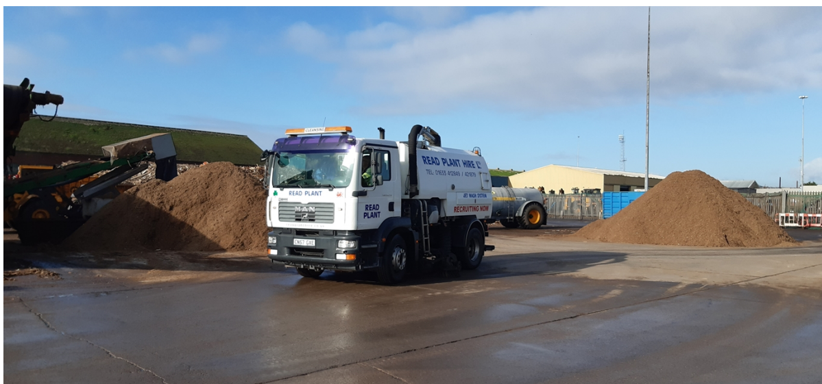
Photo 2 - On site road sweeper in constant use to minimise road deposits
